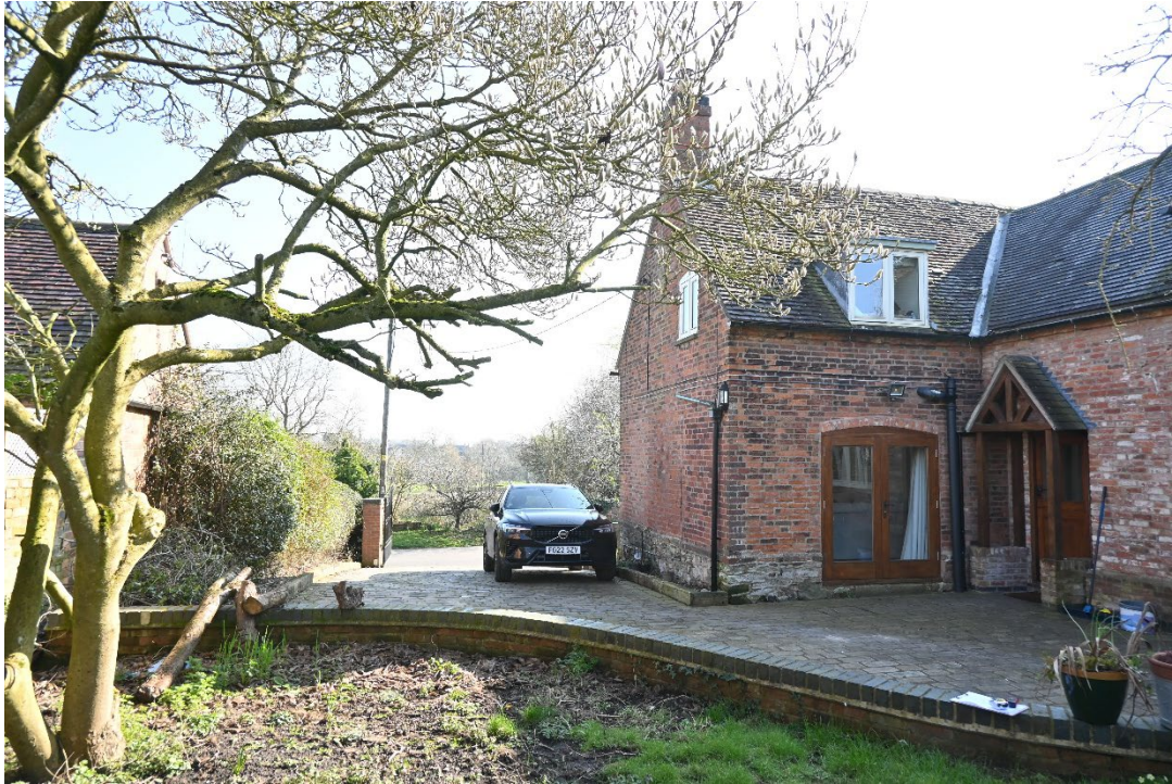
Fig. 6 Cottage Side and Rear Elevation with view down the driveway
