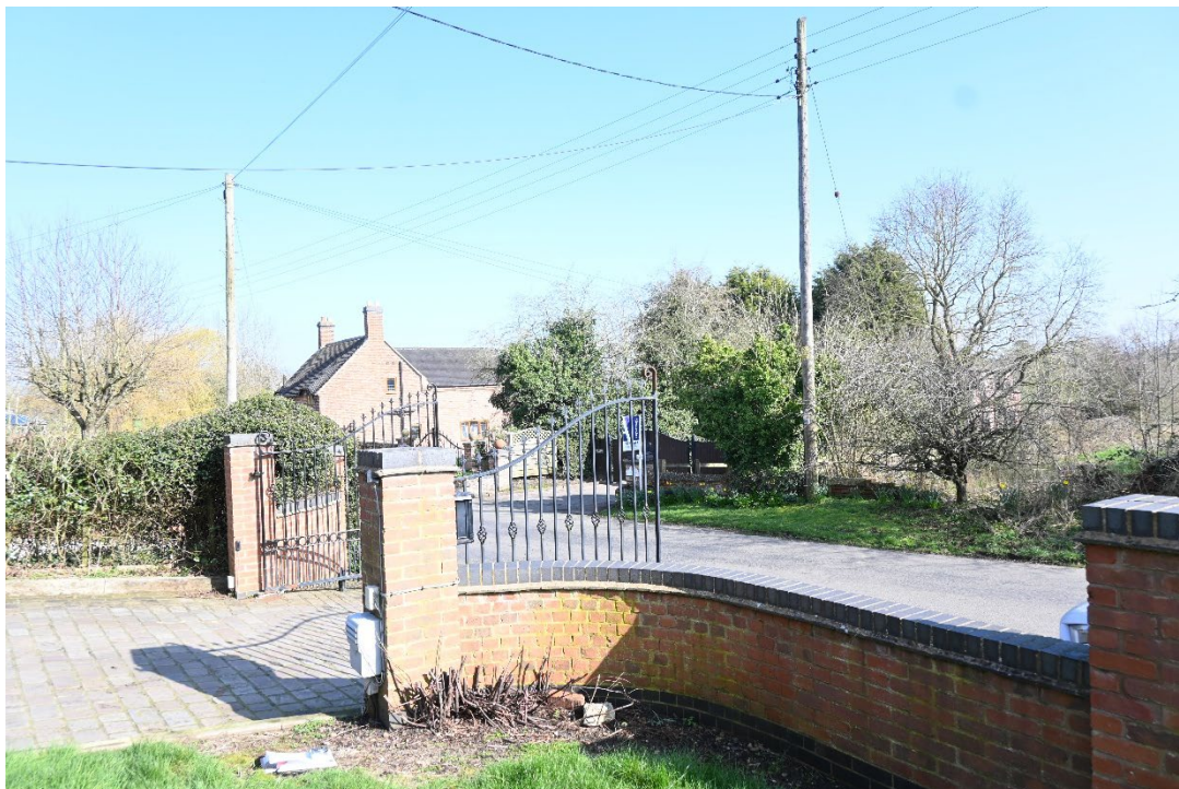
Fig. 7 Cottage front boundary wall and gated access
