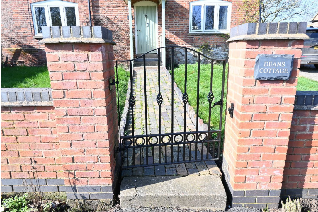
Fig. 8 Cottage front boundary wall and gated access
