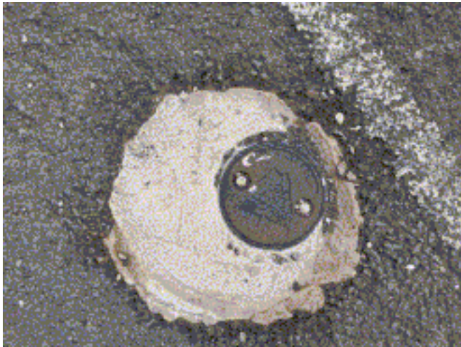
Photo 3: Monitoring well cover identified in the car park.
