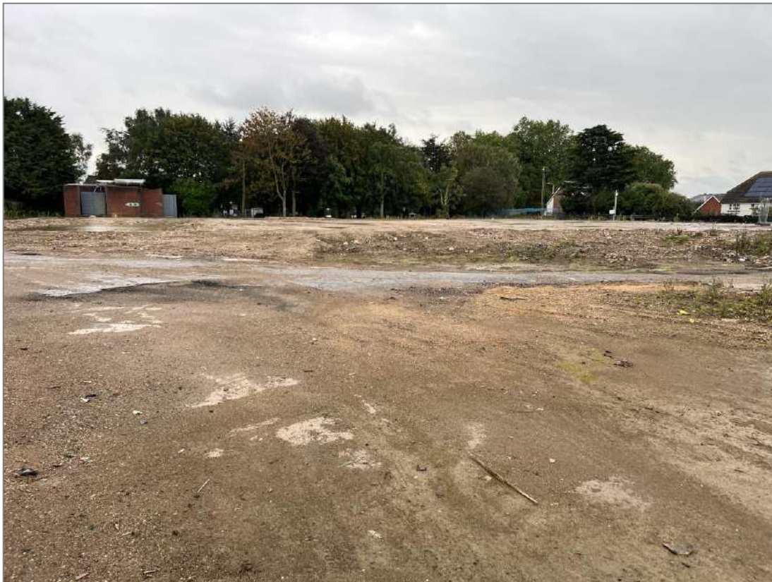
Photo 14. Example of hardstanding following building demolitions
