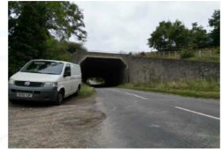
View 3. Facing left at access onto Markfield Road.
