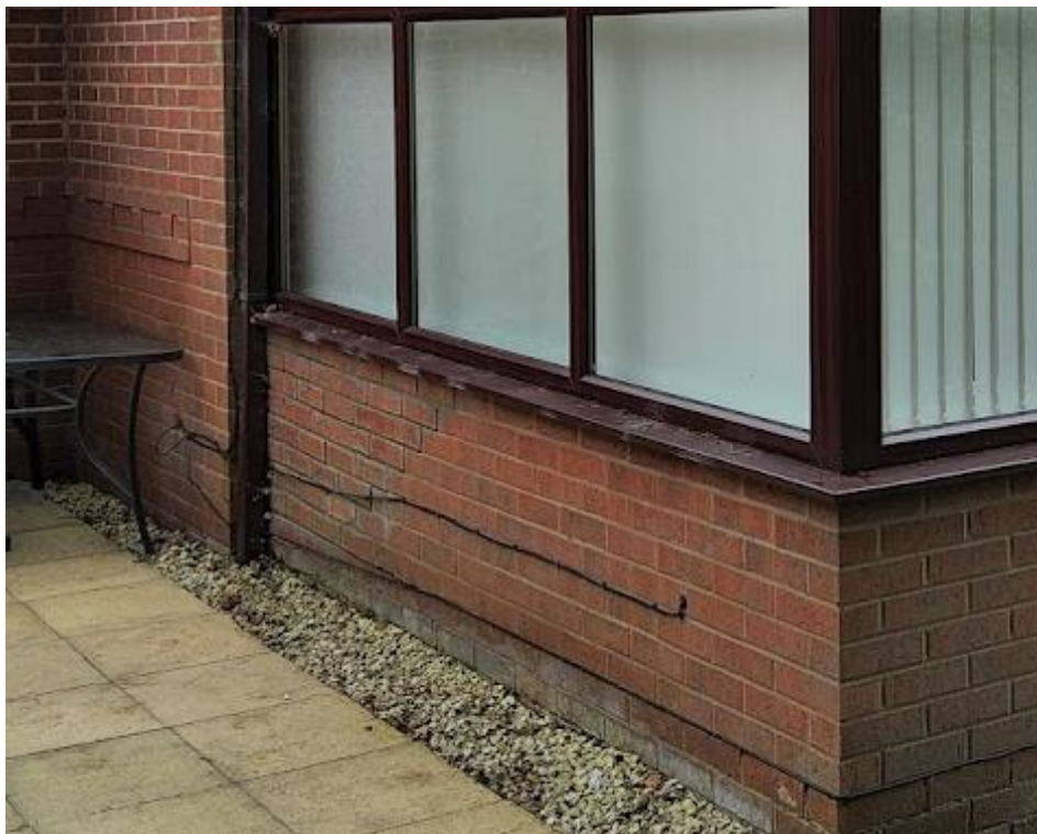
Photo 3 – Recently repaired brickwork due to subsidence movement
