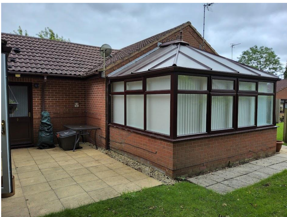
Photo 2 – Rear elevation of the property
