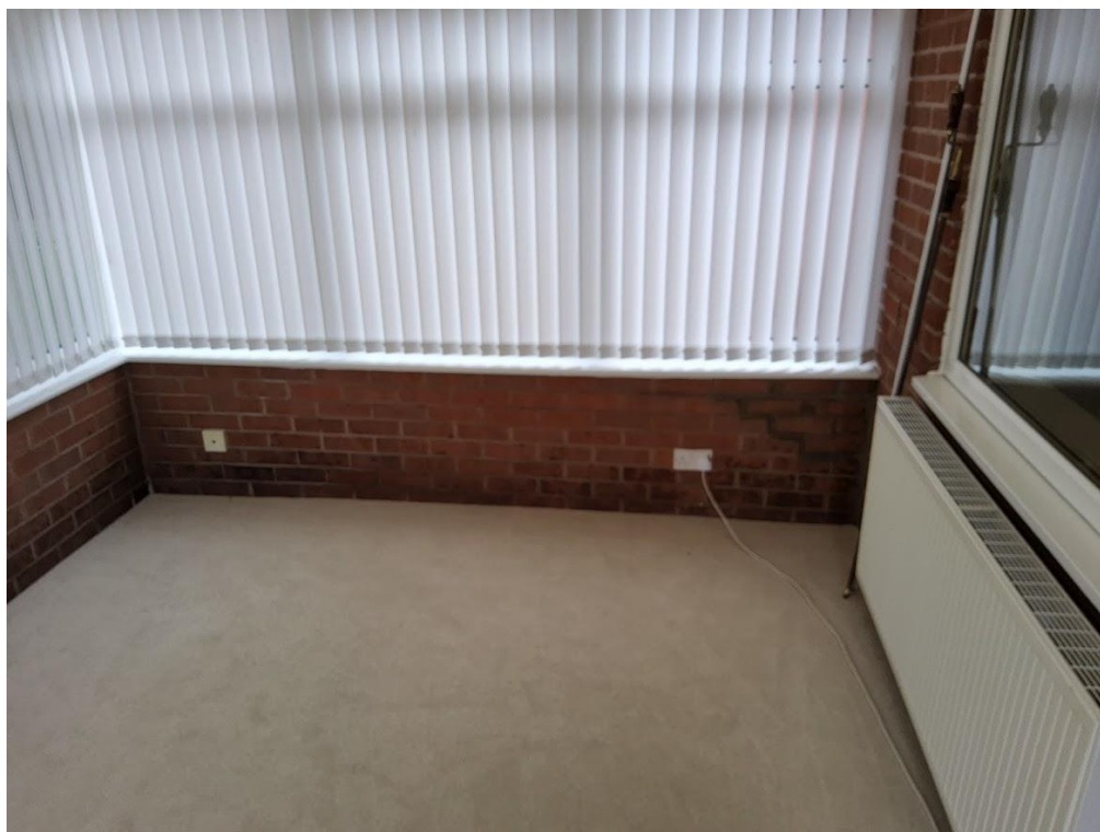
Photo 4 – Recently repaired brickwork due to subsidence movement
