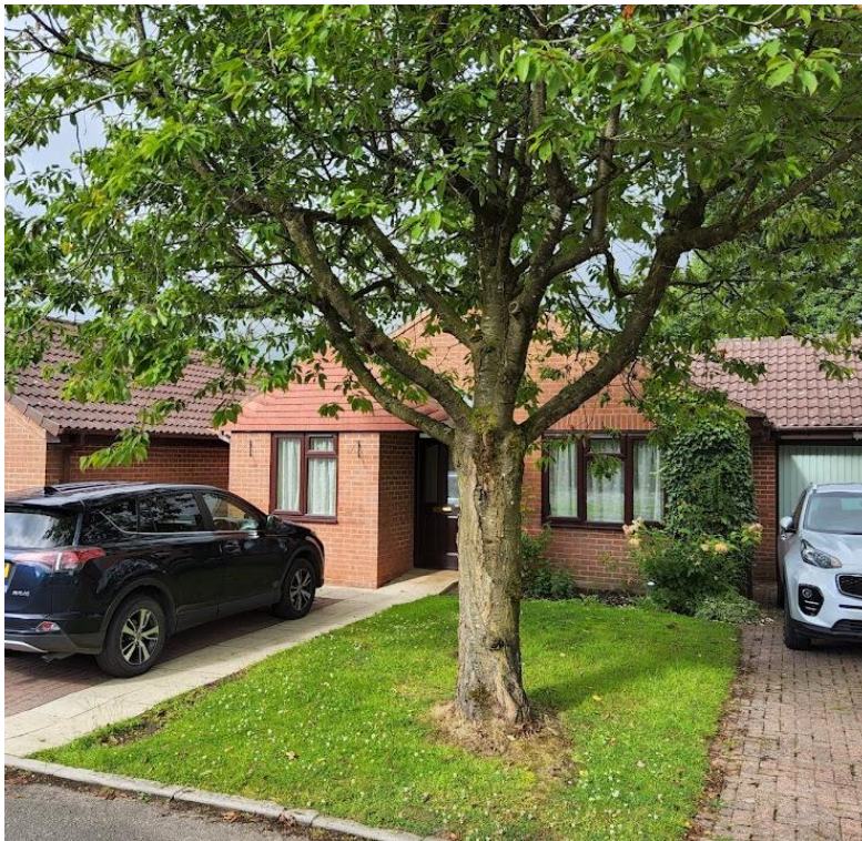
Photo 1 – Front elevation of the property
