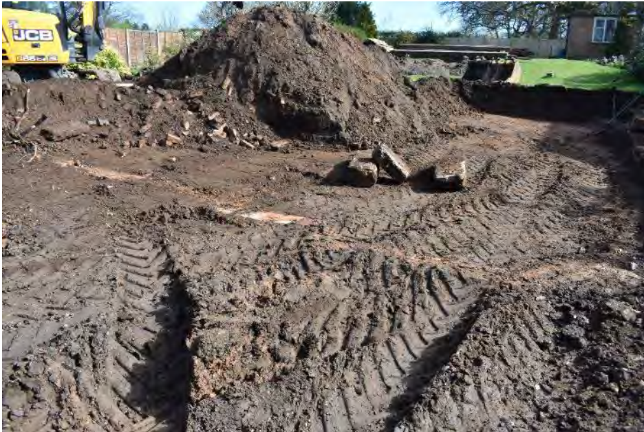
2 Working shot of ground reduction looking north-east
