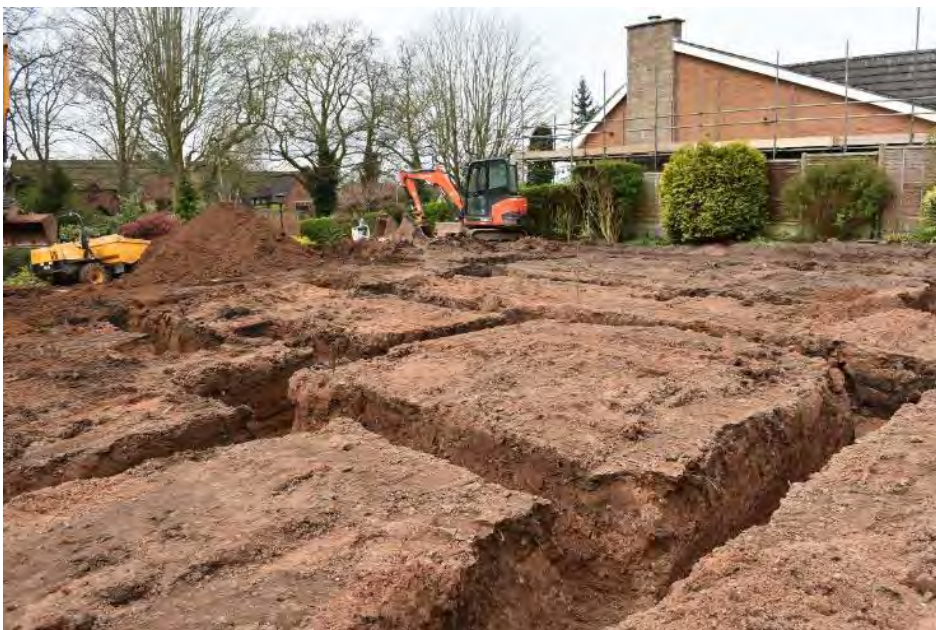
3 Excavated foundation trenches looking north-west
