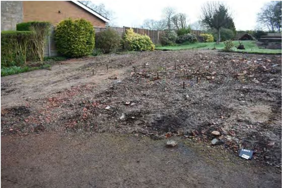
1 The Site following the removal of the demolished building, looking north-east
