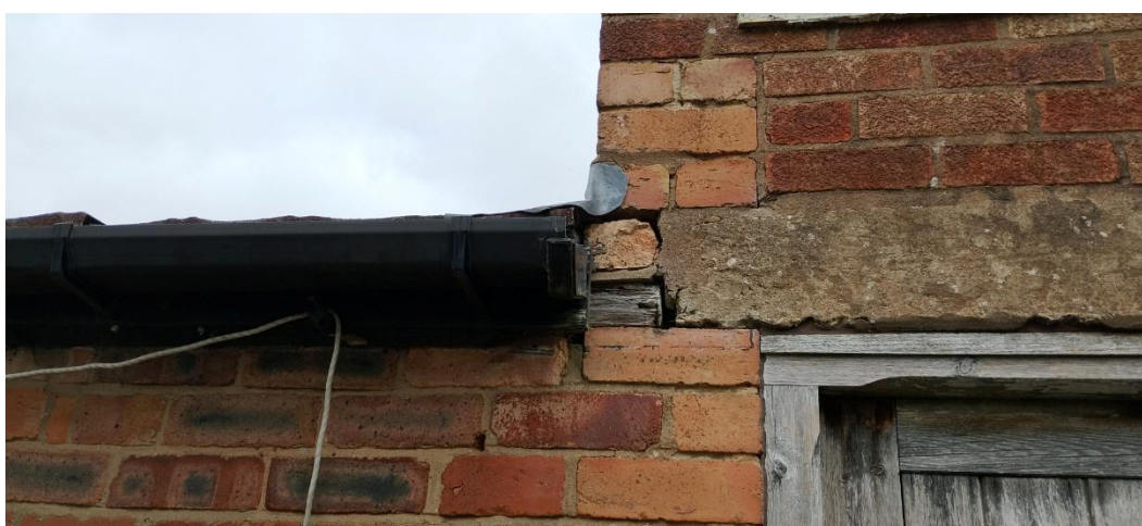
Photograph 8: Close-up of brickwork.
