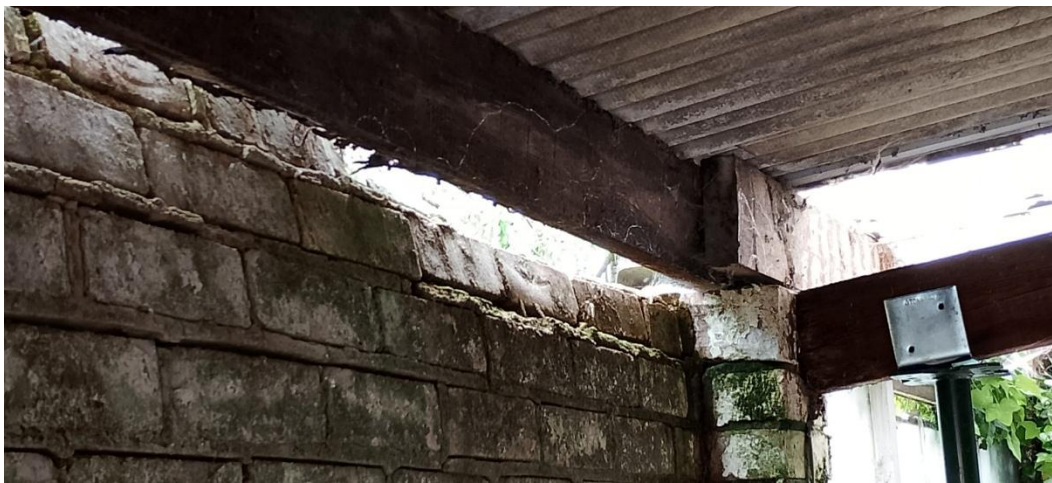
Photograph 6: Wall and roof junction.
