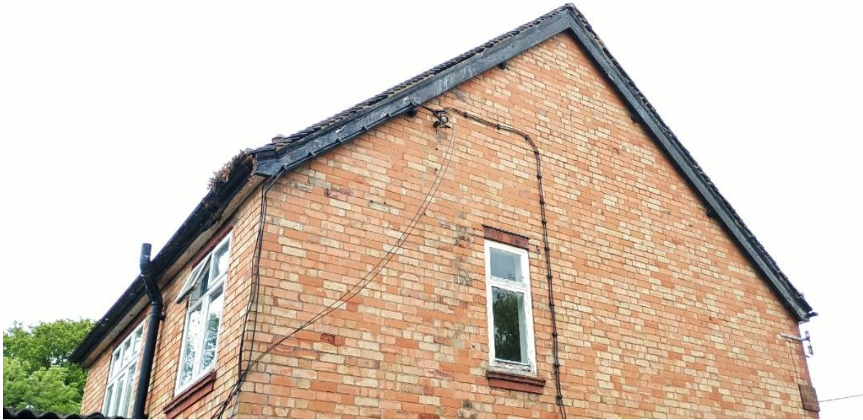
Photograph 15: Main dwelling gable elevation.
