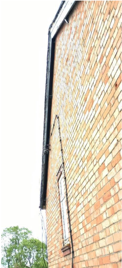
Photograph 9: View of fascias on external elevation.
