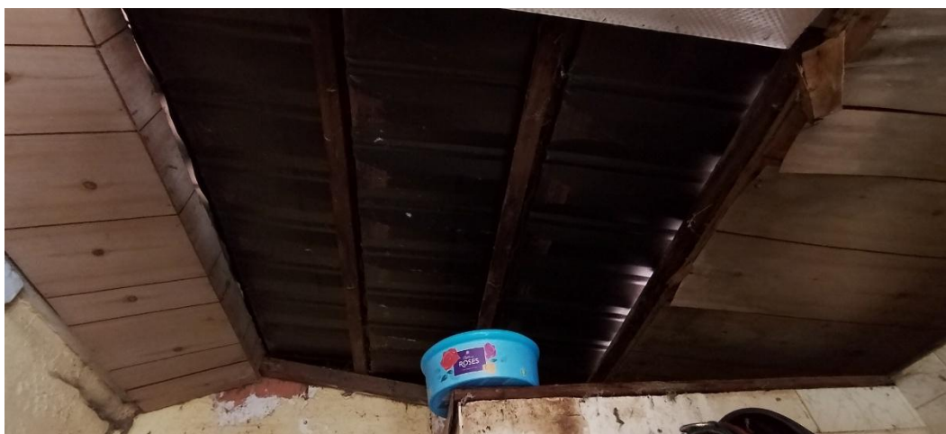
Photograph 7: Internal roof structure.
