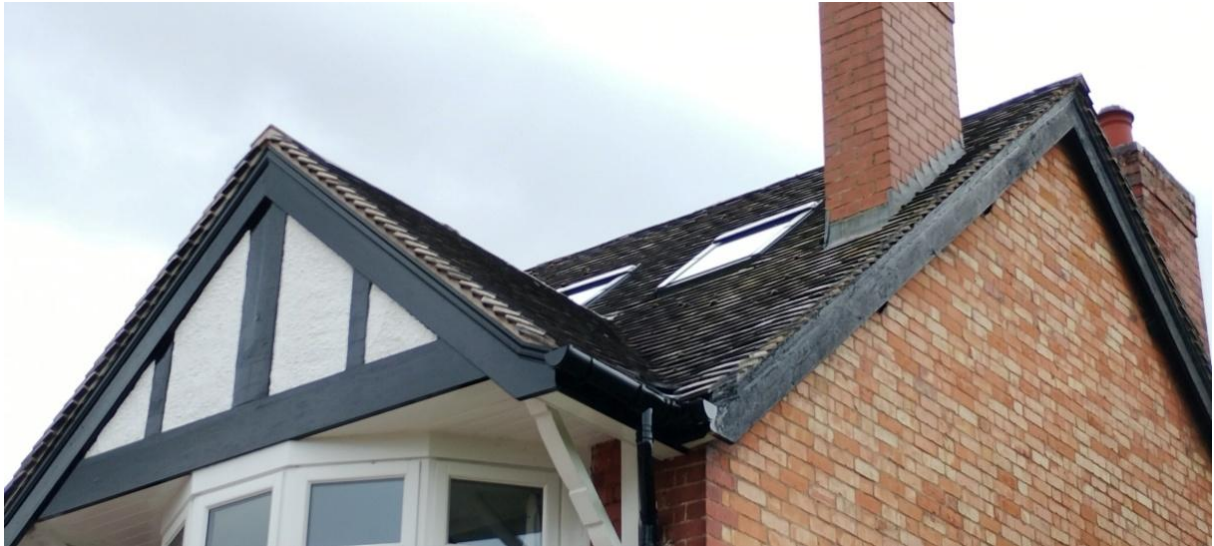
Photograph 13: Main dwelling roof slope with tiles, skylights and eaves.
