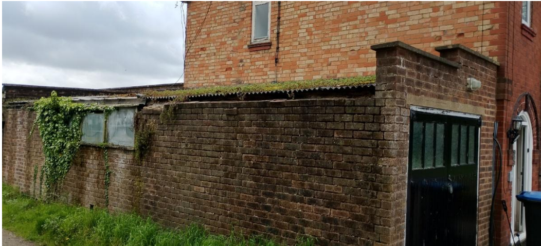
Photograph 3: View of garage section.
