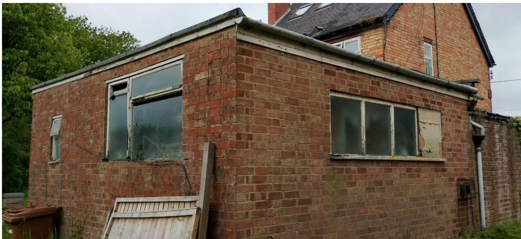
Photograph 4: External view of single-storey outbuilding.
