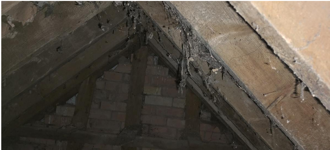
Photograph 2: Internal view of roof void.
