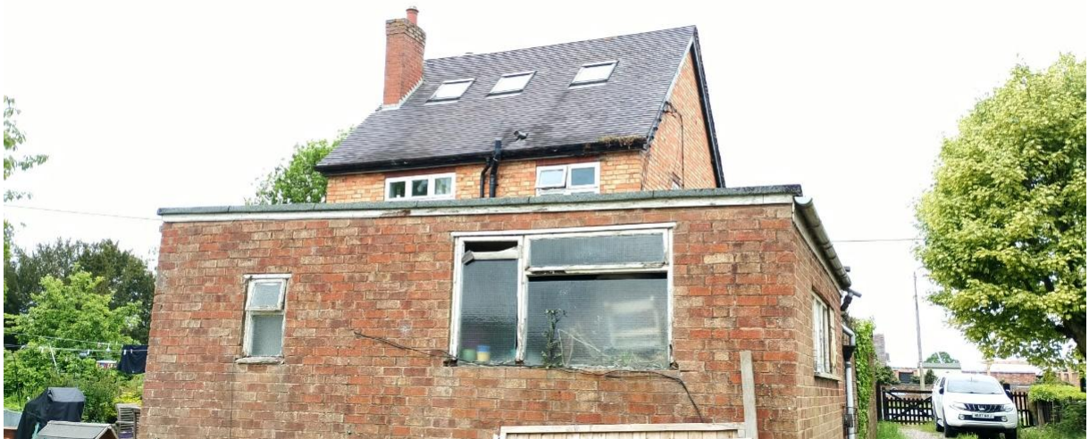
Photograph 11: Photograph of detached brick outbuilding elevation.
