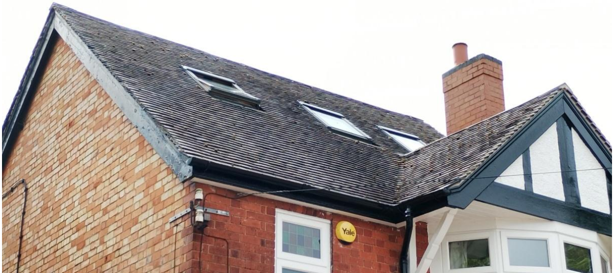
Photograph 14: Main dwelling roof and gable elevation.
