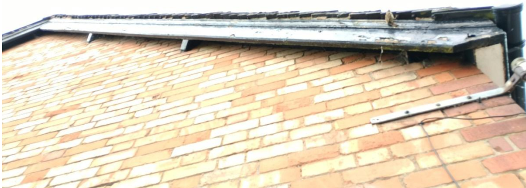
Photograph 10: View of fascias on external elevation.
