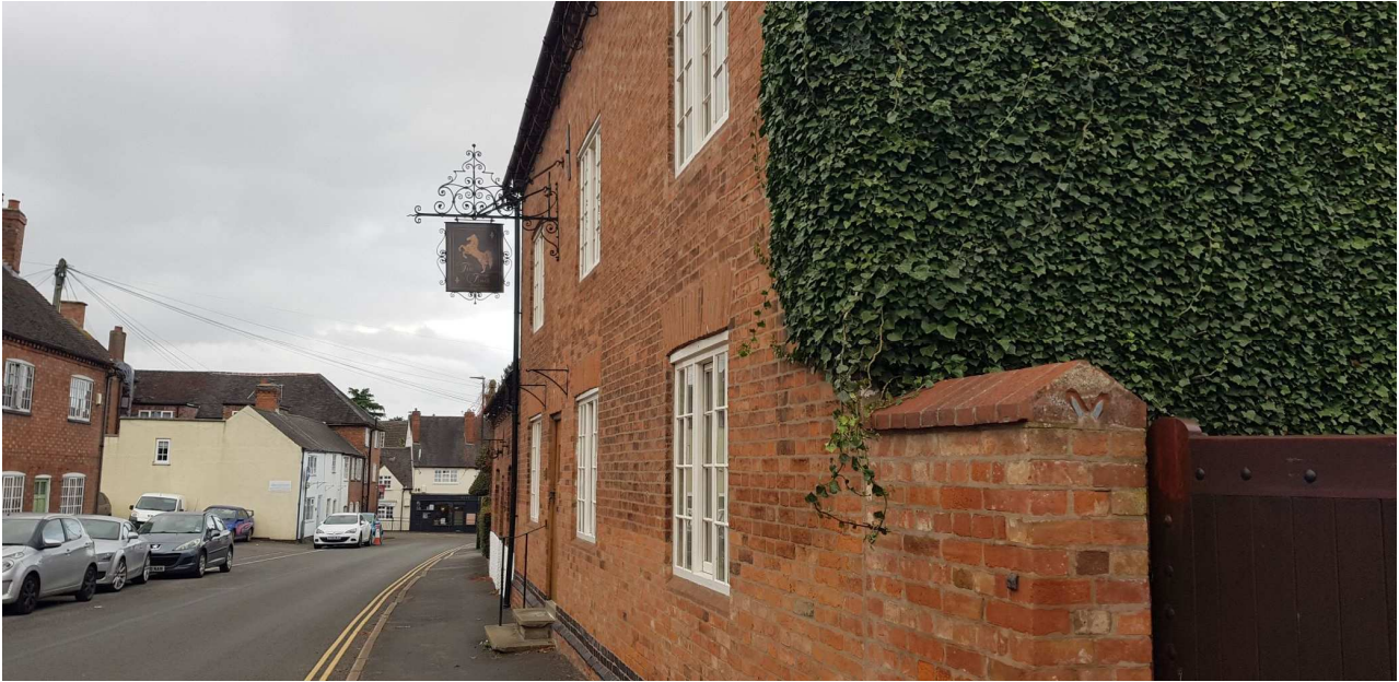
Photo 27 Front Elevation, Main House
