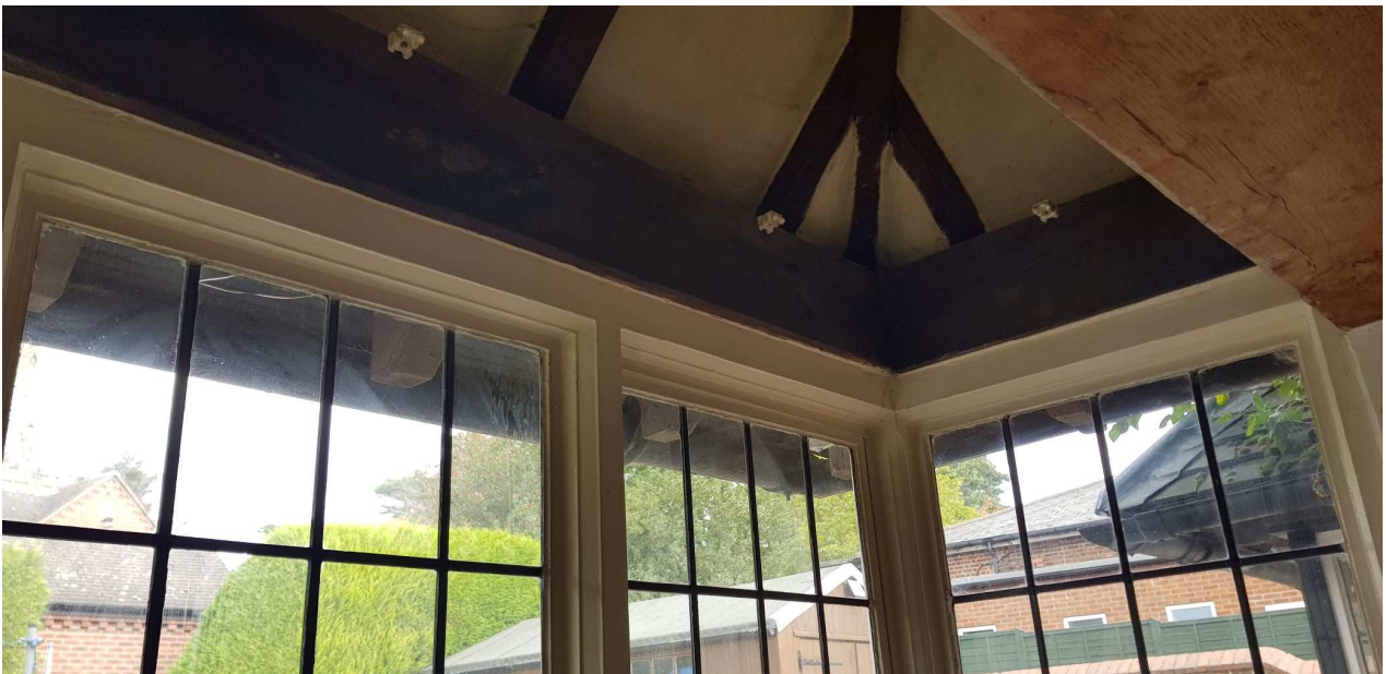
Photo 8 Structural Timber Framing to Bay Windows
