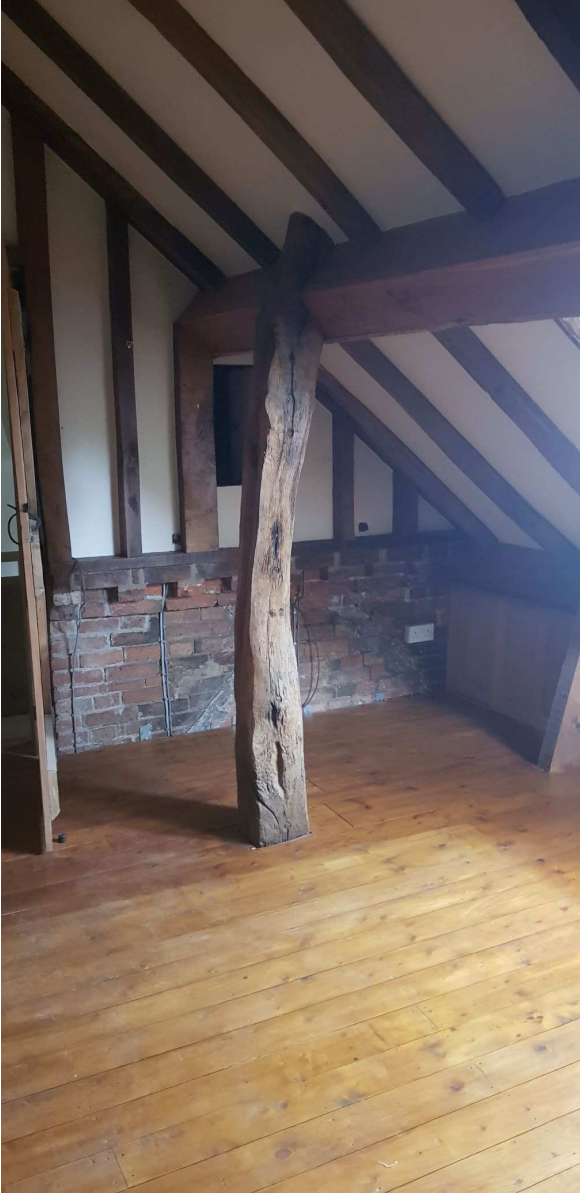
Photo 18 Second Floor Existing Timber Posts
