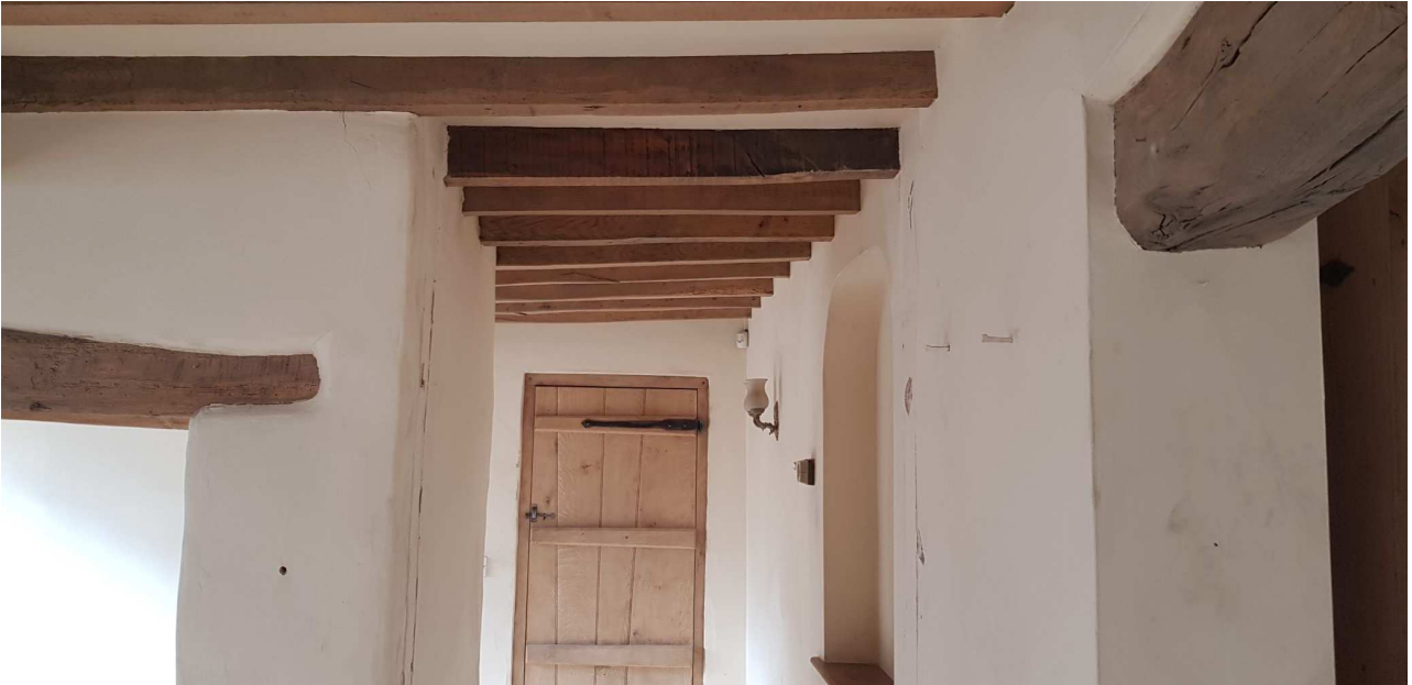
Photo 11 Sloping Ceiling in Kitchen
