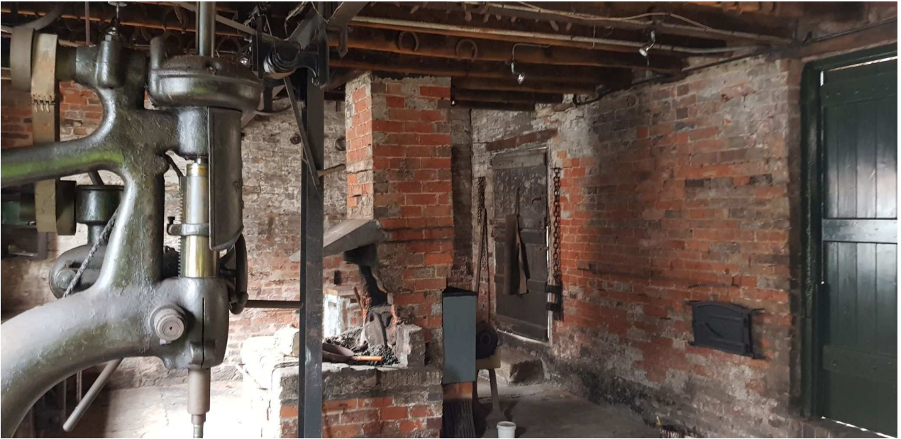
Photo 19 Internal View of Old Forge
