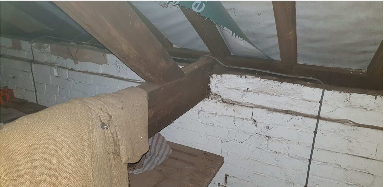
Photo 21 Old Forge Movement at Both Eaves
