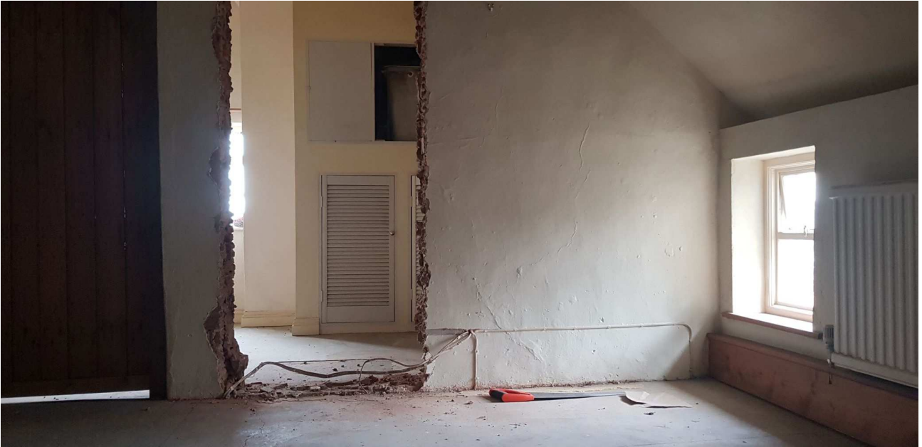
Photo 16 Second Floor Alterations Started
