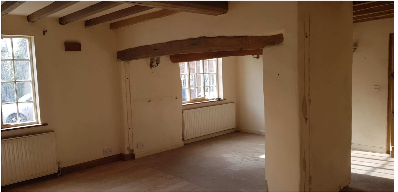
Photo 7 Timber Beams in Kitchen
