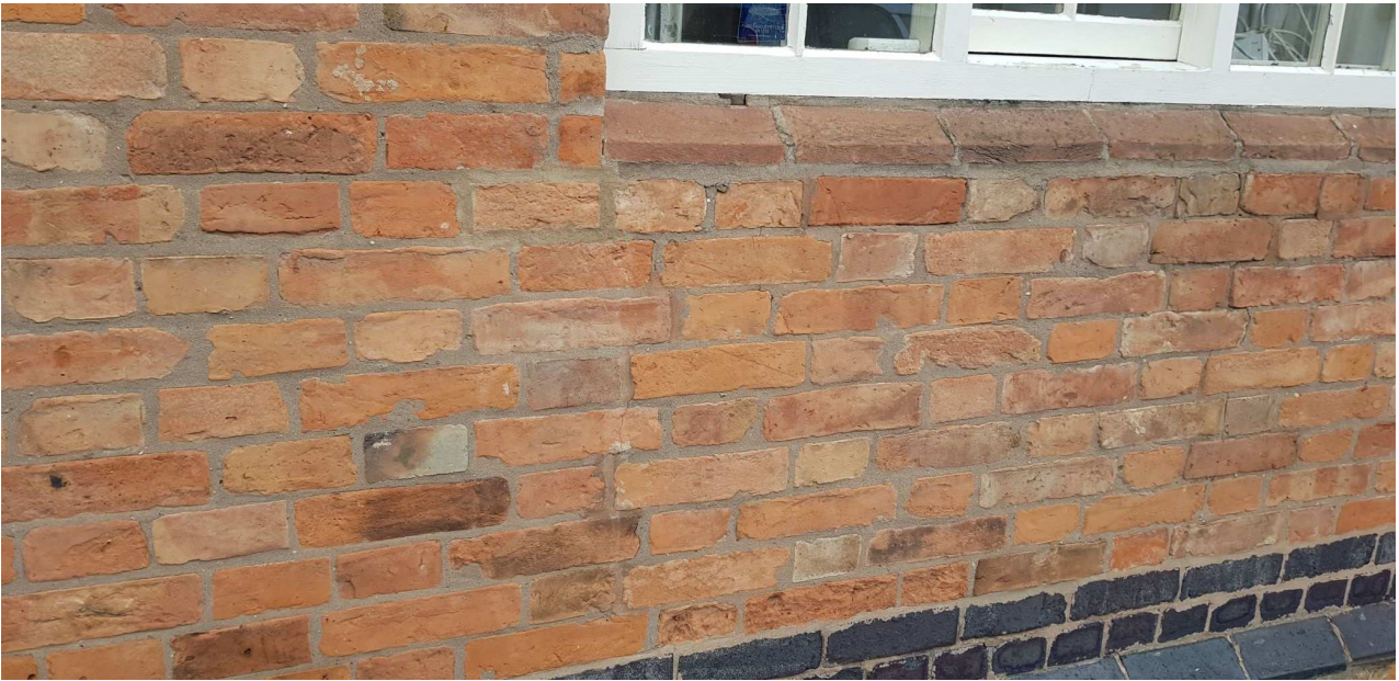
Photo 33 Previous Repointing of Front Wall
