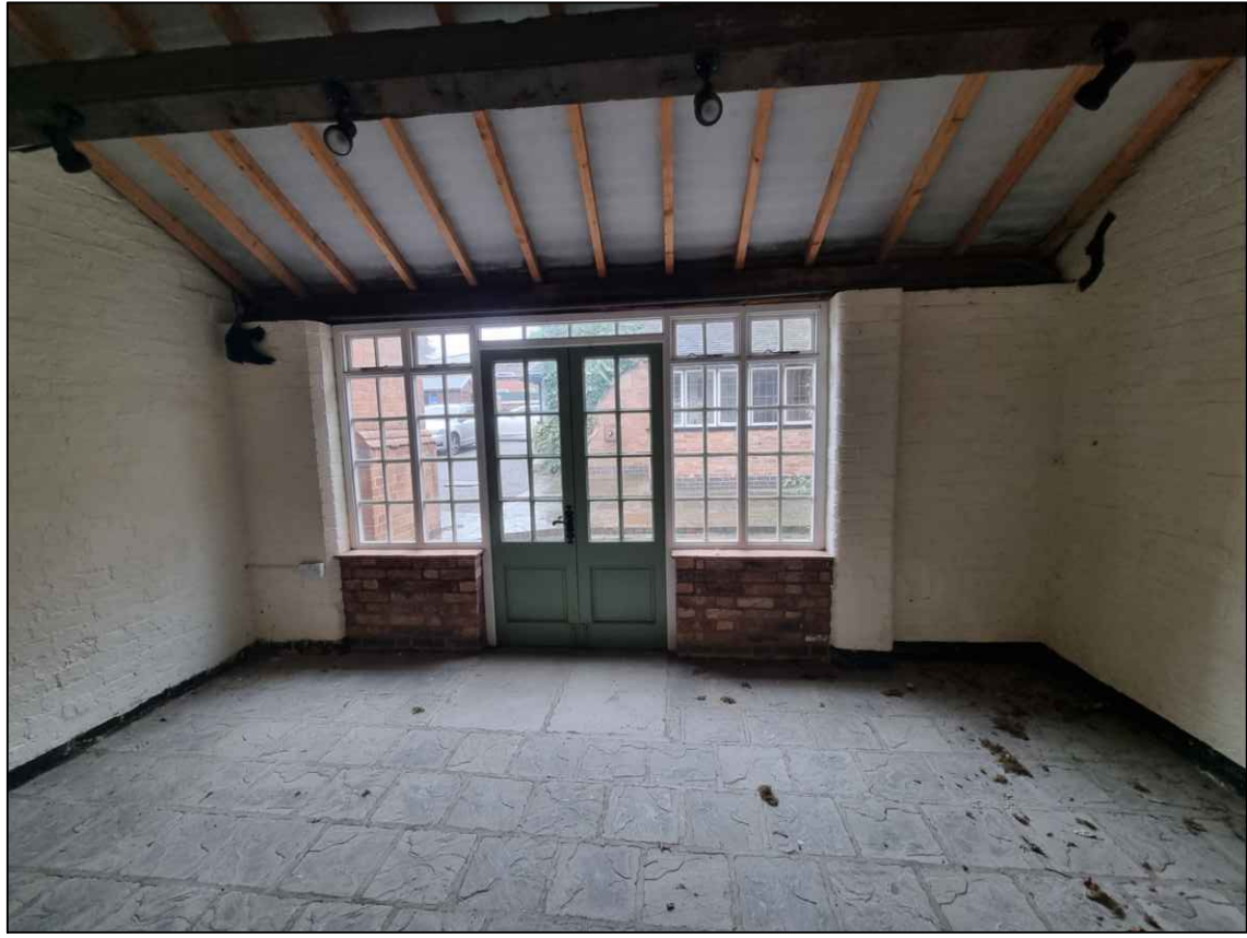
EXISTING INTERNAL IMAGE OF SERVERY - 6
