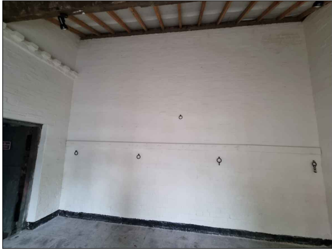
EXISTING INTERNAL IMAGE OF SERVERY - 8
