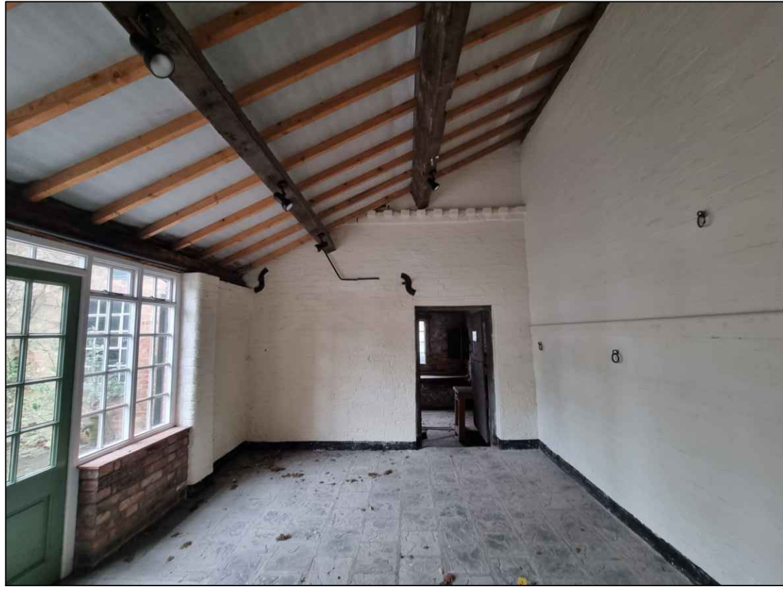
EXISTING INTERNAL IMAGE OF SERVERY - 7
