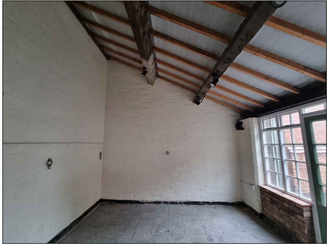
EXISTING INTERNAL IMAGE OF SERVERY - 5
