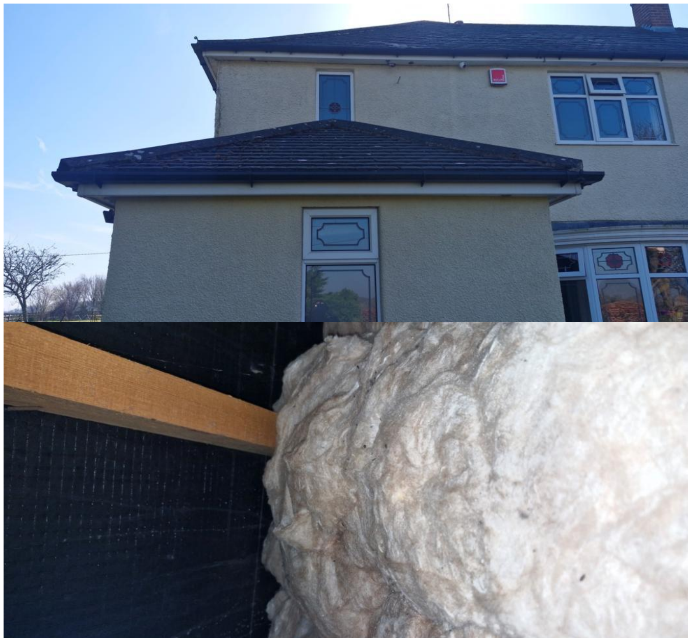
Front single storey with internal small loft image
