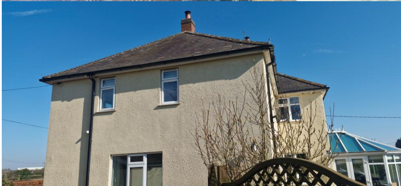
Main loft space and side elevation of building
