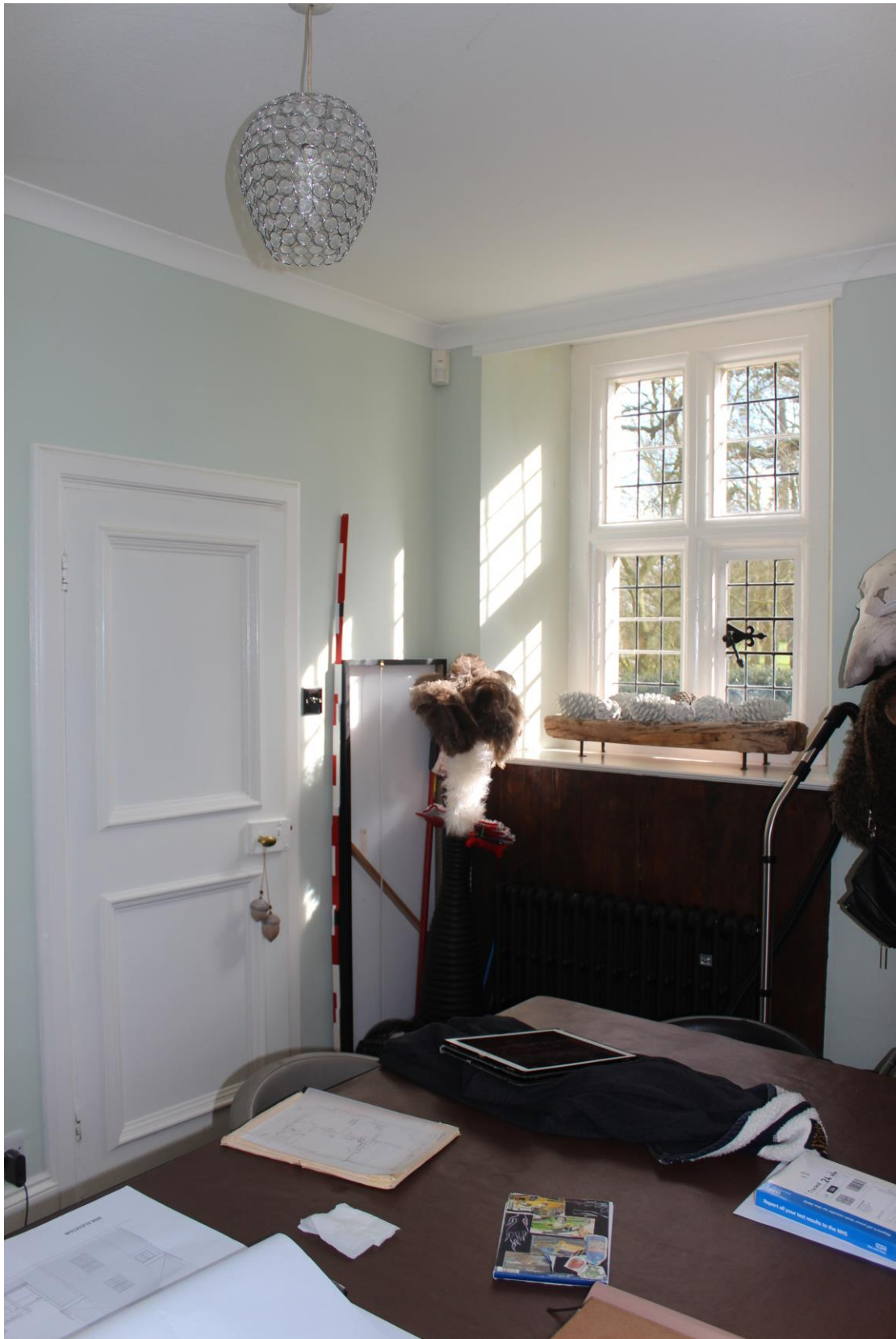
Plate 16: The dining room, showing a heavily moulded two-panel door, contrasting with the utilitarian doors on the 1st floor.
