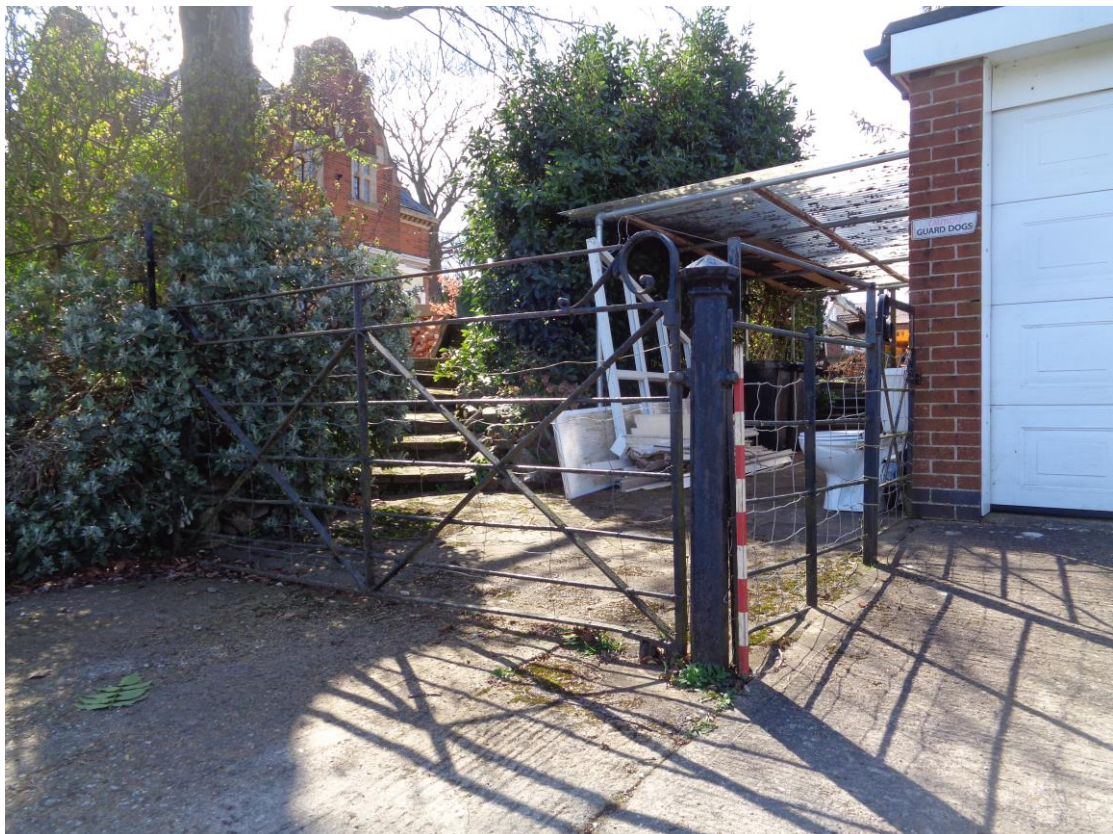
Plate 8: View of rear gates from northeast.
