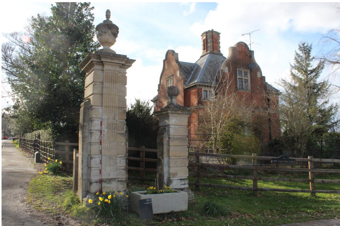
Plate 5: View of northern gate piers from southeast.
