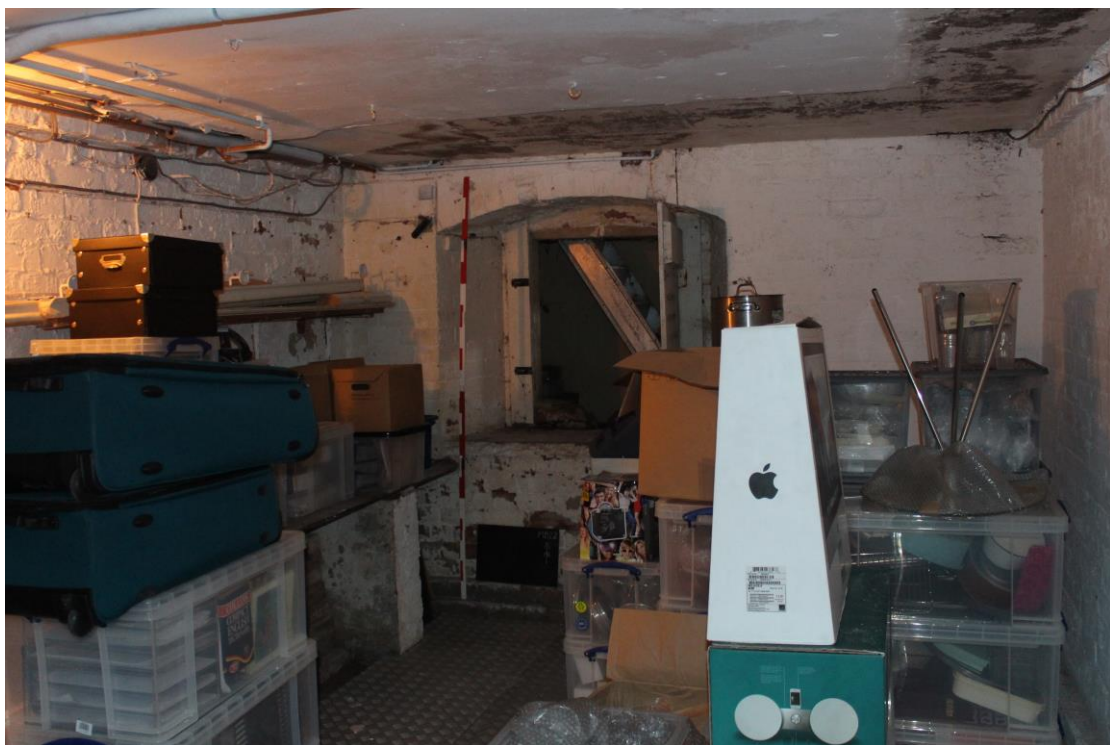
Plate 21: The cellar, showing the slate cold-shelf and the masonry of the casement window. The mullion was removed, a simple doorway added, and a short ladder inserted into the lightwell to provide external access.
