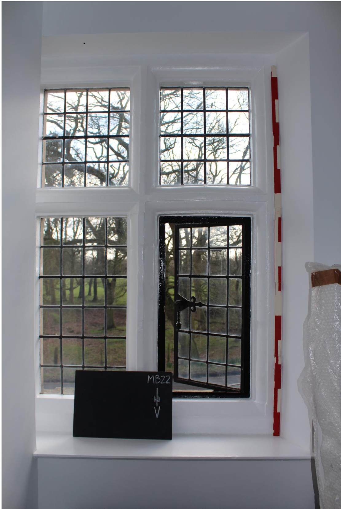
Plate 9: A 1st floor at the front partially blocked by an internal wall but preserving the symmetry of the front elevation.
