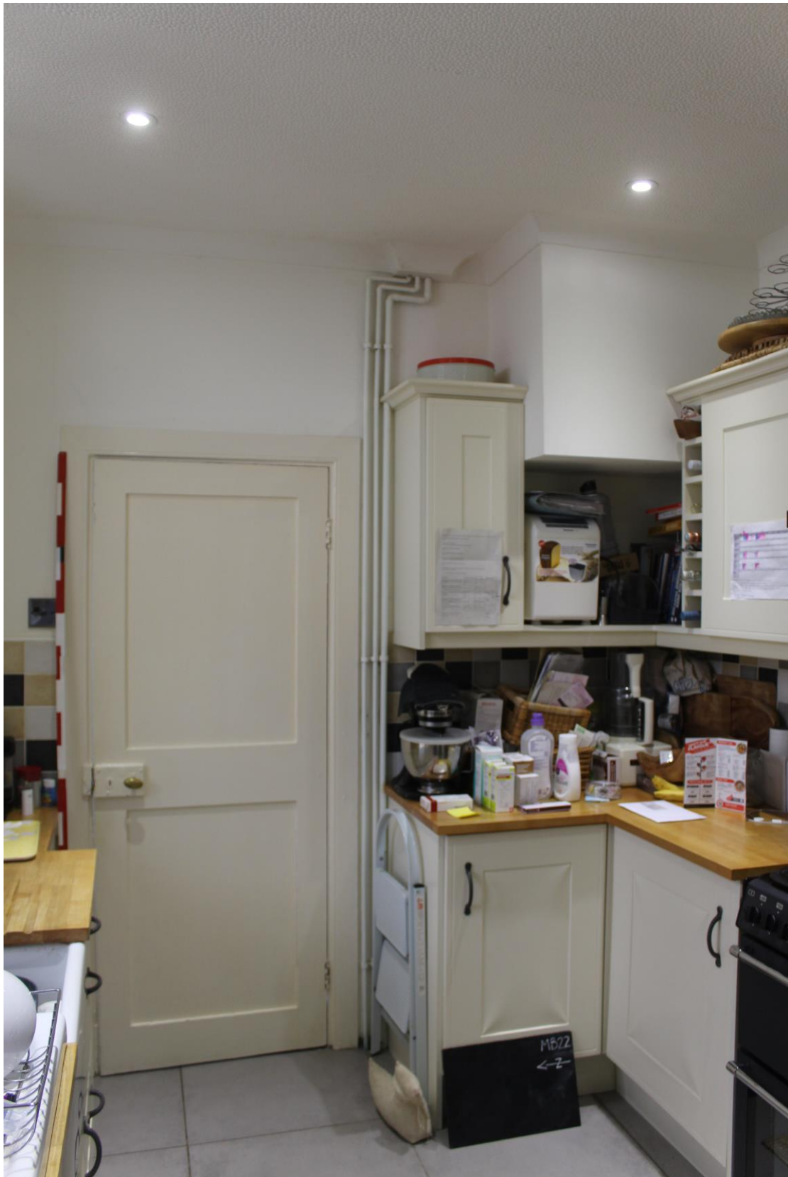
Plate 18: The kitchen showing an original utilitarian door and what appears to be the remains of a chimney flue over the site of a probable range.
