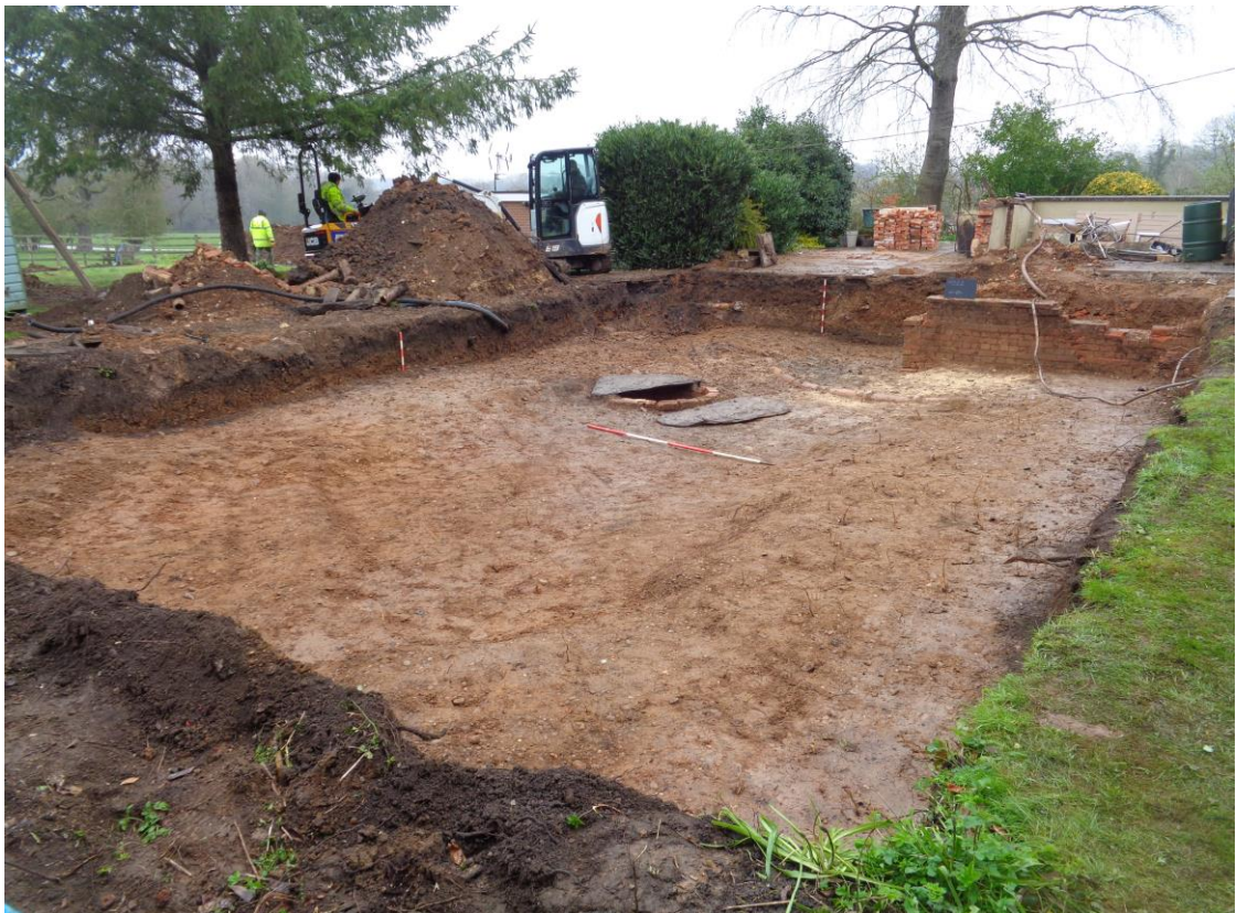
Plate 2: ASMSE area, view northeast.
