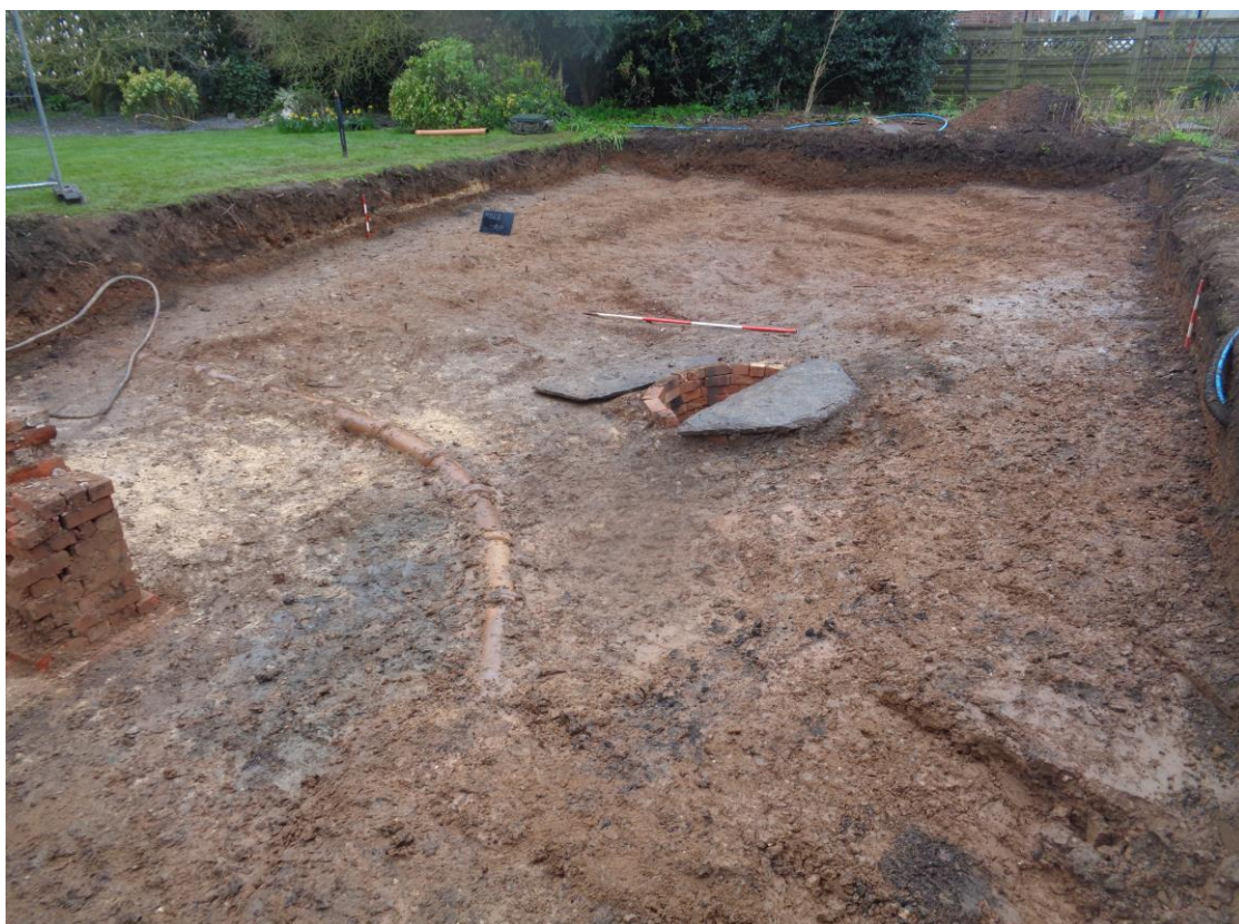
Plate 3: ASMSE area, view west.
