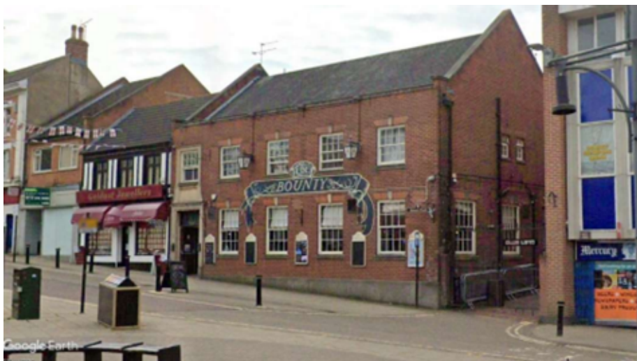
Figure 3. The replacement of the George Hotel. 1960.
