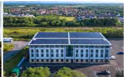
Roof mounted solar panels
