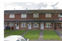
6 - Two-storey terraced houses
