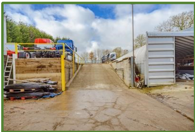
Fig.10 The appearance of the existing industrial site shall be enhanced through clearing materials, surface repairs and levelling of potholes, landscaping and planting elements, as well as sections of natural wood cladding (sustainable) to containers to blend with the surrounding woodland. Old industrial floodlights to be replaced with non-intrusive eco-friendly LED lighting.
