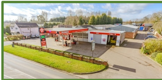
Fig.12a Ample existing access into site.
