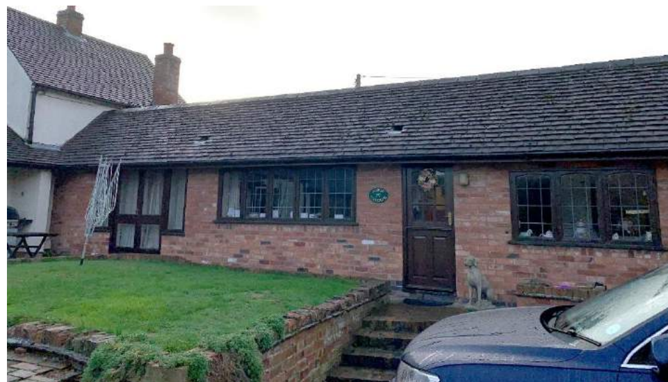
Looking South East from courtyard - single storey residential element
