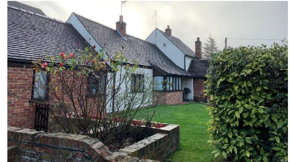
Looking South East from courtyard - white rendered dwelling
