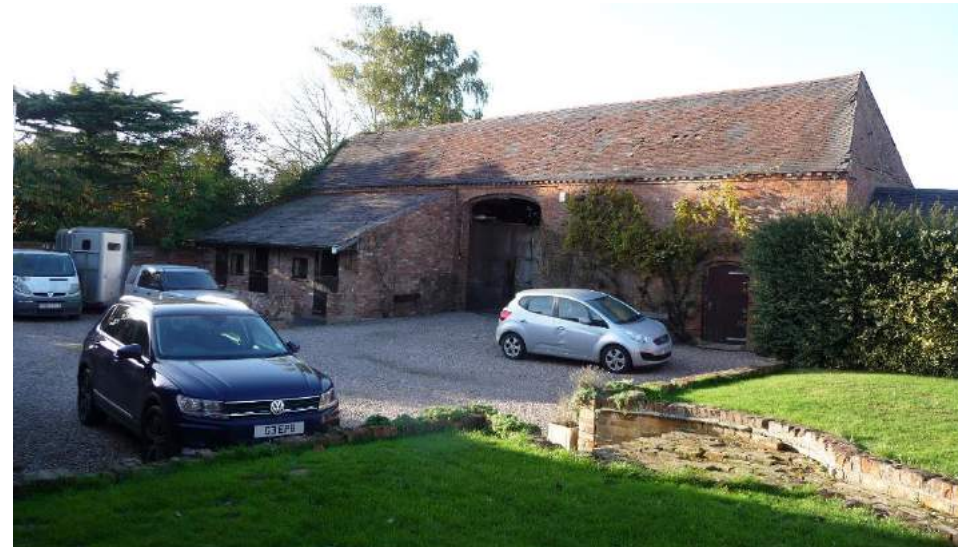
Main barn with lean too stables. Gravel courtyard and low level walls.
