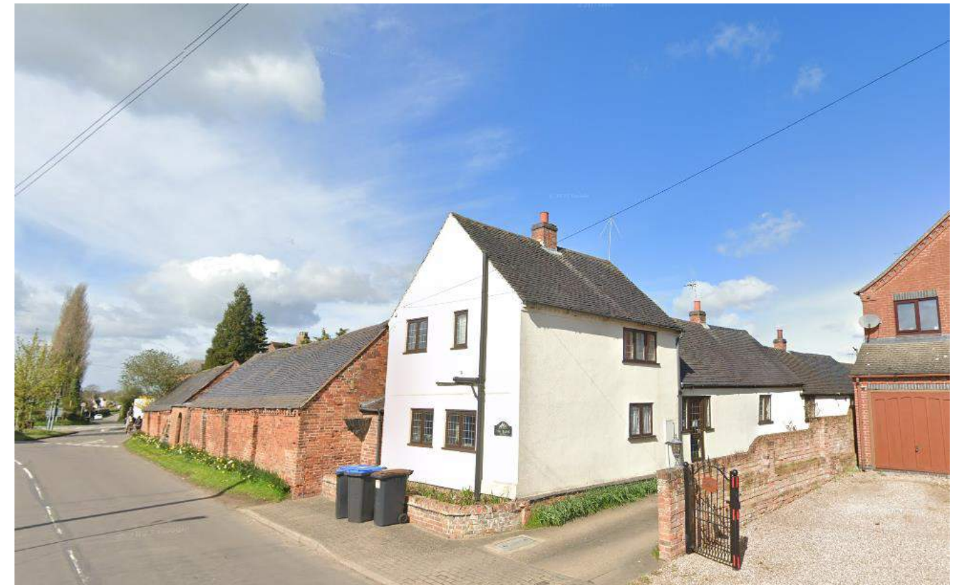
The Barns – viewed from Main St. Two storey element in the foreground.
