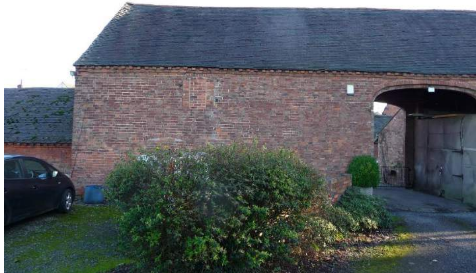
Looking South – Main Barn c/w courtyard access
