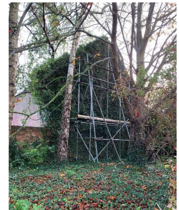
Threshing Barn gables – subject to structural movement / collapse. The barn requires significant investment to secure its useable future. The West gable is supported / braced by scaffold to counter movement due to tree root proximity
