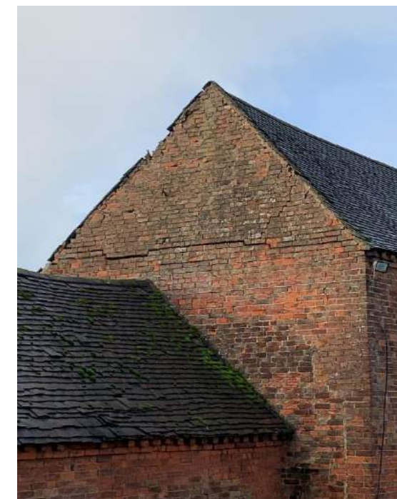
Threshing Barn gables – subject to structural movement / collapse. The barn requires significant investment to secure its useable future. The West gable is supported / braced by scaffold to counter movement due to tree root proximity
