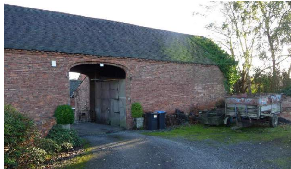
Looking South – Main Barn c/w courtyard access
