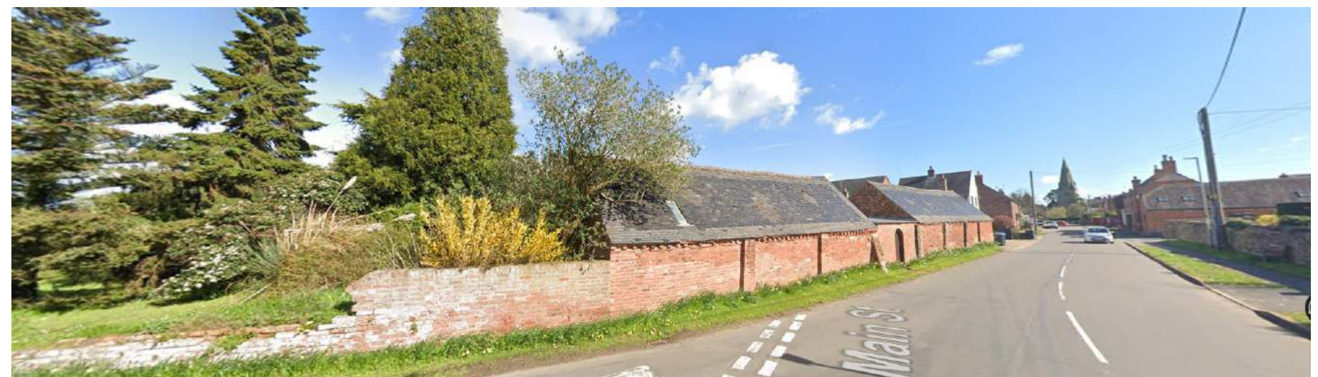
View of site from Main St. looking East (Site obscured by buildings and vegetation) Note section of corrugated roof to be removed.
