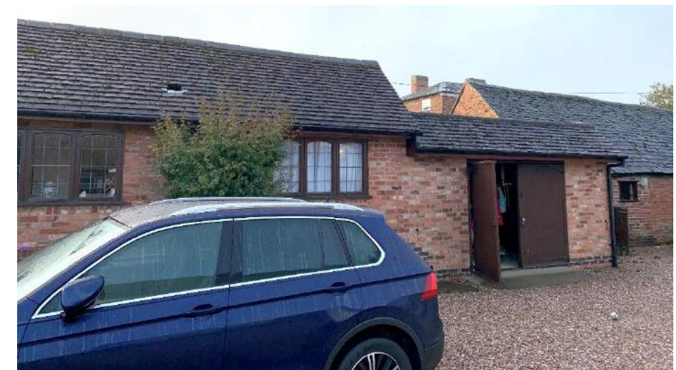
Looking South from courtyard - residential element and outbuildings
