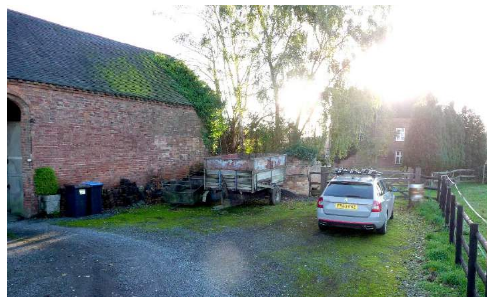
Looking South East from courtyard - single storey residential element
