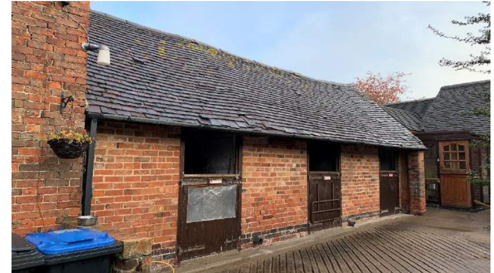
Looking North East from courtyard Stables to East end of main barn.
