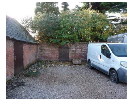
Pedestrian access off Ibstock Road
