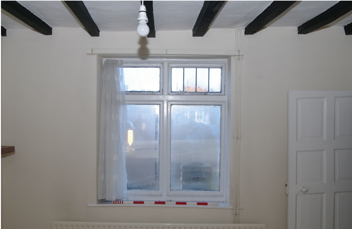
Figure 61: Room G5, window detail Looking south-west. 1m scale
