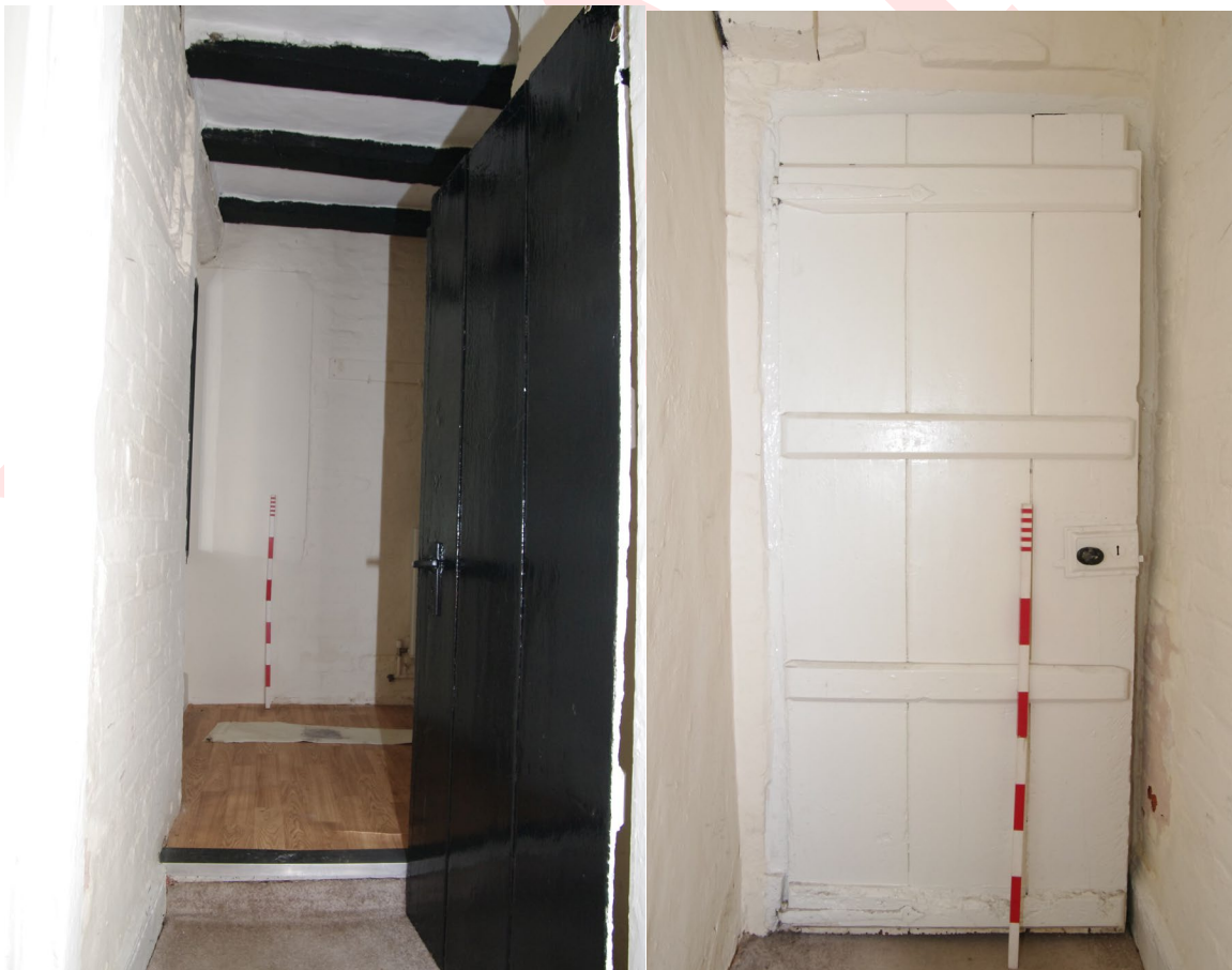
Figure 56: Room G4, doorway to Room G6 and flat-roofed extension The door is made of three wide planks. Left picture: Looking north-west. Right picture shows the northern face of the door. 1m scale
