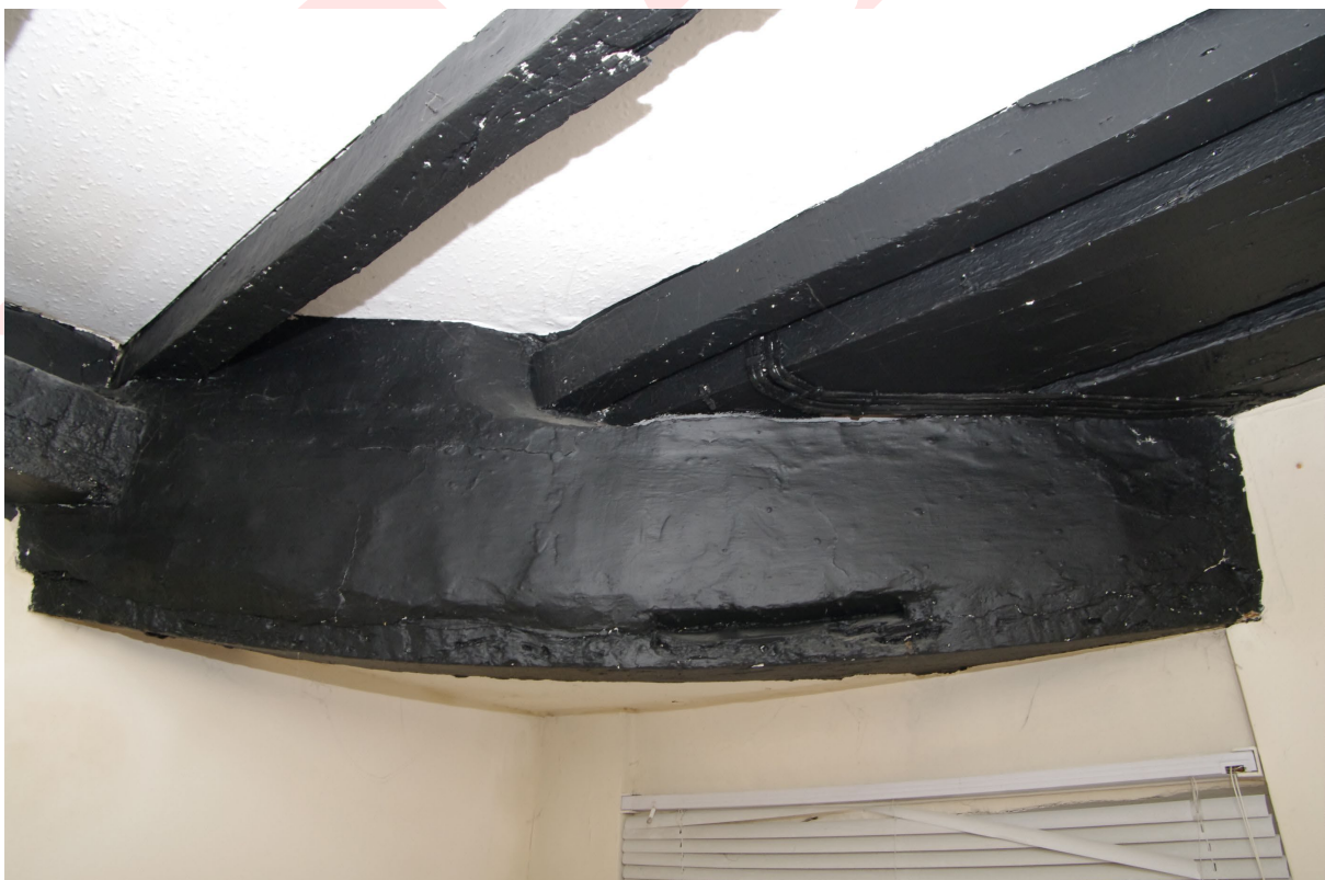
Figure 67: Room G5 within arched area, corner timber detail Looking east. The redundant sockets indicate reuse from elsewhere
