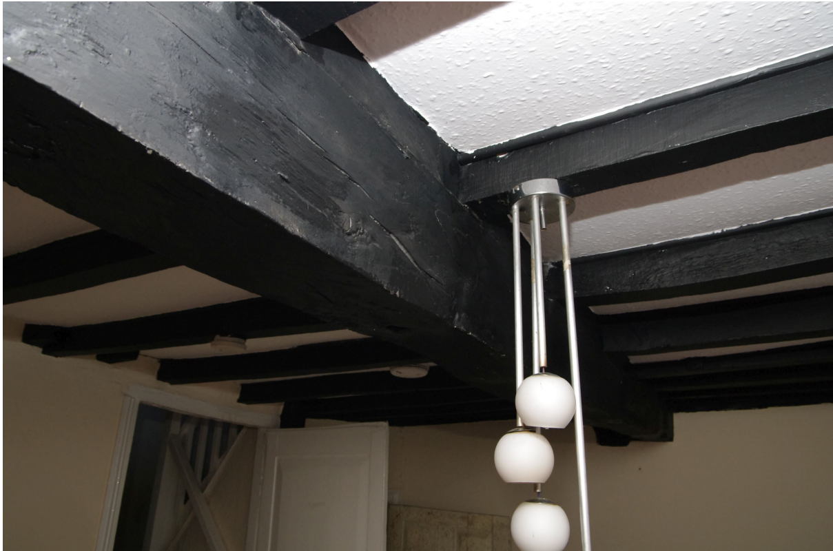
Figure 53: Room G4, axial beam detail Looking south-east
