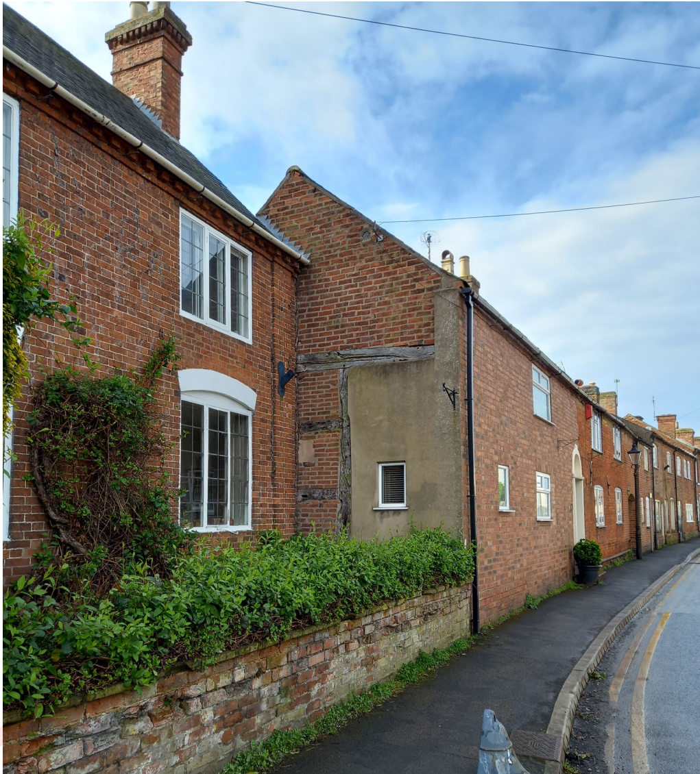
Figure 104: Example of a box framed house on Kirkby Road, Desford
