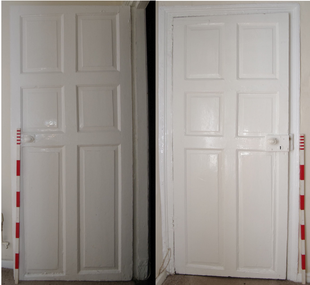
Figure 60: Room G5 door detail 1m scale
