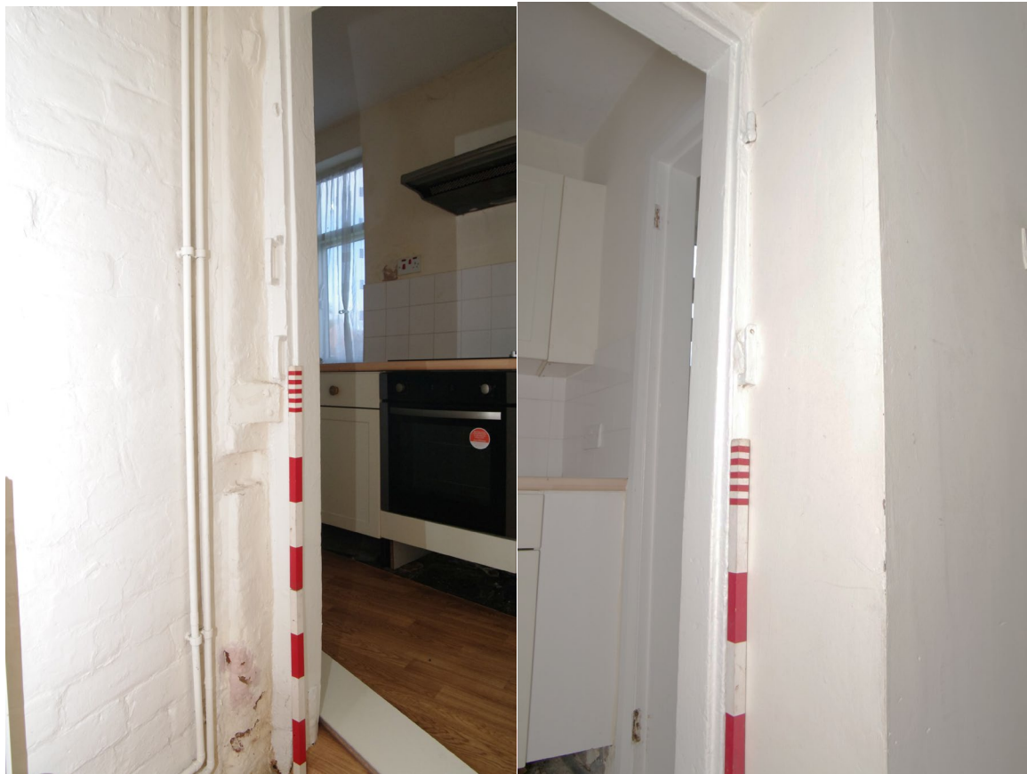
Figure 71: Room G6, doorframe detail Left: north side, right: south side. Both pictures looking north-east from G6
