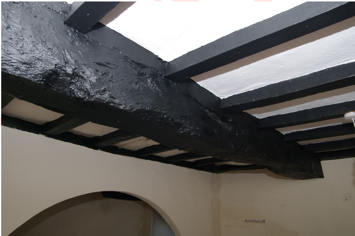
Figure 62: Room G5, axial beam detail Looking south-east
