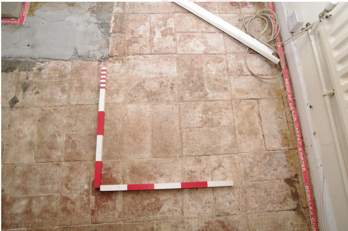
Figure 64: Room G5, brick floor detail 2 x 0.5m scales
