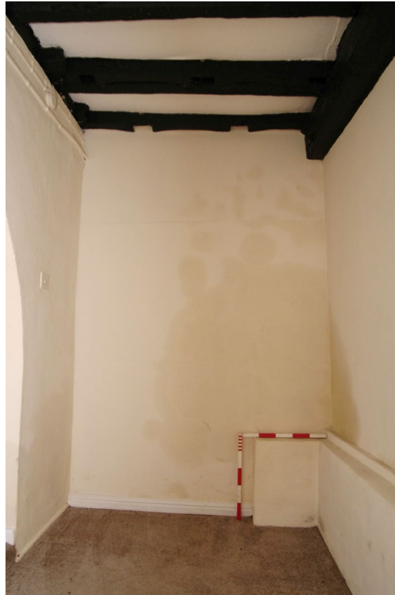
Figure 66: Room G5, within arched area Looking north-west. Note the thickened wall base and where it stops. Also the reused ceiling rafters. 2 x 0.5m scales
