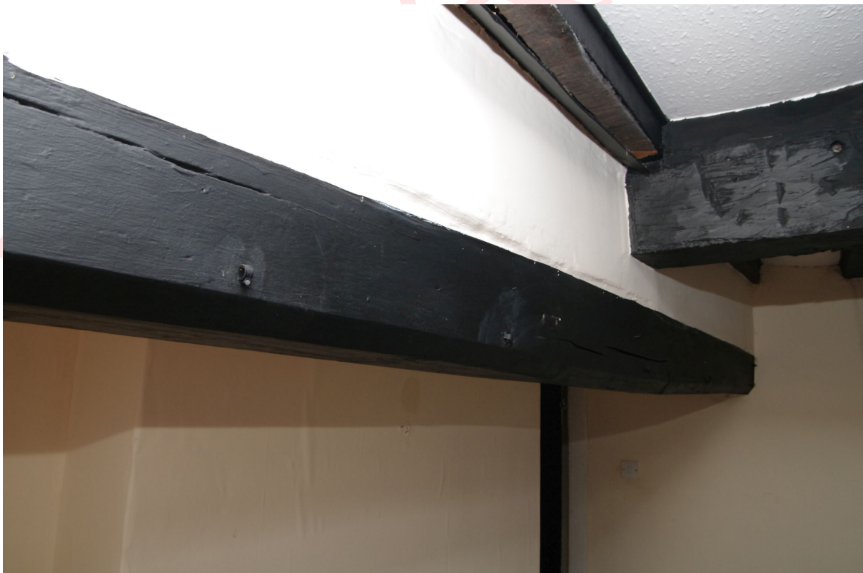
Figure 54: Room G4, bresumer beam detail Looking north-east
