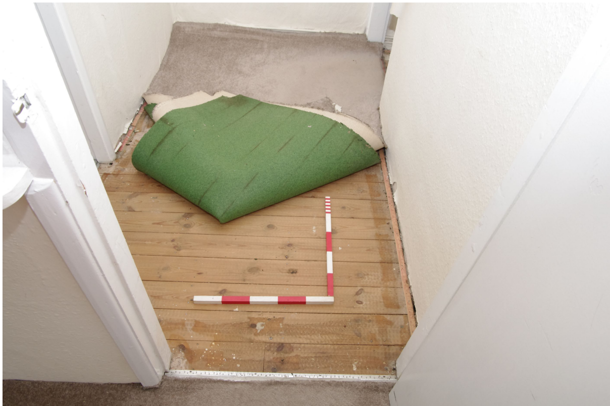
Figure 100: Room F8, location of former stairs from G1 Looking north-east from the doorway of F6. The doorway to bathroom F7 is on the left. 2 x 0.5m scales
