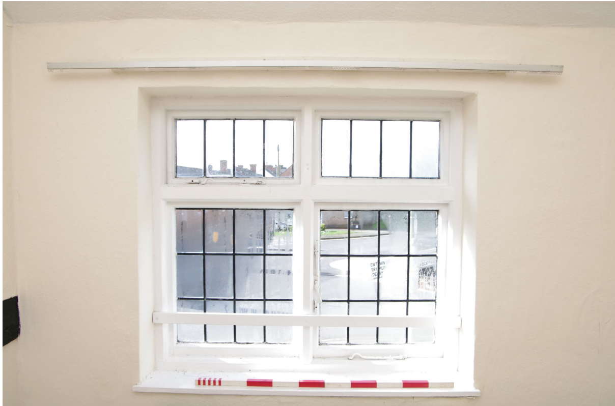
Figure 90: Room F4, window detail Looking south-west. 1m scale
