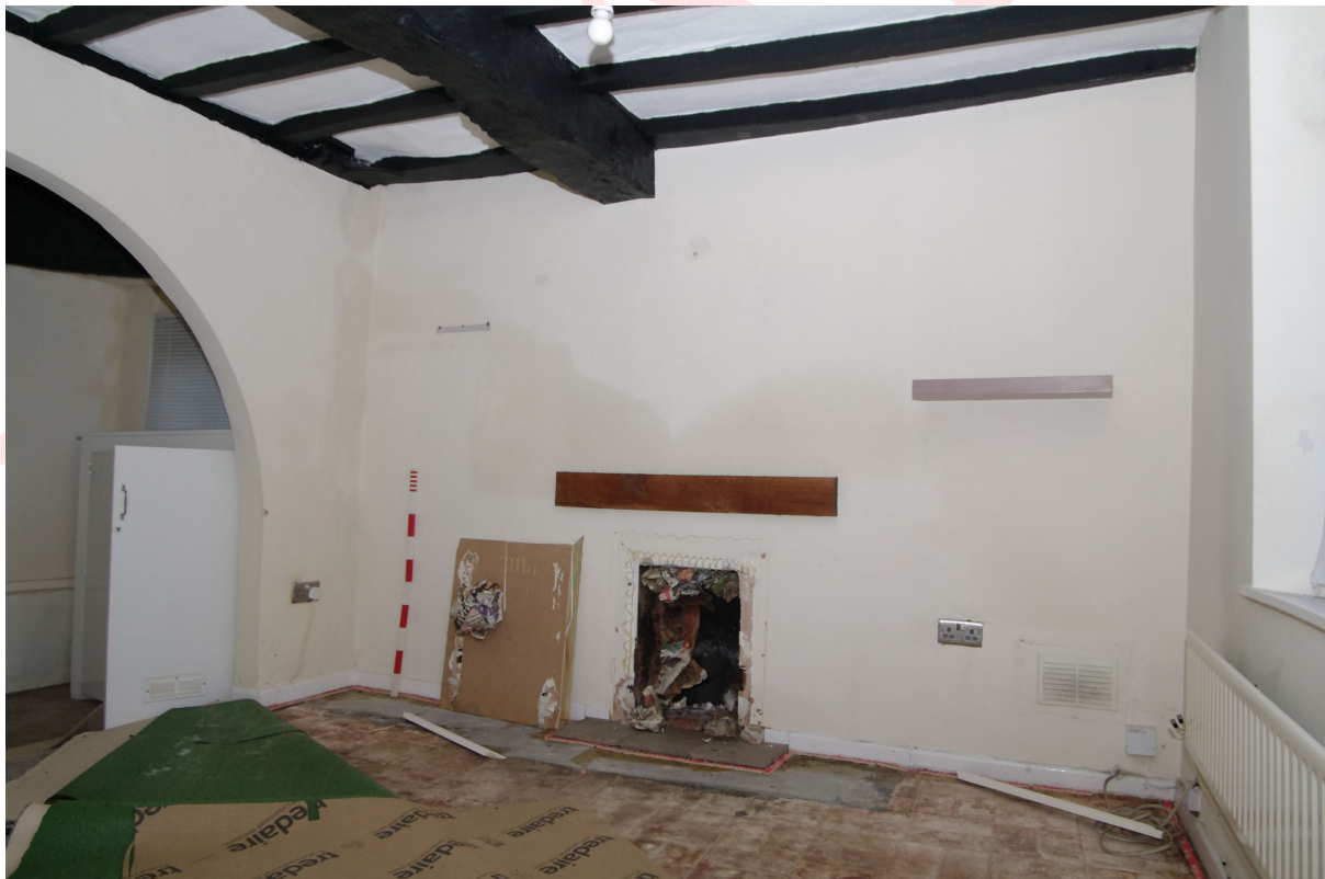
Figure 57: Room G5, fireplace Looking south. Note the archway on the left. 1m scale
