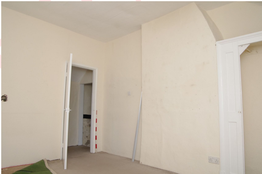
Figure 93: Room F5, general view Looking east. Note the mark on the chimney breast of a former blocked fireplace. 1m scale
