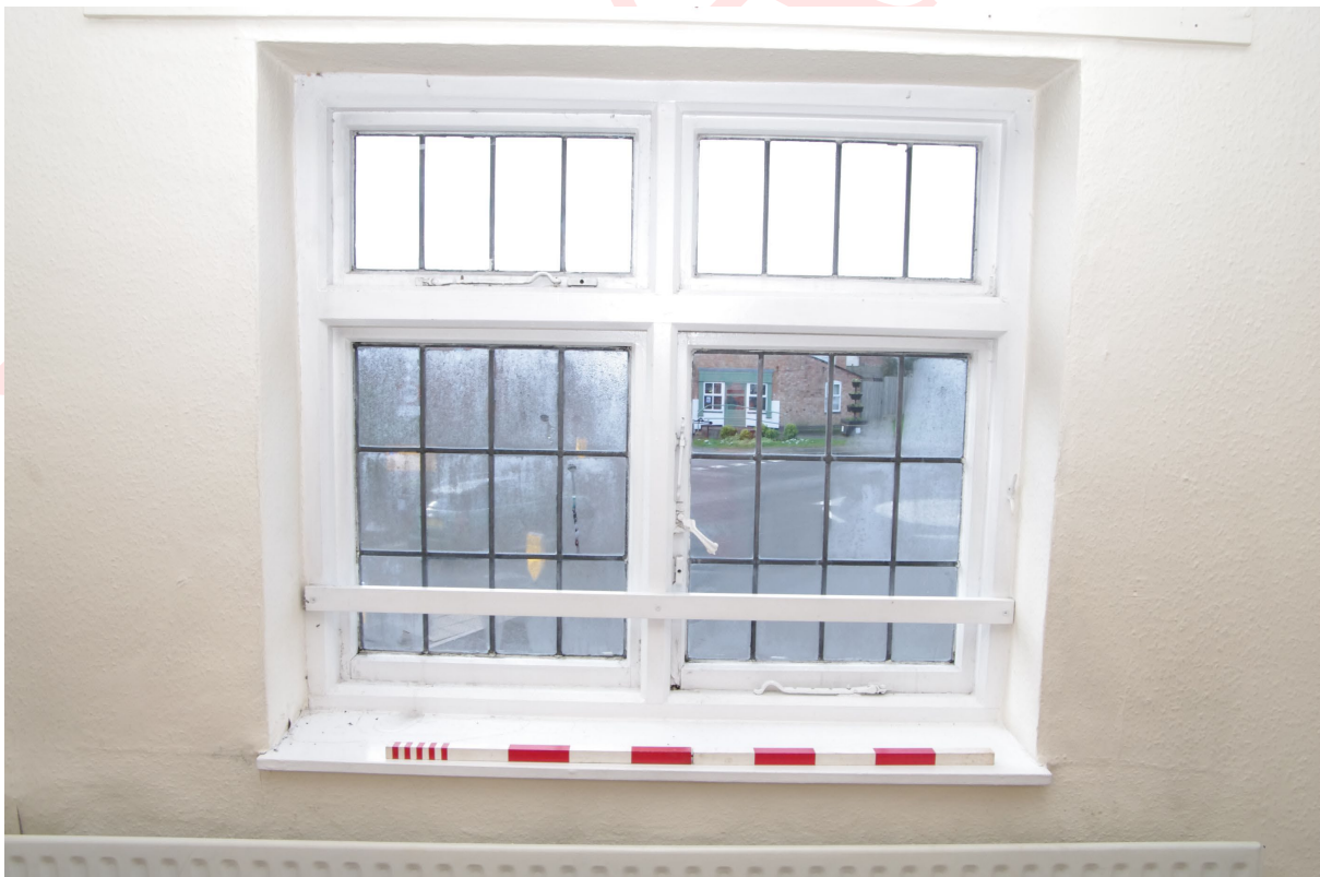
Figure 83: Room F1, western window detail Looking south-west. 1m scale
