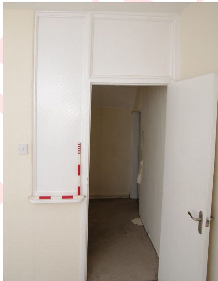
Figure 96: Room F6, doorway detail Looking north-east. The two recessed panels are painted-over glass. 2 x 0.5m scales
