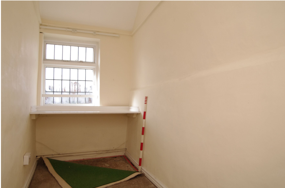
Figure 85: Room F3, general view Looking west. Note the top of the timber beam just above the tip of the 1m scale
