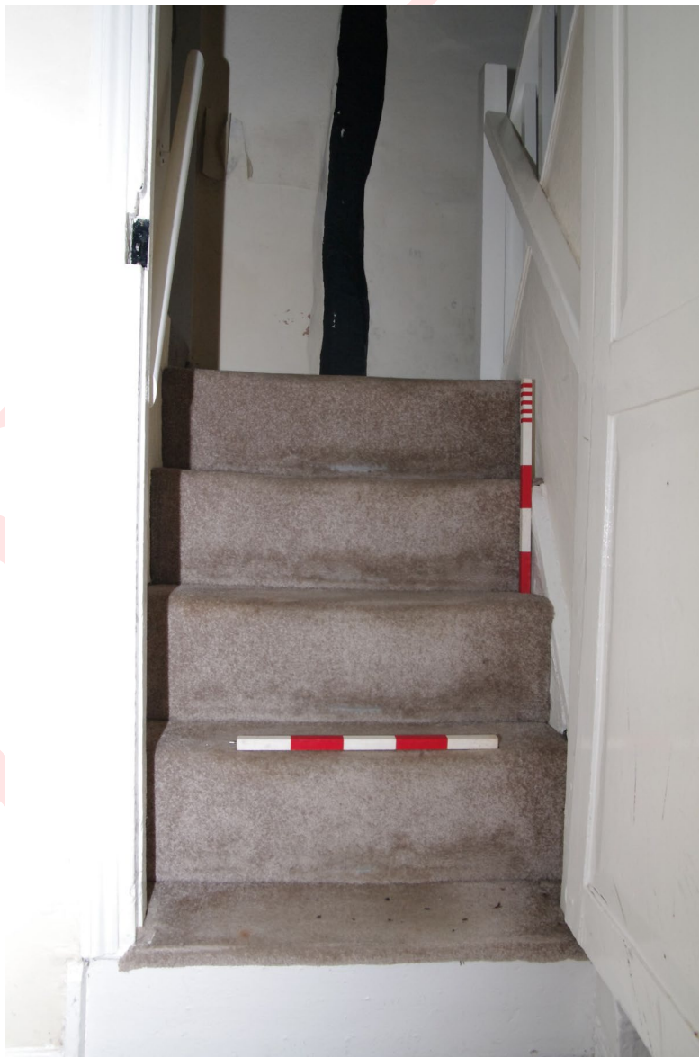
Figure 75: First flight of steps up to first floor Looking north-east. 2 x 0.5m scales
