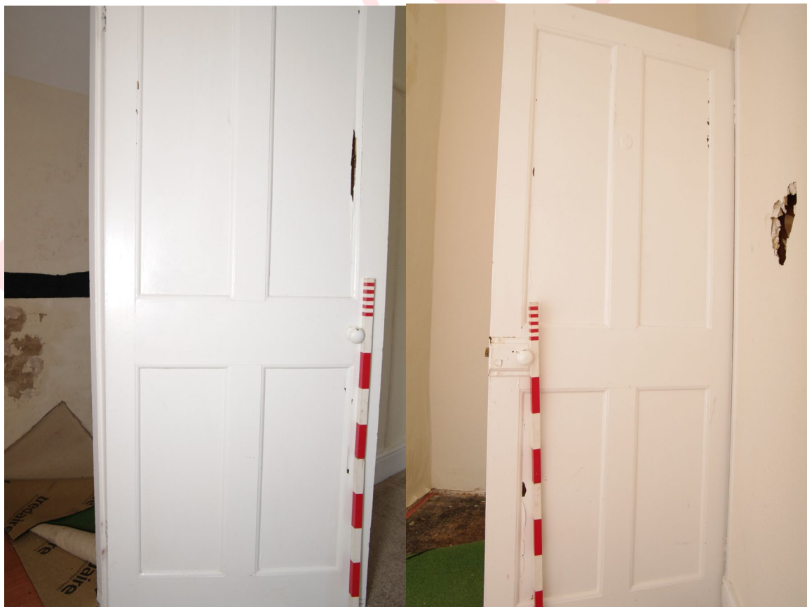
Figure 91: Room F4 door detail Left: landing facing side, right: internal face. 1m scale
