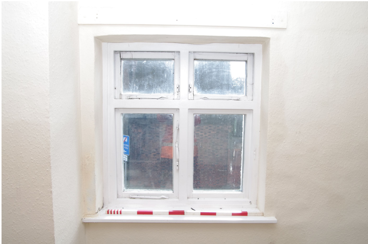
Figure 84: Room F2, southern window detail Looking south-east. 1m scale
