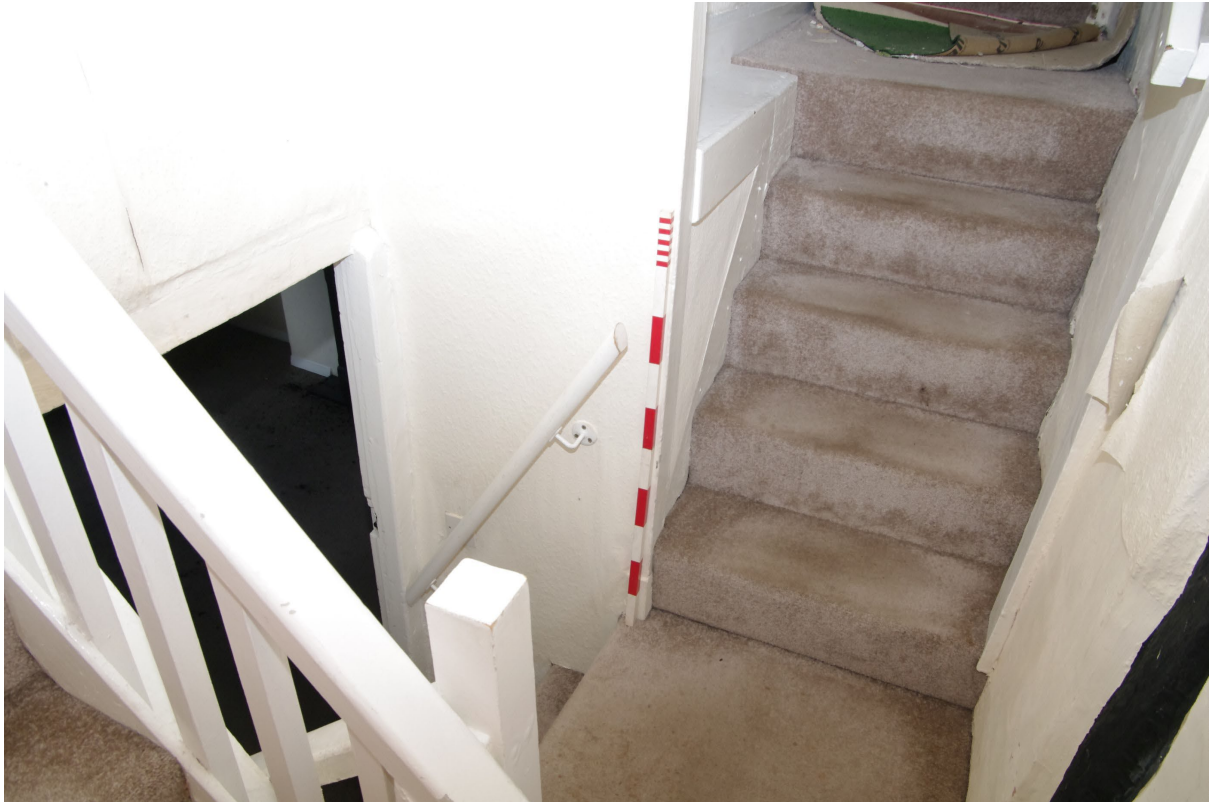
Figure 79: Room F1, steps up to F8 Looking north-west. Door down to ground floor on the left. 1m scale
