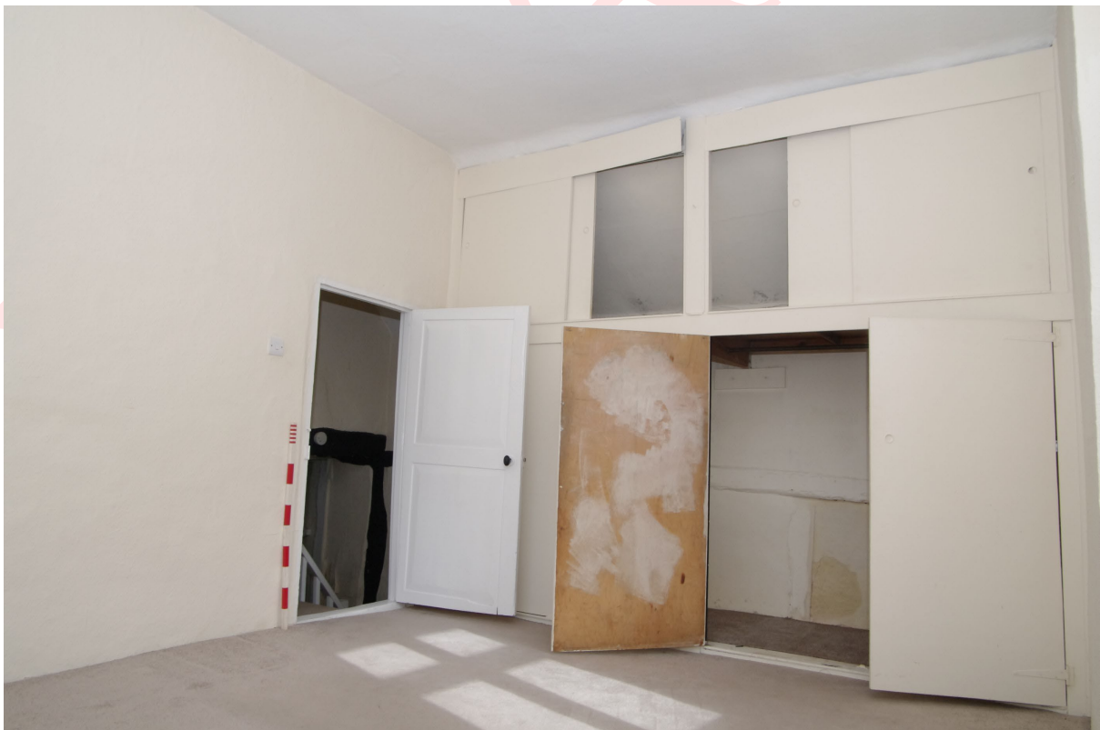
Figure 81: Room F2, general view Looking north-east. Note the timber frame within the wardrobe. 1m scale
