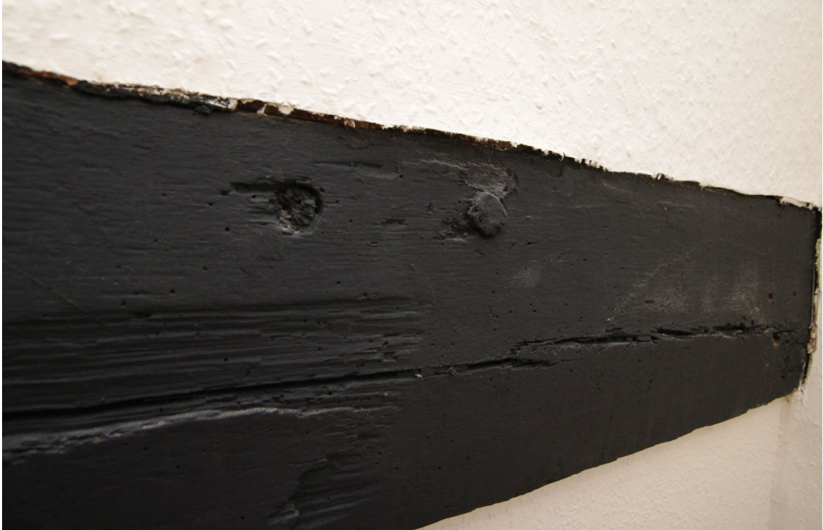
Figure 88: Room F4, detail of wooden pegs in the timber beam
