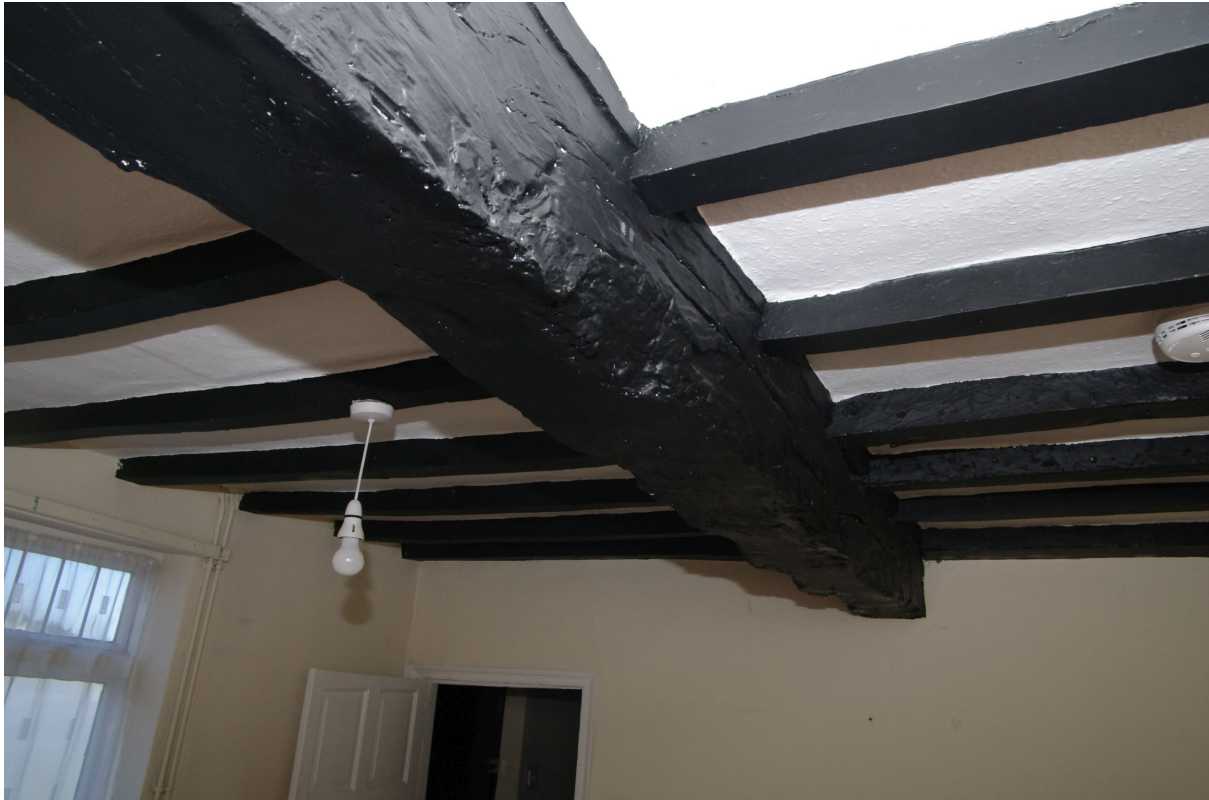
Figure 63: Room G5, axial beam detail Looking north-west
