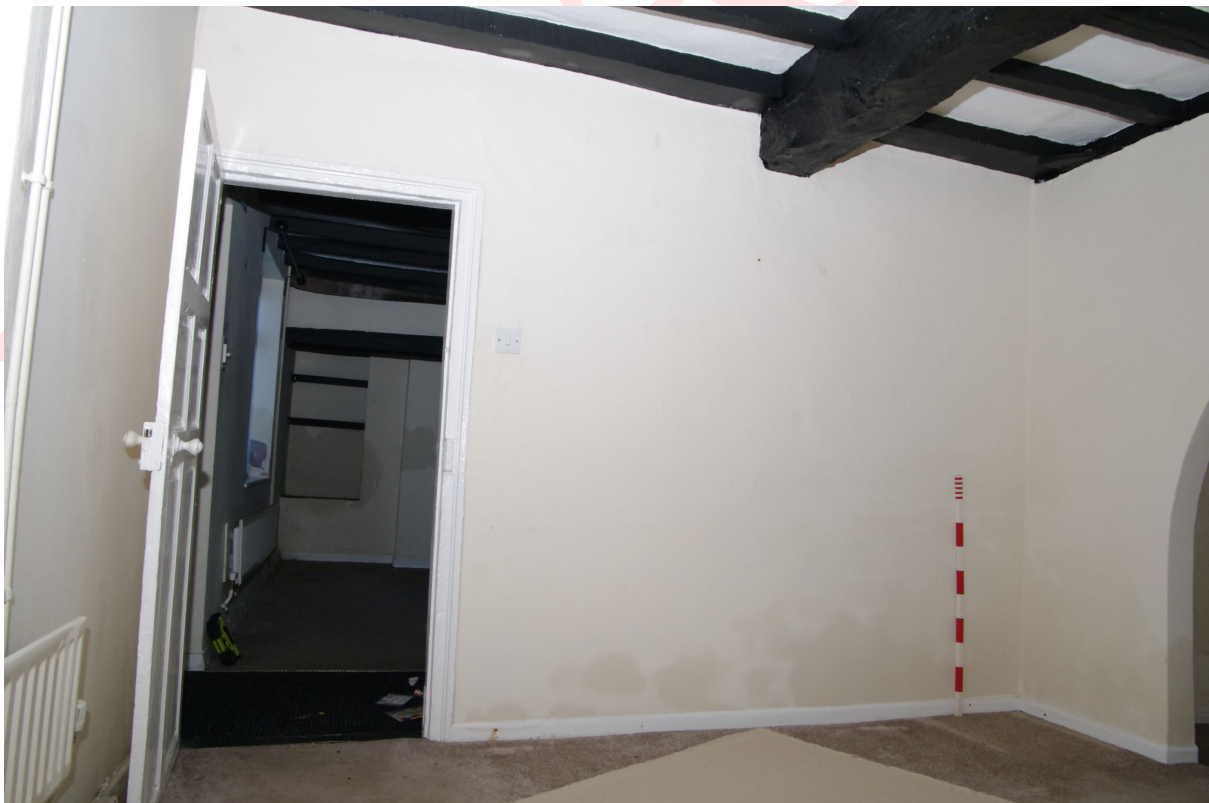
Figure 59: Room G5, general view Looking north-west. Doorway into Room G4. 1m scale
