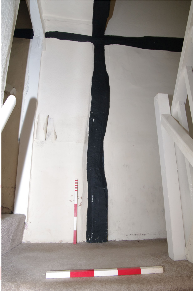
Figure 76: Room F1 timbers in the wall Looking north-east. Steps up to F8 on the left. 2 x 0.5m scales
