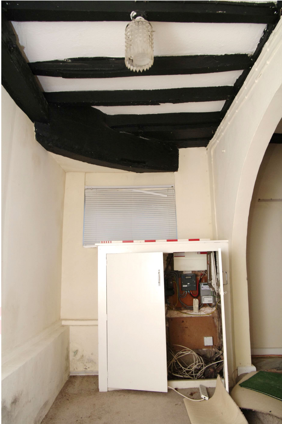
Figure 65: Room G5, within arched area
