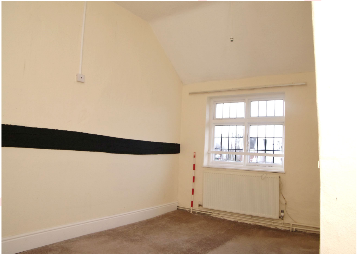
Figure 87: Room F4, general view
