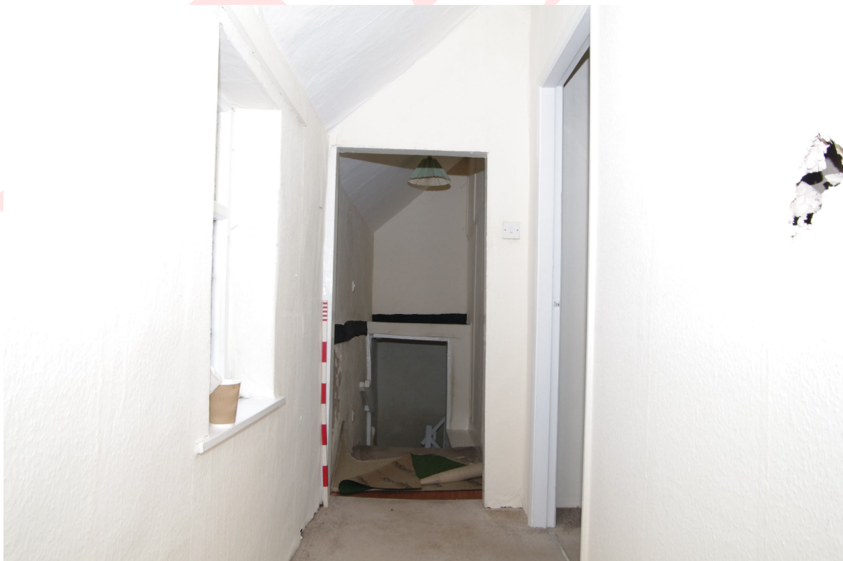
Figure 101: Room F8, general view Looking south-east. Stairs down to ground floor in the distance. Door to F5 to the right. 1m scale
