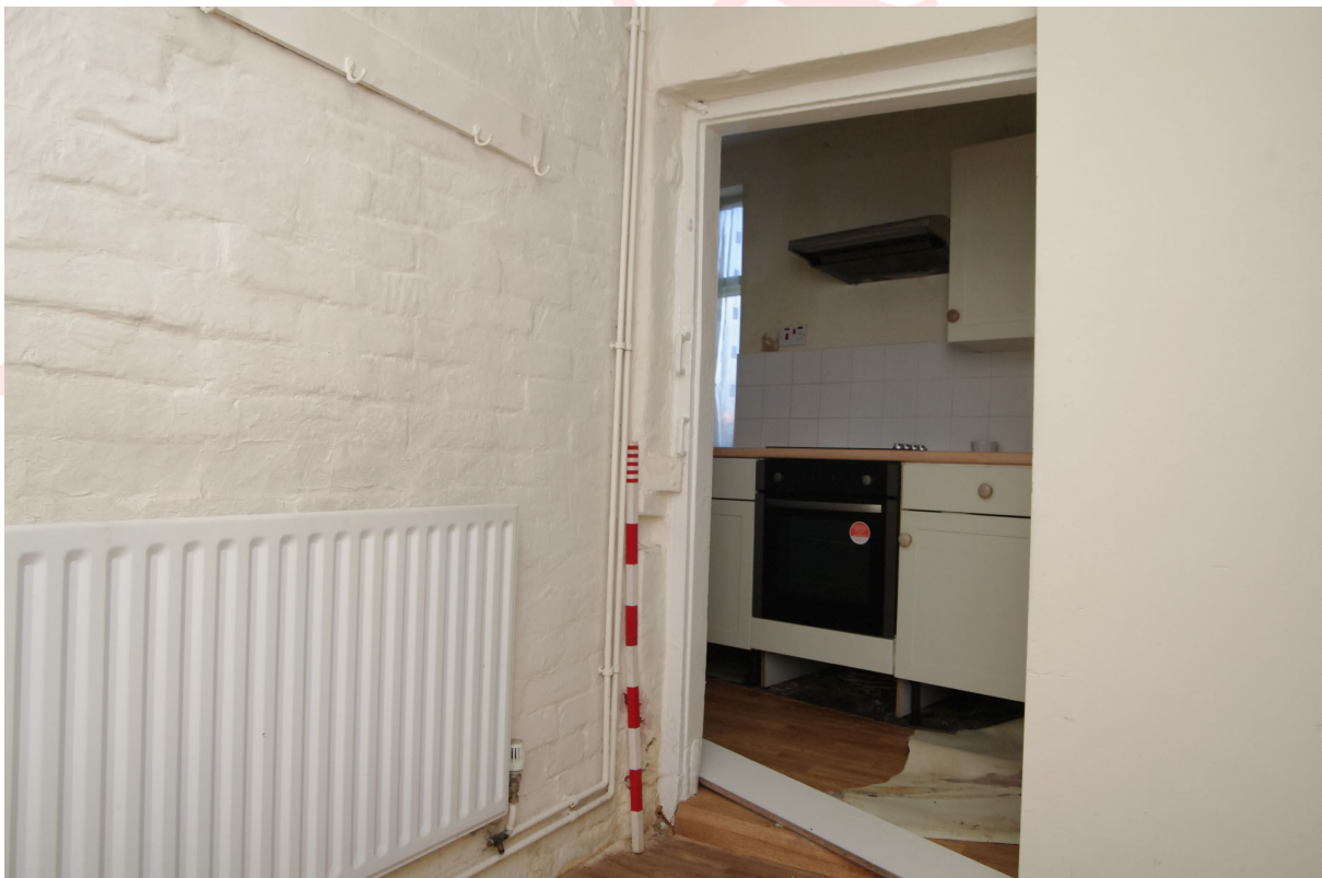
Figure 70: Room G6 looking towards doorway to G7 Looking north. Note the brackets on the door frame. 1m scale
