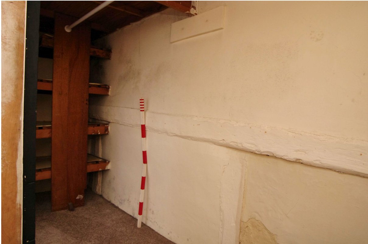
Figure 82: Room F2, timber frame on eastern wall Looking north-east. This continues through to Room F1. 1m scale
