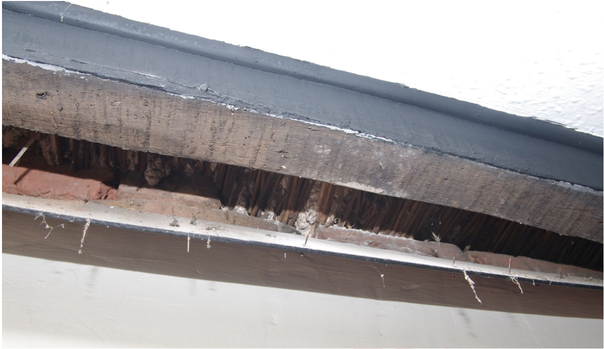
Figure 55: Room G4, underside of reed and gypsum floor detail behind bresumer beam Looking north-east up towards the ceiling
