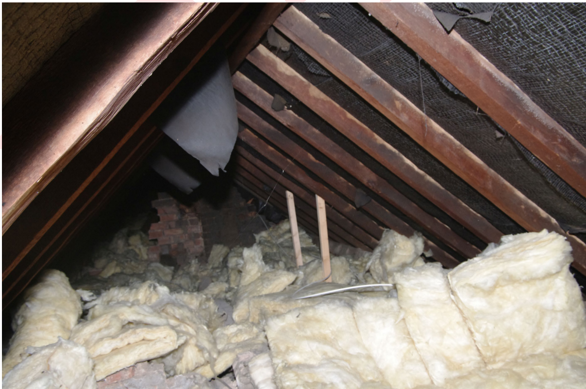
Figure 99: Room F7, roof space Looking south-west through loft hatch in F7
