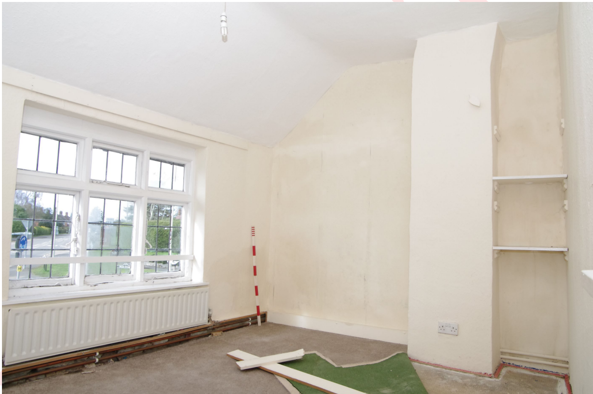
Figure 94: Room F6, general view Looking north-west. 1m scale
