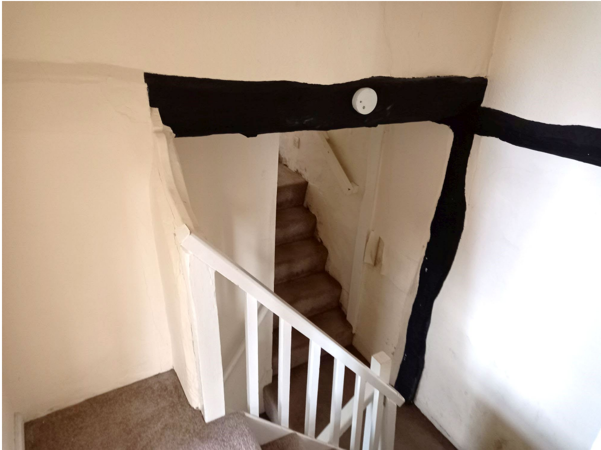
Figure 77: Room F1, timber frame
