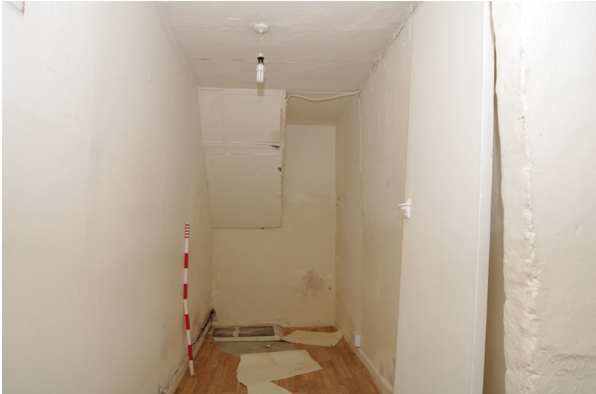
Figure 69: Room G6, space above the cellar and beneath the first floor landing Looking south-east. Note the narrow sloping section which is the underside of the stairs. 1m scale
