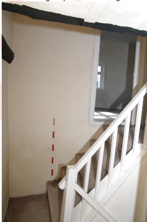
Figure 78: Room F1, steps up to F2 and F3 Looking south. Doorway to F2 in centre. 1m scale
