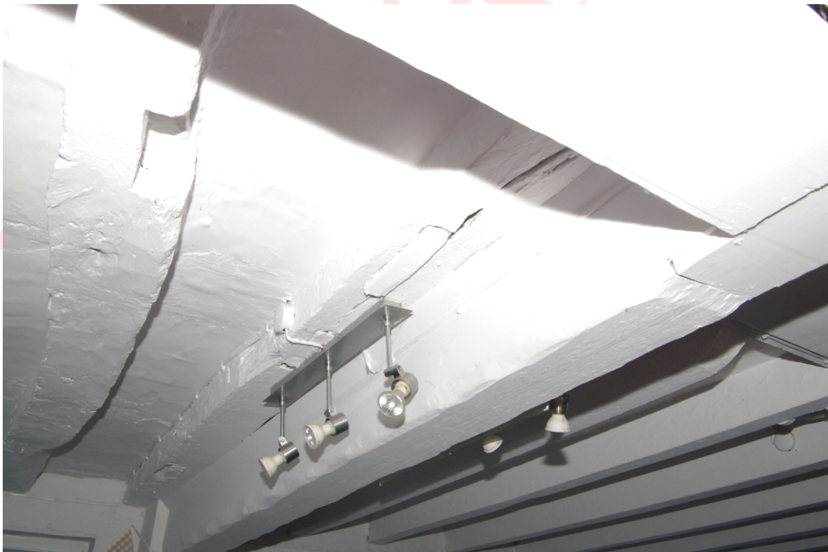
Figure 43: Room G1, reused timbers as ceiling joists
