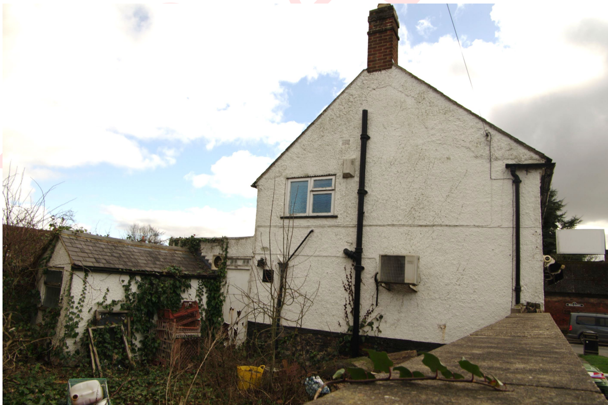
Figure 32: North-west facing elevation Looking south-east. Note the small extension on the left
