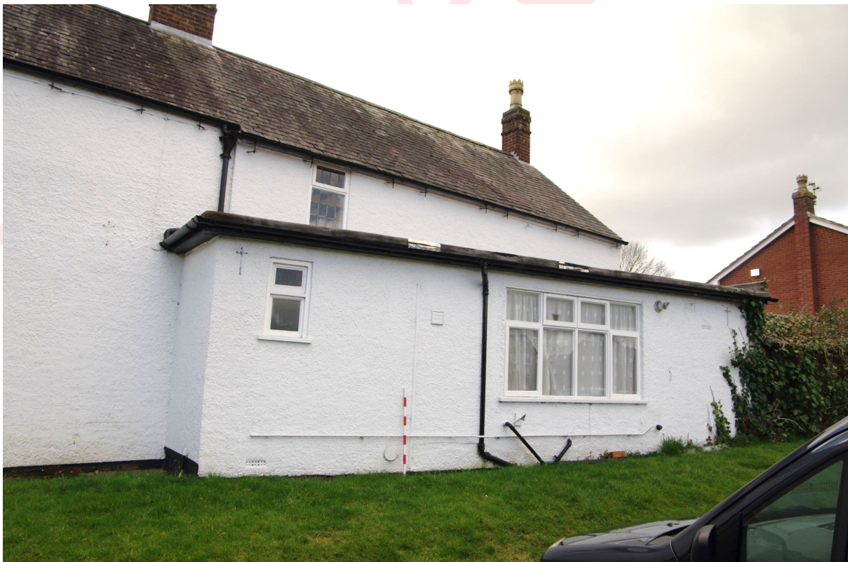
Figure 29: NE facing elevation, flat-roofed extension Looking north-west. Note the step in wall and eaves line to the right of the first floor downpipe. 1m scale
