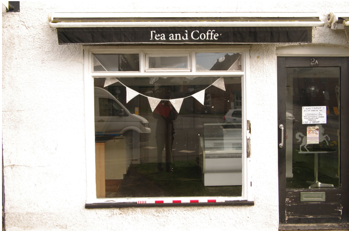
Figure 12: SW facing elevation, No 2A, ground floor window and door detail Looking north-east. 1m scale. Note the Lloyds Bank logo on the door
