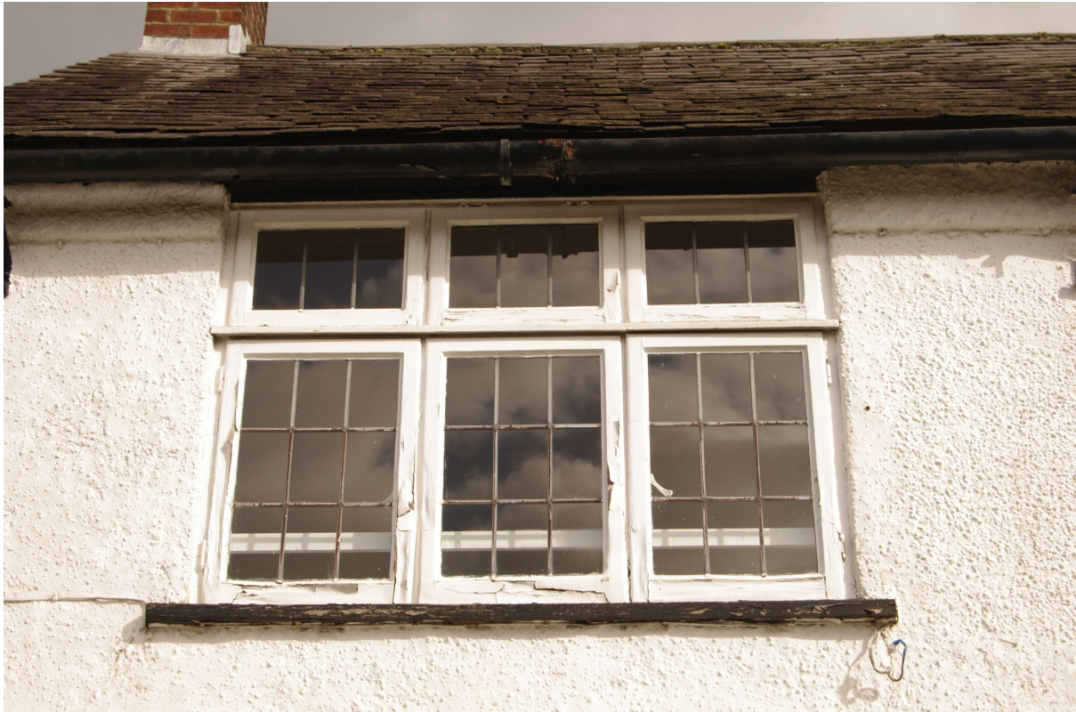
Figure 14: SW facing elevation, first floor window detail above 2A (left window) Looking north-east
