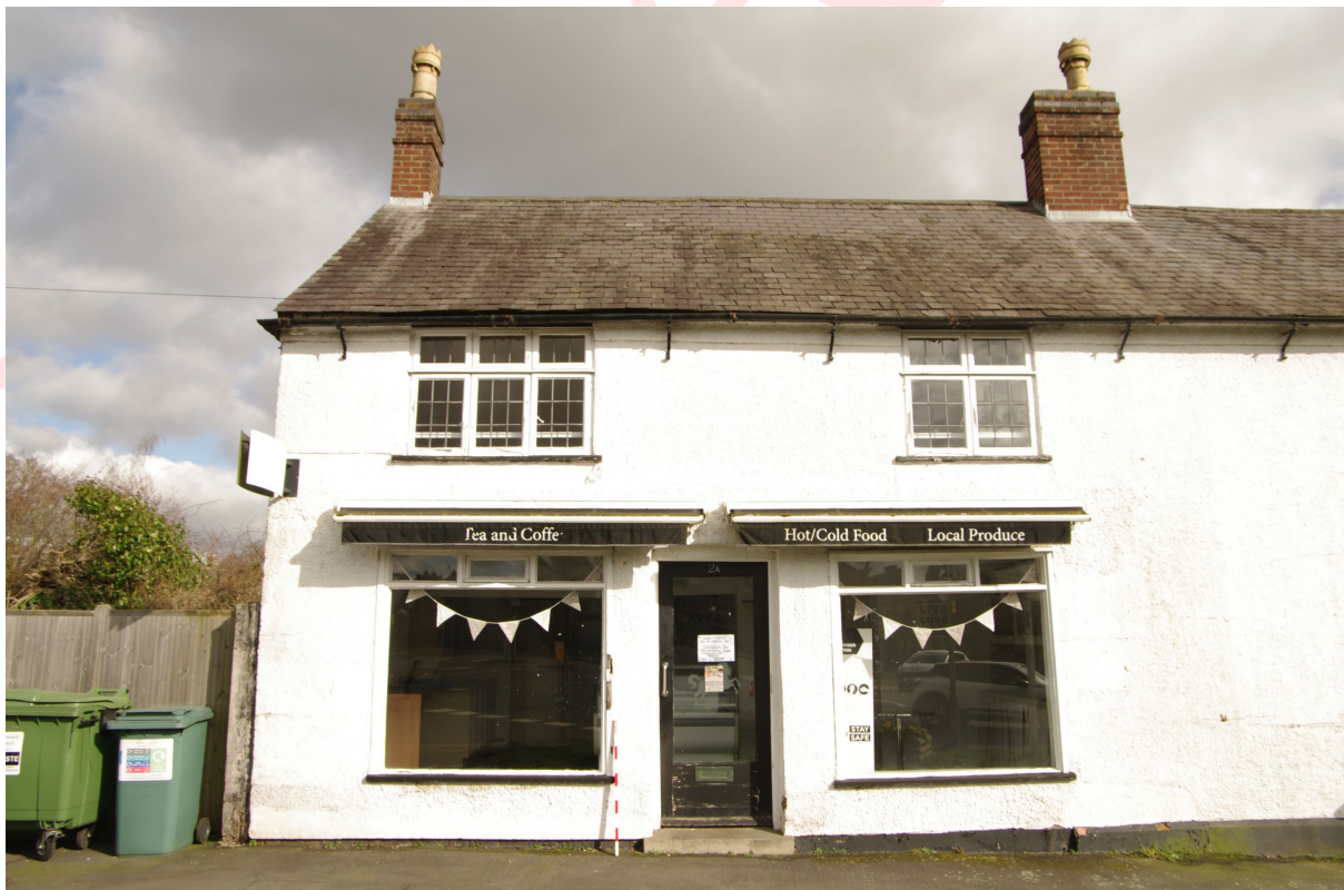
Figure 11: SW facing elevation, Number 2A Main Street
