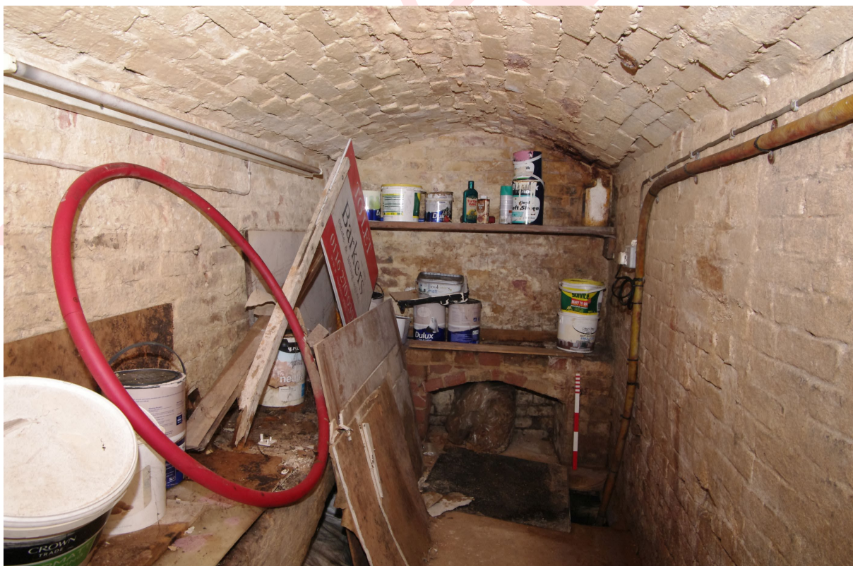
Figure 35: Cellar, general view Looking north-west. 0.5m scale
