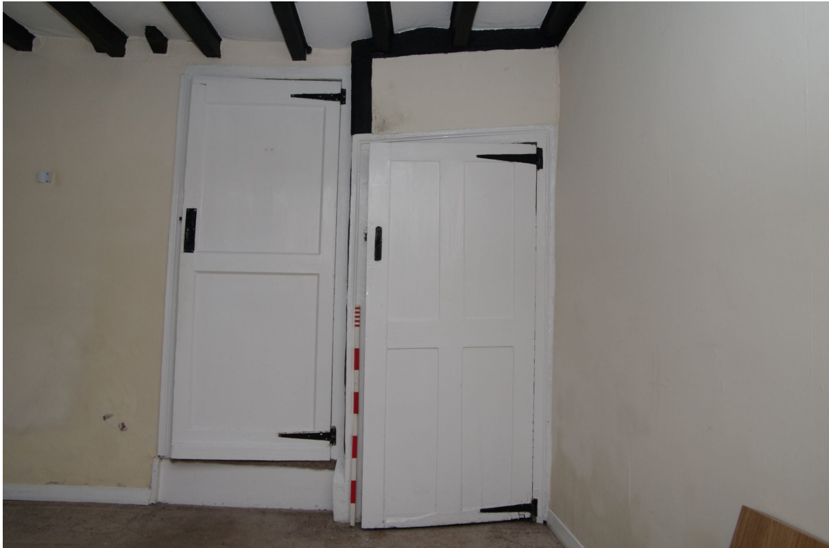
Figure 49: Room G4, doors to first floor stairs and cellar Same view as previous picture but with doors closed. 1m scale
