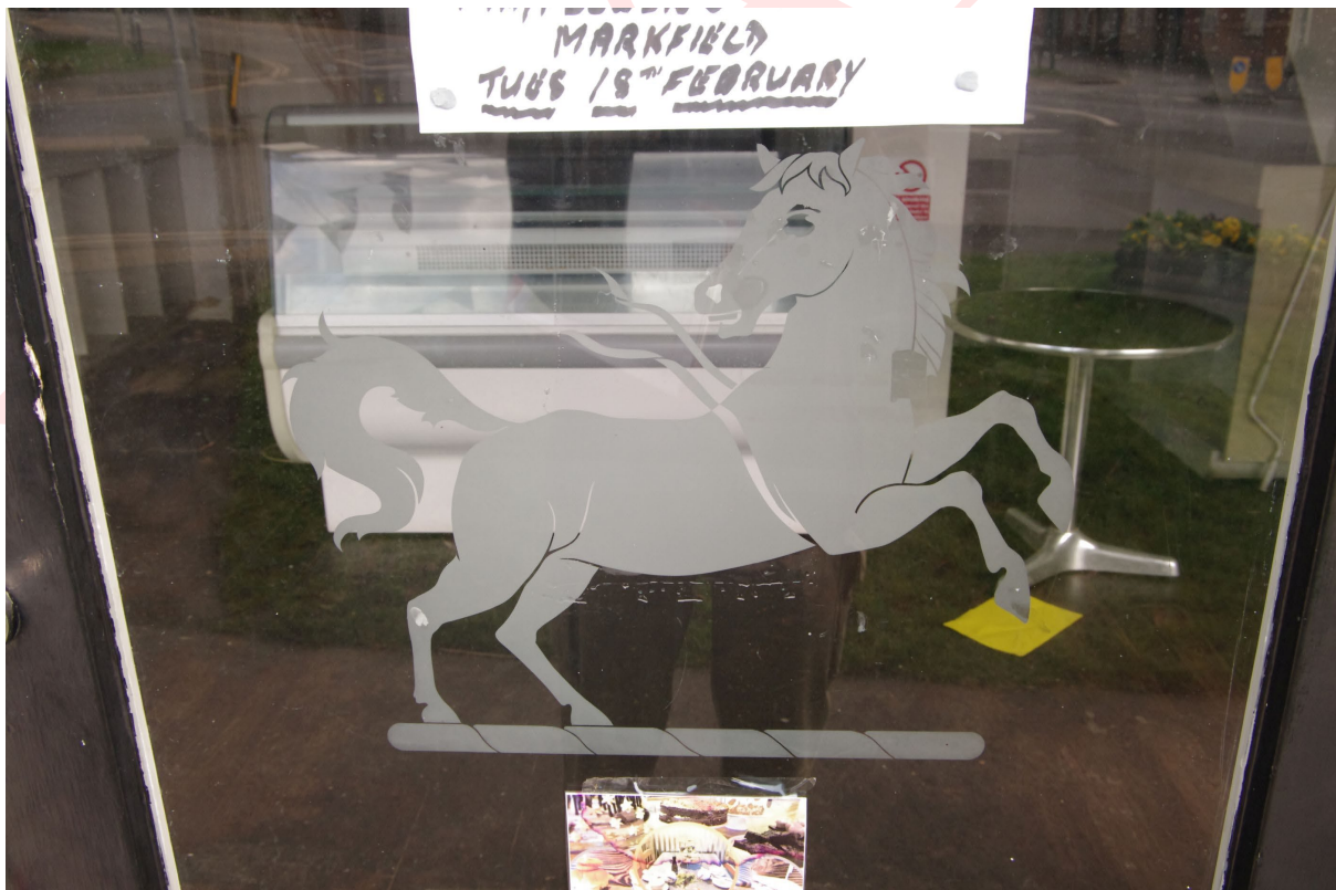
Figure 13: SW facing elevation, No 2A, ground floor door logo detail Looking north-east
