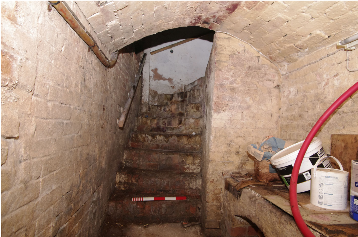
Figure 36: Cellar steps Looking south-east. Note brick-arched thrall on the right. 0.5m scale
