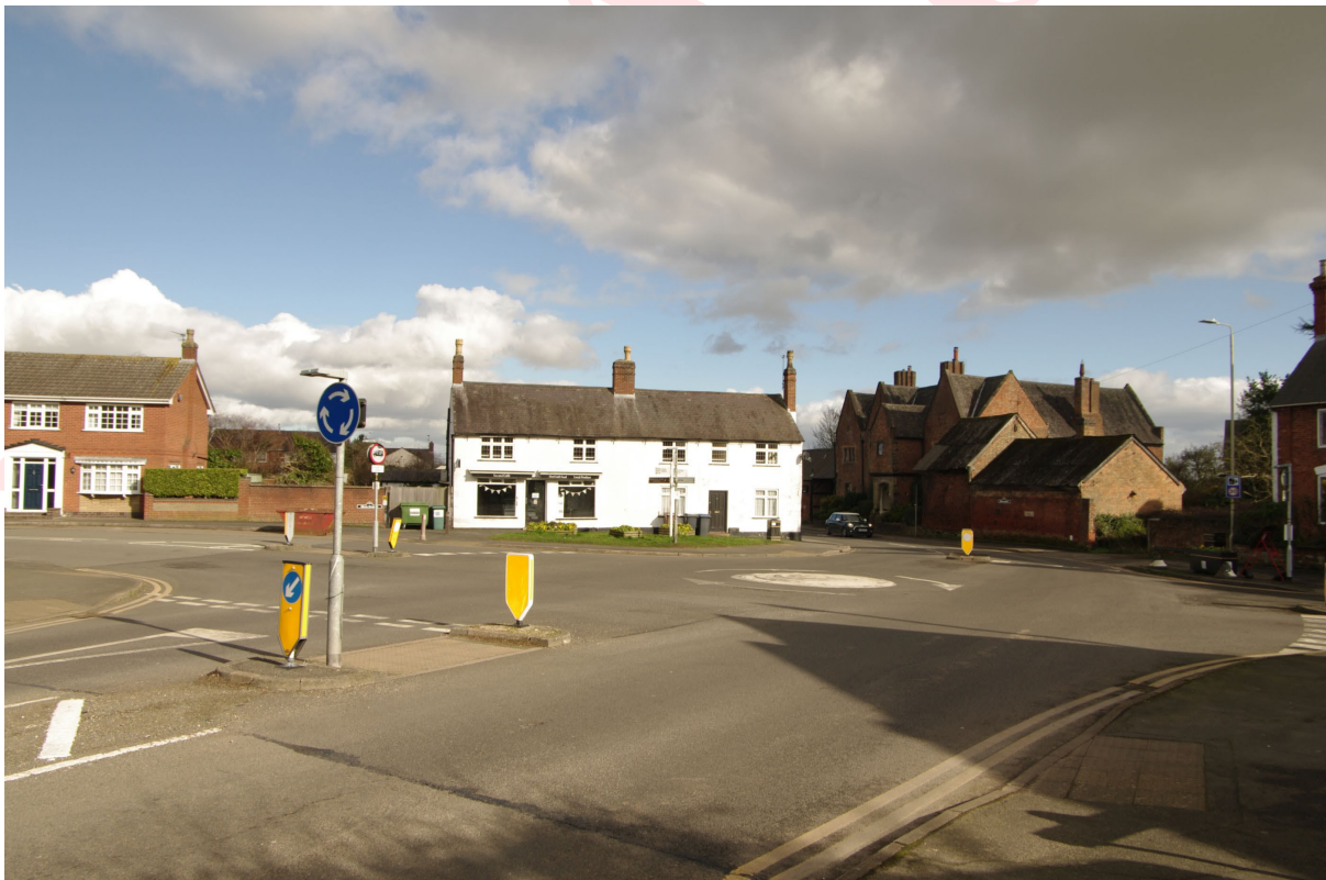
Figure 5: View of the surveyed building seen from Manor Road
