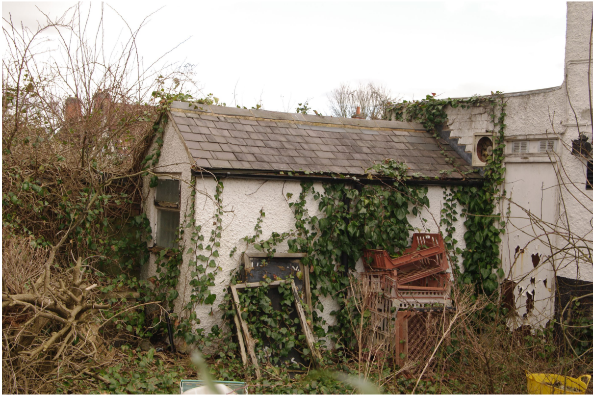
Figure 22: SW facing elevation of the extension on the NW side of the building Looking south-east. Note how it joins with the flat-roofed rear extension
