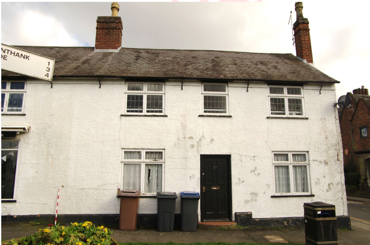
Figure 17: SW facing elevation of Number 37 High Street Looking north-east. 1m scale. High Street can be seen on the right
