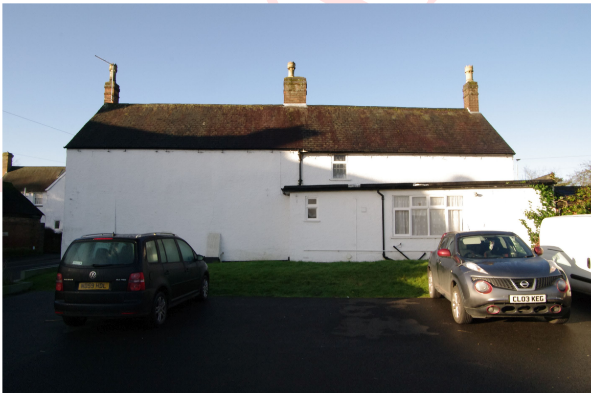
Figure 27: North-east facing elevation Looking south-west. Note the single storey extension to the right and lack of window and door openings on this elevation
