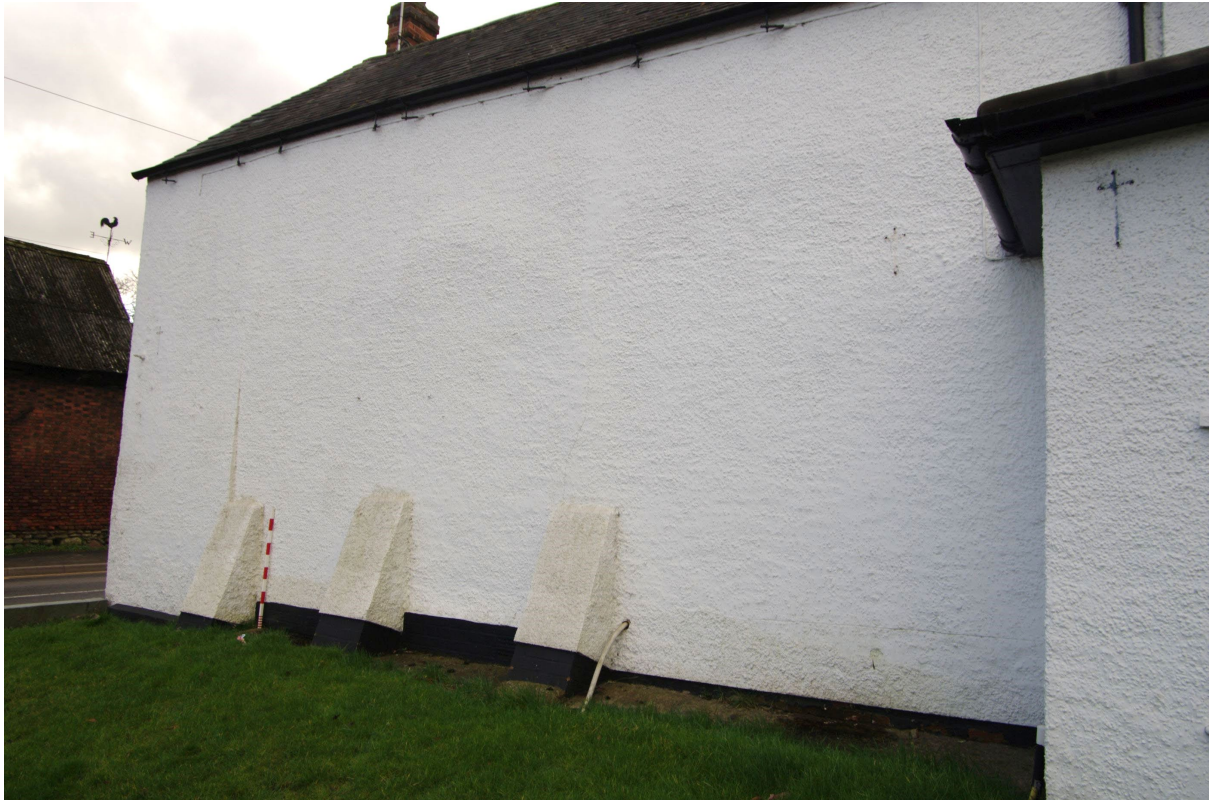
Figure 28: NE facing elevation, southern end with step in the wall line Looking south. The step can be seen as a line just beyond the left hand buttress. 1m scale
