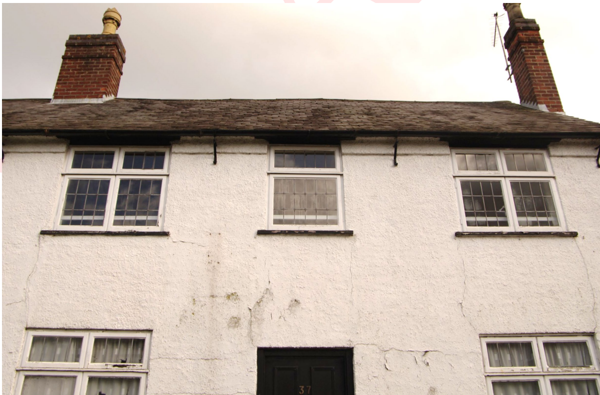
Figure 21: SW facing elevation of No 37, first floor window detail Looking north-east. As with No 2A these first floor windows have leaded panes
