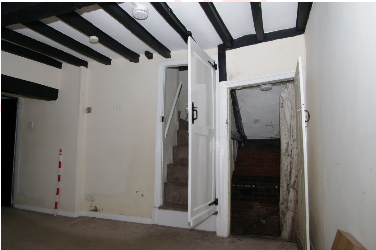
Figure 48: Room G4, doors to first floor stairs and cellar Looking north-east. Note the change in wall thickness to the right of the 1m scale
