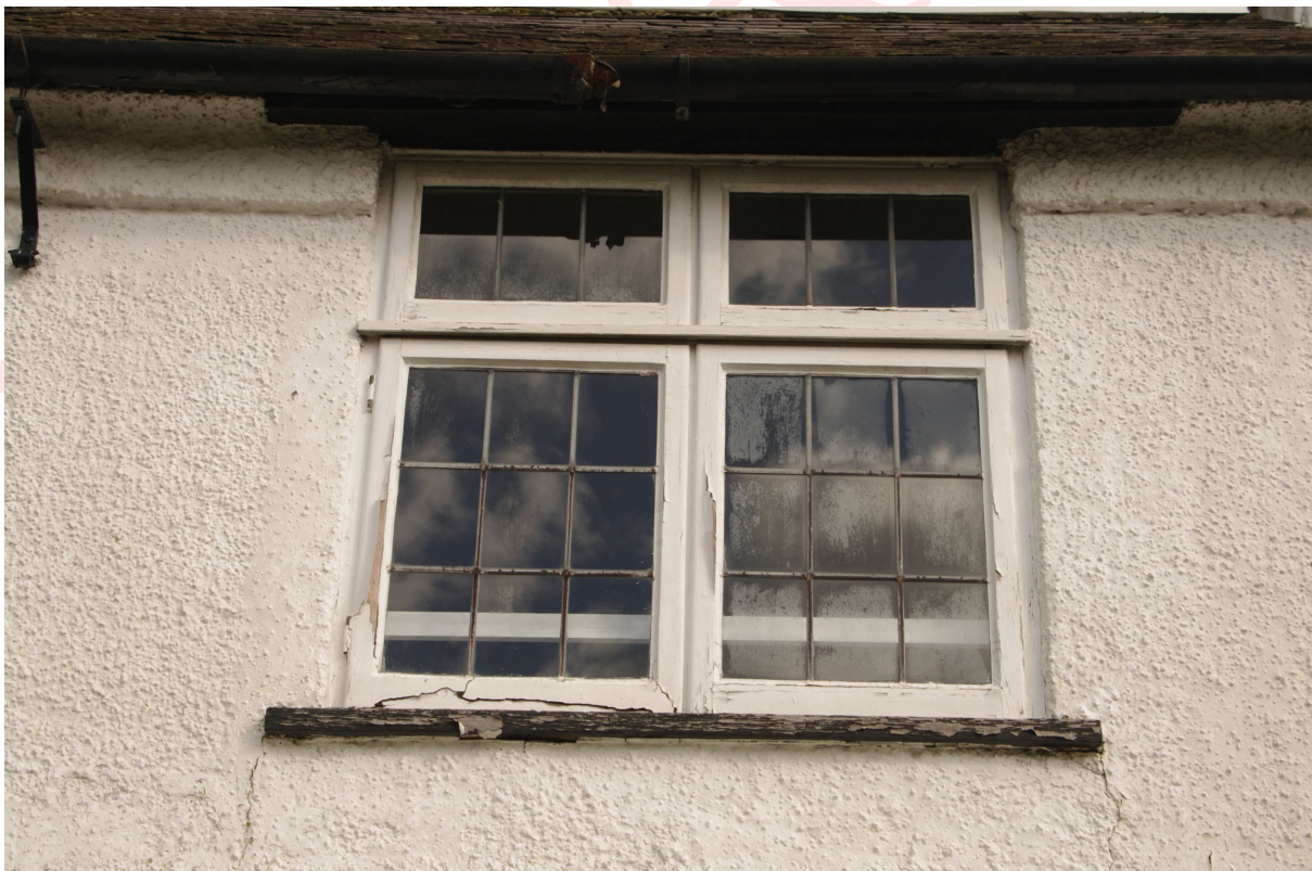
Figure 15: SW facing elevation, first floor window detail above 2A (right window) Looking north-east
