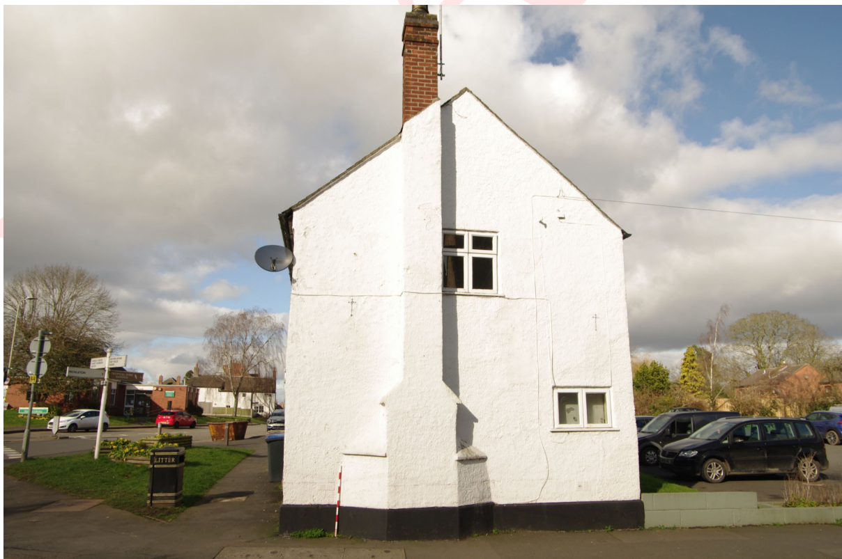
Figure 24: South-east facing elevation of 37 High Street
