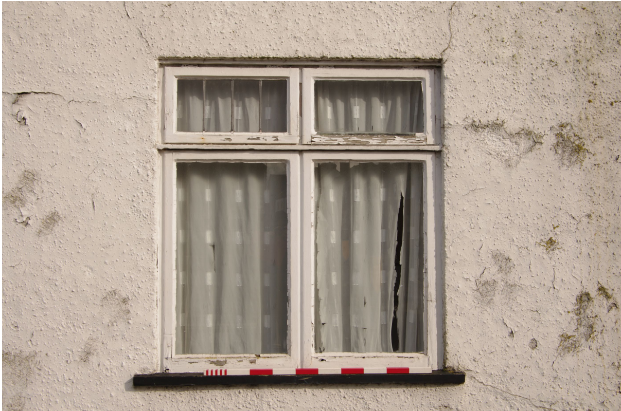
Figure 20: SW facing elevation of No 37, ground floor window detail to right of door Looking north-east. 1m scale
