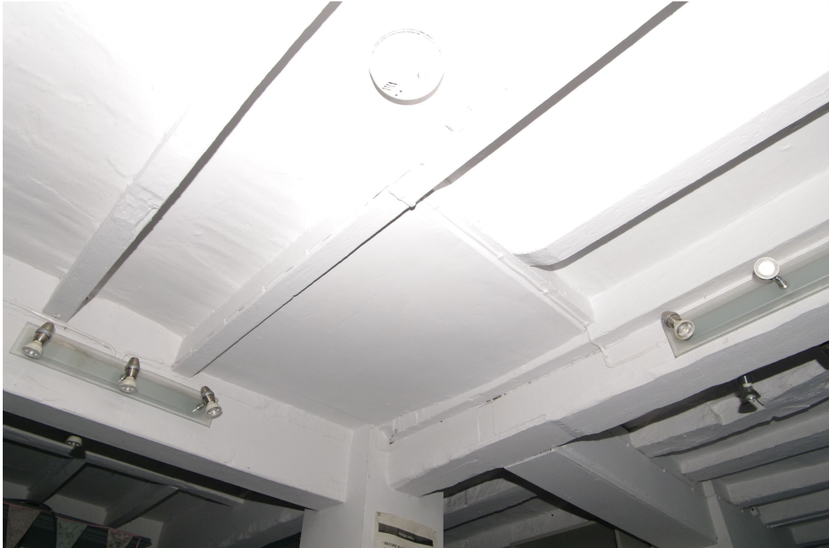
Figure 44: Room G1, location of former staircase up to first floor Looking east
