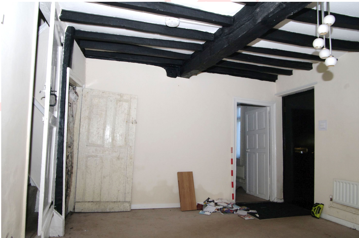
Figure 50: Room G4, southern wall Looking south. Doorway to Room G5 to right of 1m scale. Front door on far right. Stairs and cellar doors are on the left
