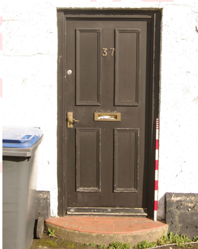
Figure 19: SW facing elevation of No 37, door detail Looking north-east. 1m scale
