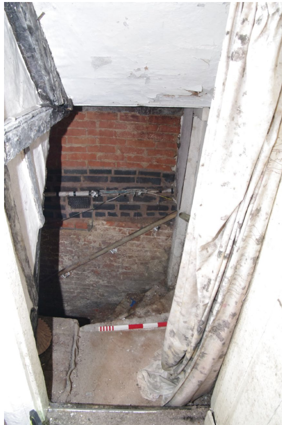
Figure 34: Cellar steps seen from ground floor Room G4 Looking north-east. 0.5m scale
