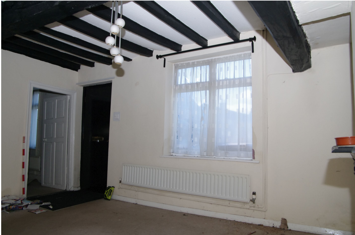
Figure 51: Room G4, western wall Looking south-west. 1m scale
