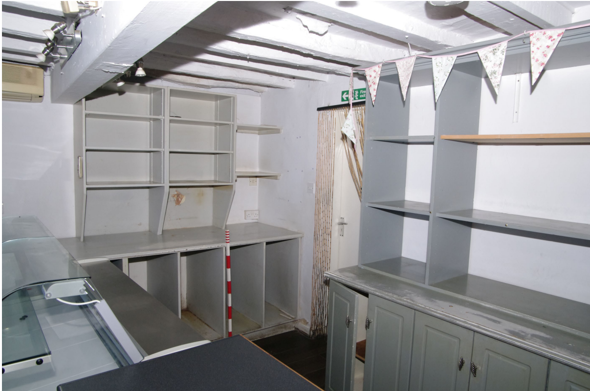
Figure 42: Rear of Room G1
