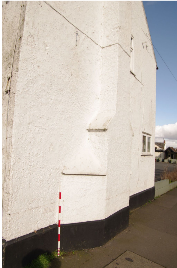
Figure 25: SE facing elevation chimney breast detail Looking north. 1m scale
