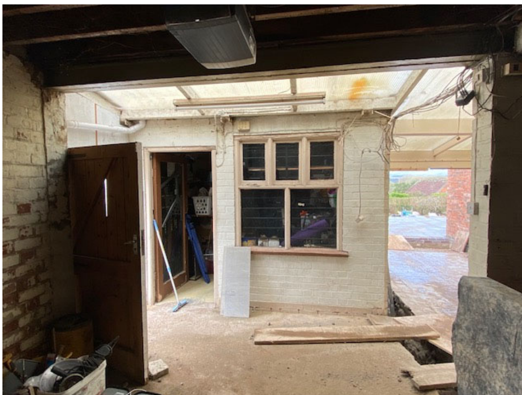
Fig 8. No. 44 Newbold Road – Internal view of Workshop and Garage
