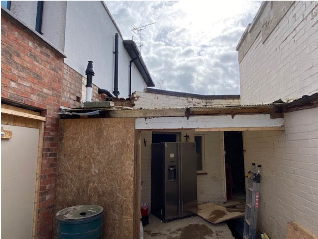
Fig 4. No. 44 Newbold Road – Link between house and Workshop and Garage
