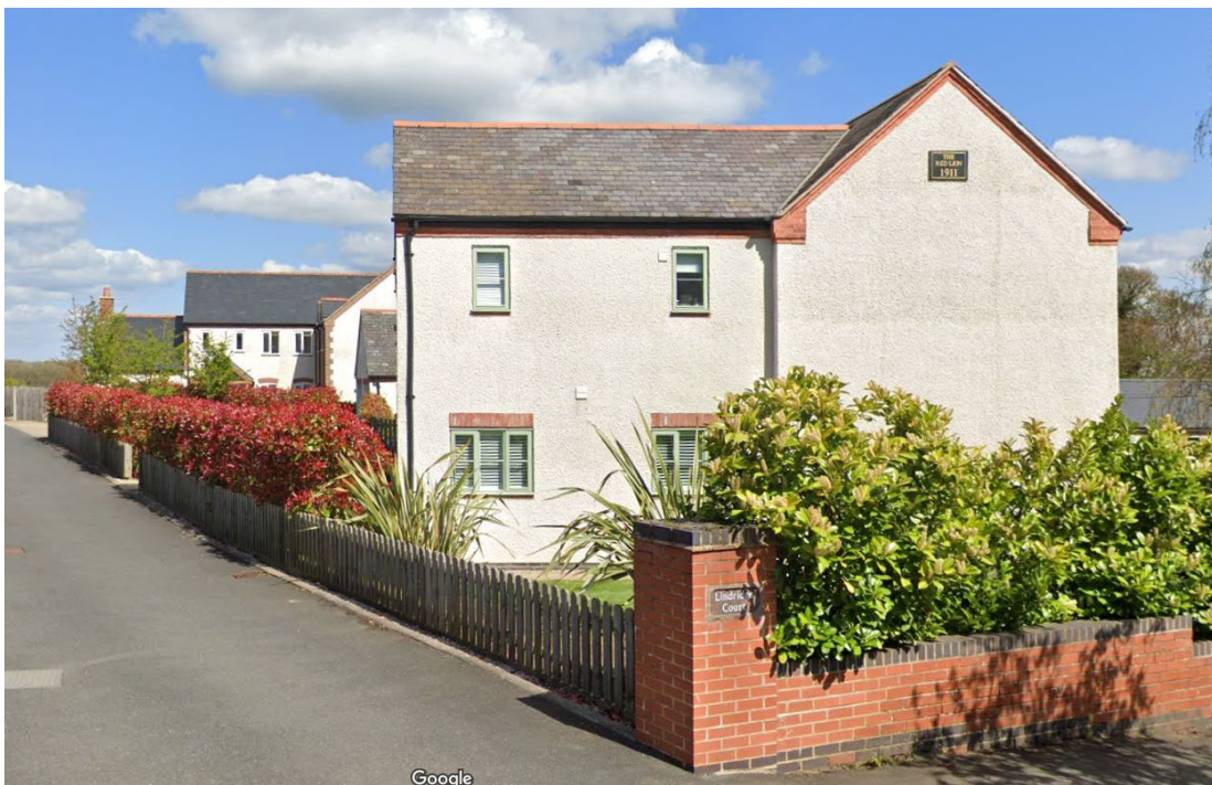
Fig 17. Brick features with render detached dwelling on Newbold Road (Infill development)
