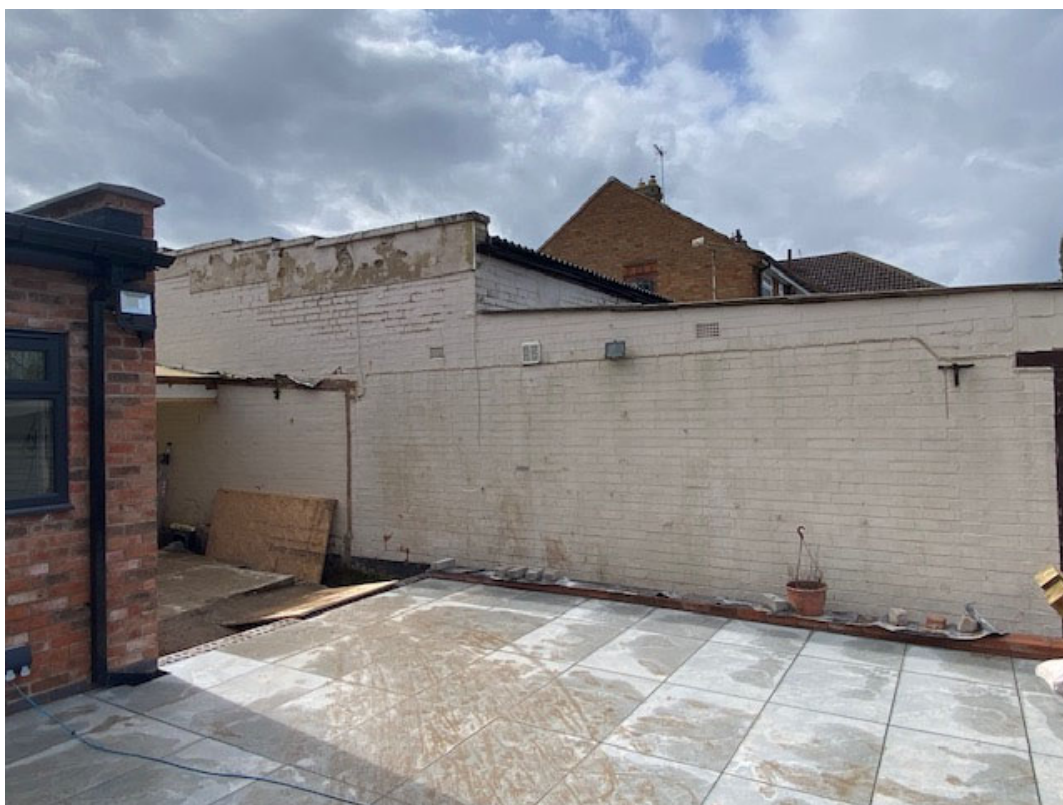
Fig 6. No. 44 Newbold Road – Side elevation of Workshop and Garage
