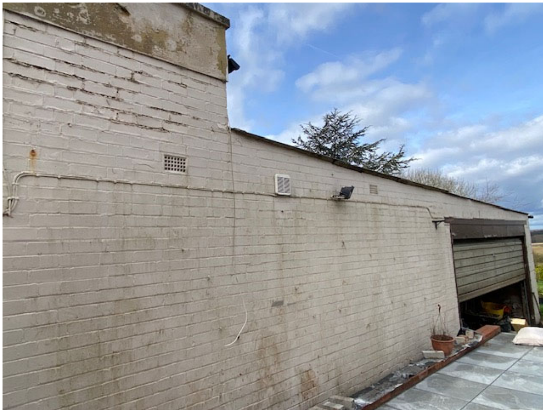
Fig 5. No. 44 Newbold Road – Side elevation of Workshop and Garage
