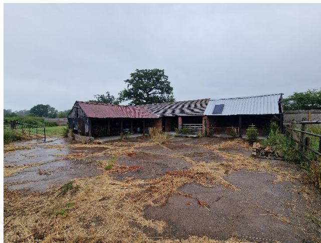
Photo 2: Sealed surface and building on site.
