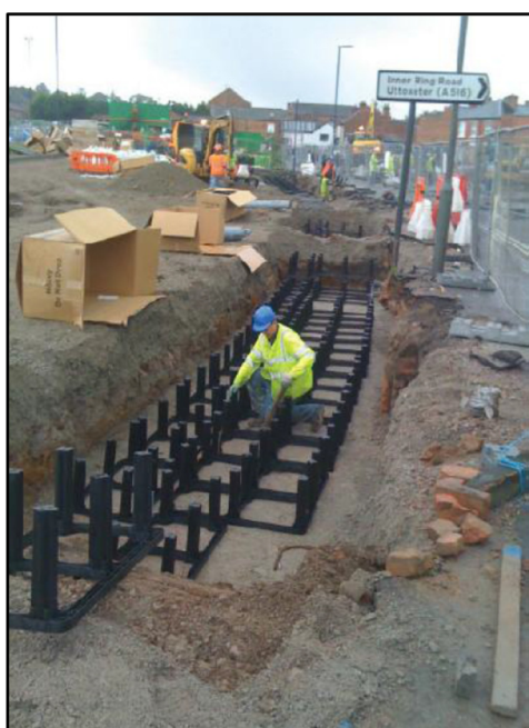
(Top) Fig. 5.1 Silva Cell TM design specification. (L) Fig. 5.2 Silva Cell TM Installation (R) Fig. 5.3 Completion. All images © Deep Root Ltd.
