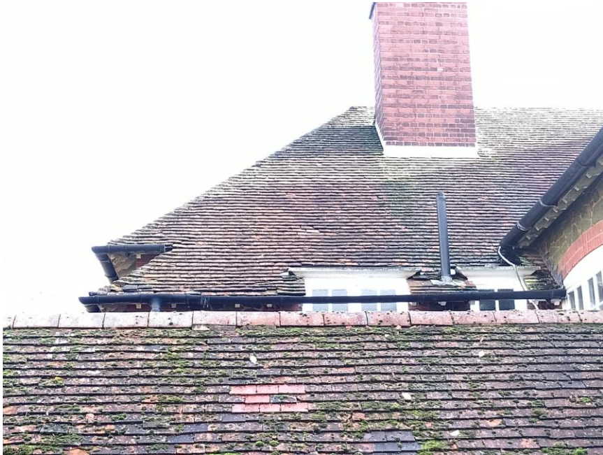
Img.5. North elevation with dropped 2 story tile section PRF's.
