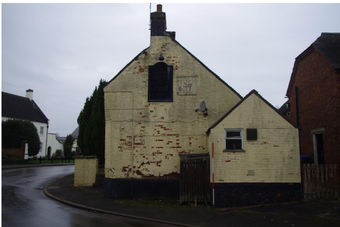
Figure 9 Building A , East – North East Facing Gable (Looking West – South West).
