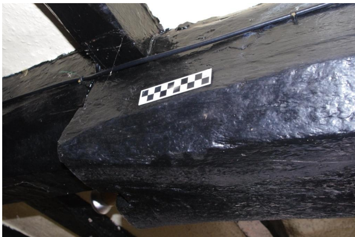
Figure 13 A(3) , Chamfered & Stopped Bridging Beam (Looking South East).
