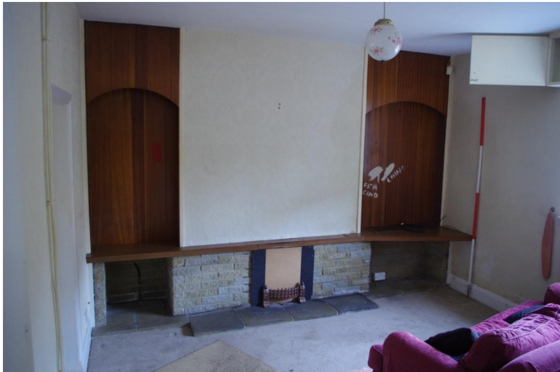
Figure 22 A (5), General View (Looking East).
