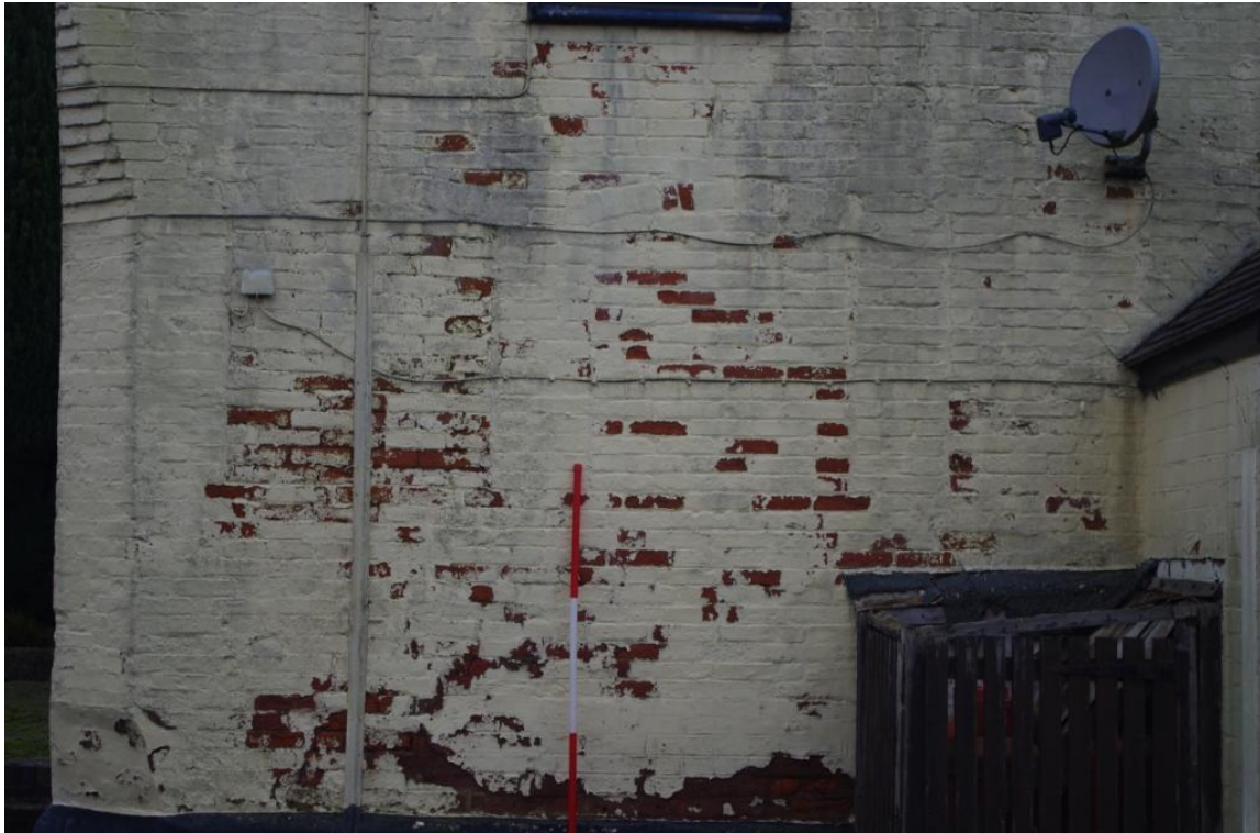
Figure 10 Building A , East – North East Facing Gable, Showing Blocked Openings (Looking West – South West).
