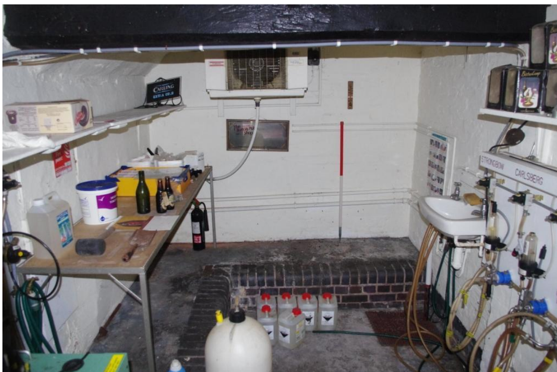
Figure 14 A (4), Barrel Store (Looking East – North East).
