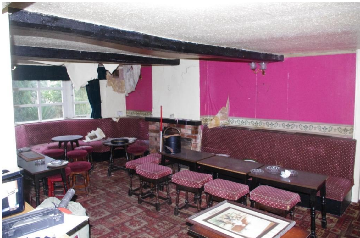
Figure 23 A (2), General View (Looking South West).
