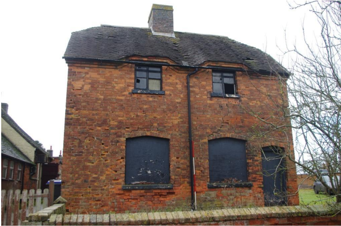
Figure 16 Building B, Principal Elevation (Looking West).
