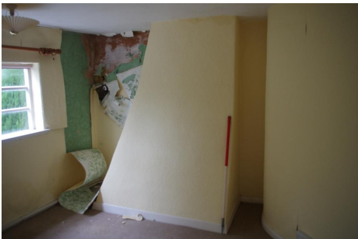
Figure 15 A (9), Chimney Breast (Looking West – South West).
