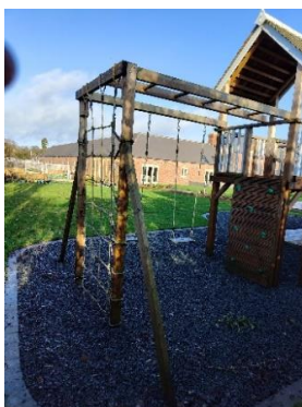
PLAYHOUSE & CLIMBING FRAME WITH SEMI POROUS SOFT PLAYSURFACING
