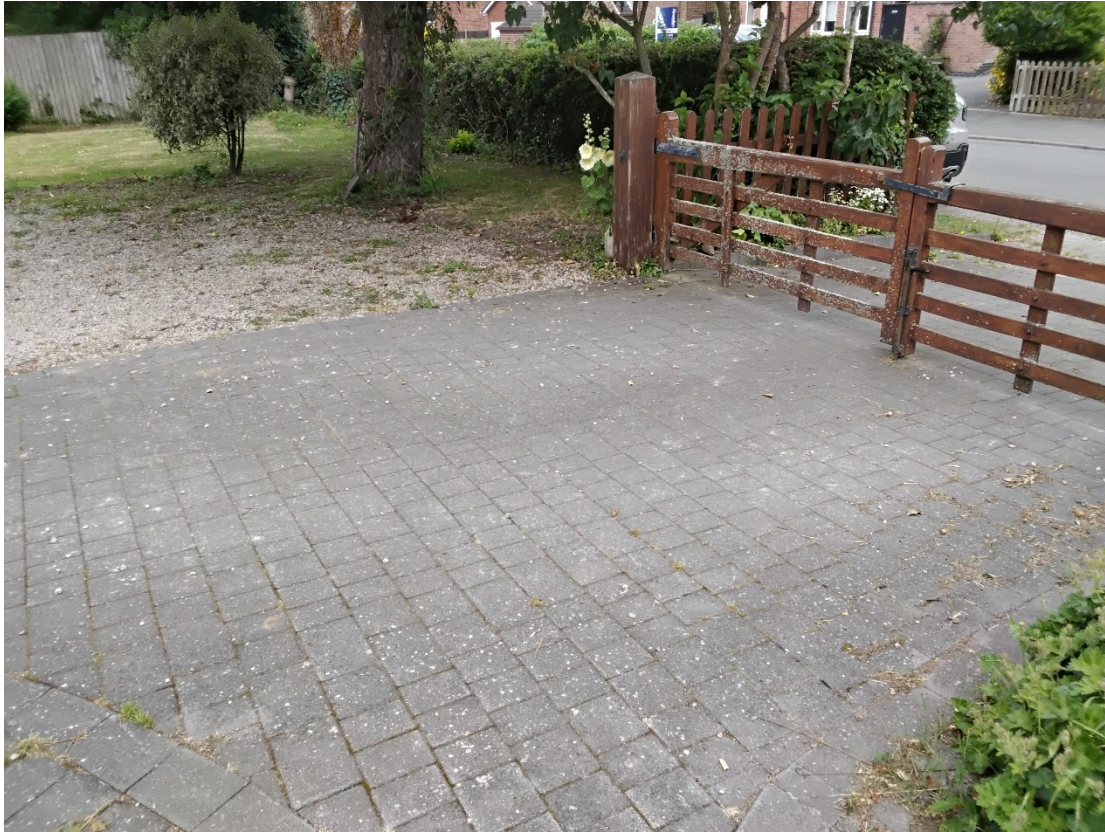
Figure 3 Sealed surface brick driveway in the northeast of the Site (facing southwest)
