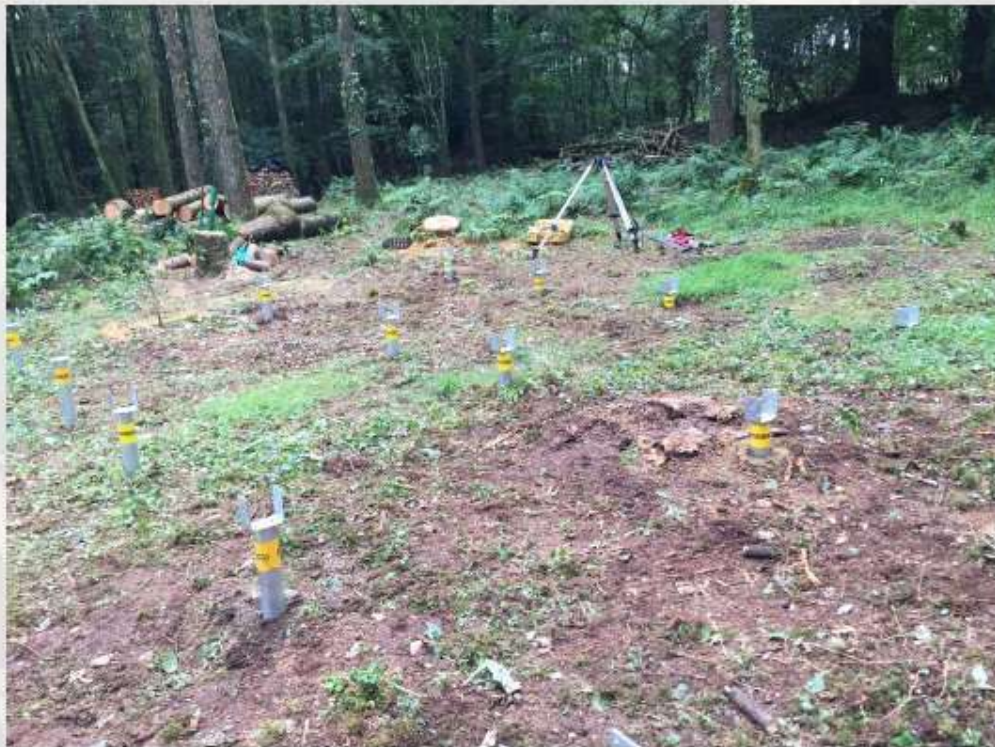
Screws installed ready for base frame
