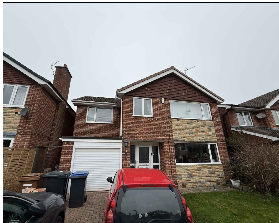
Site Photograph As Existing
