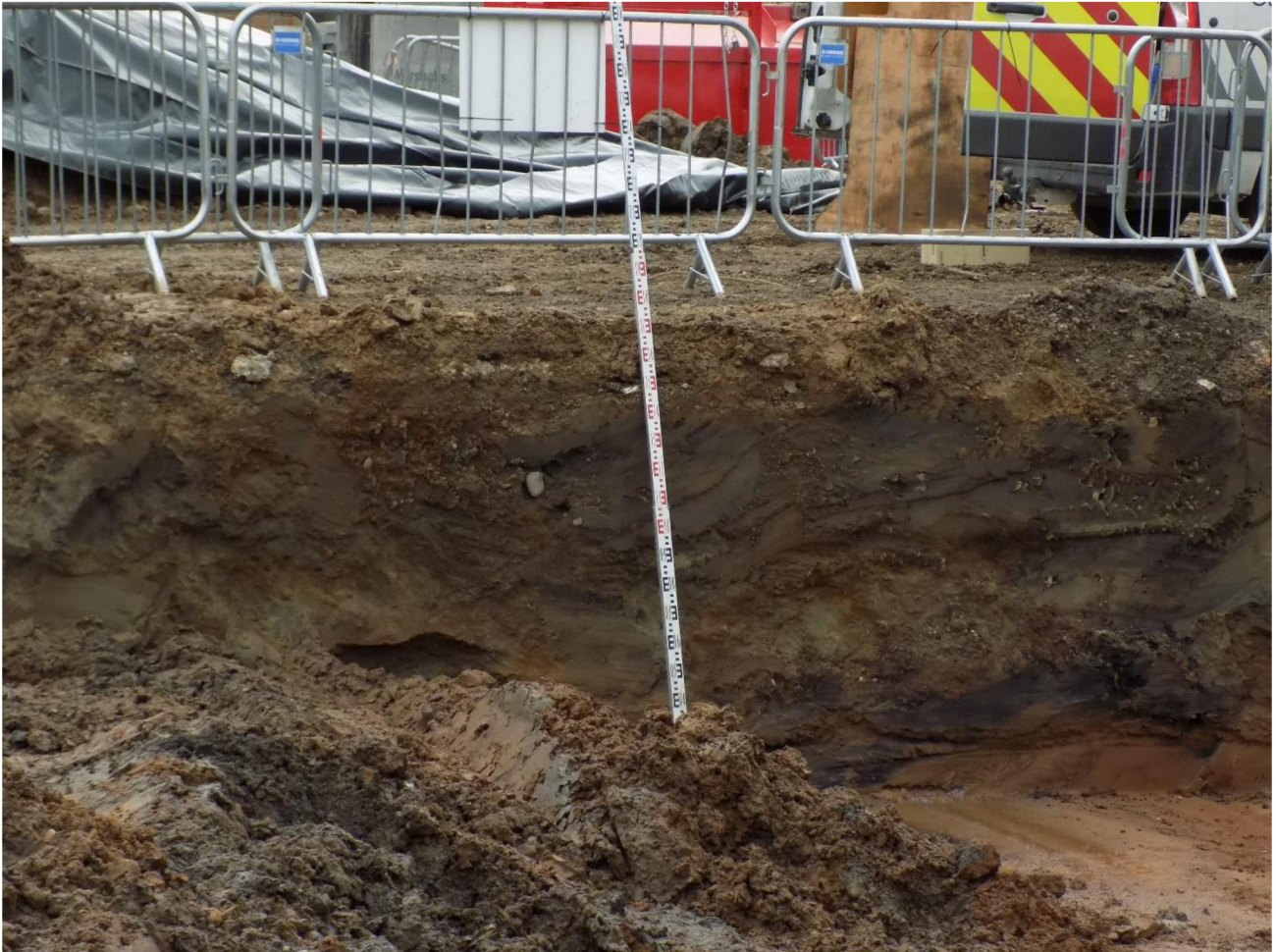
Figure 5: Photograph of Trial Pit Area
