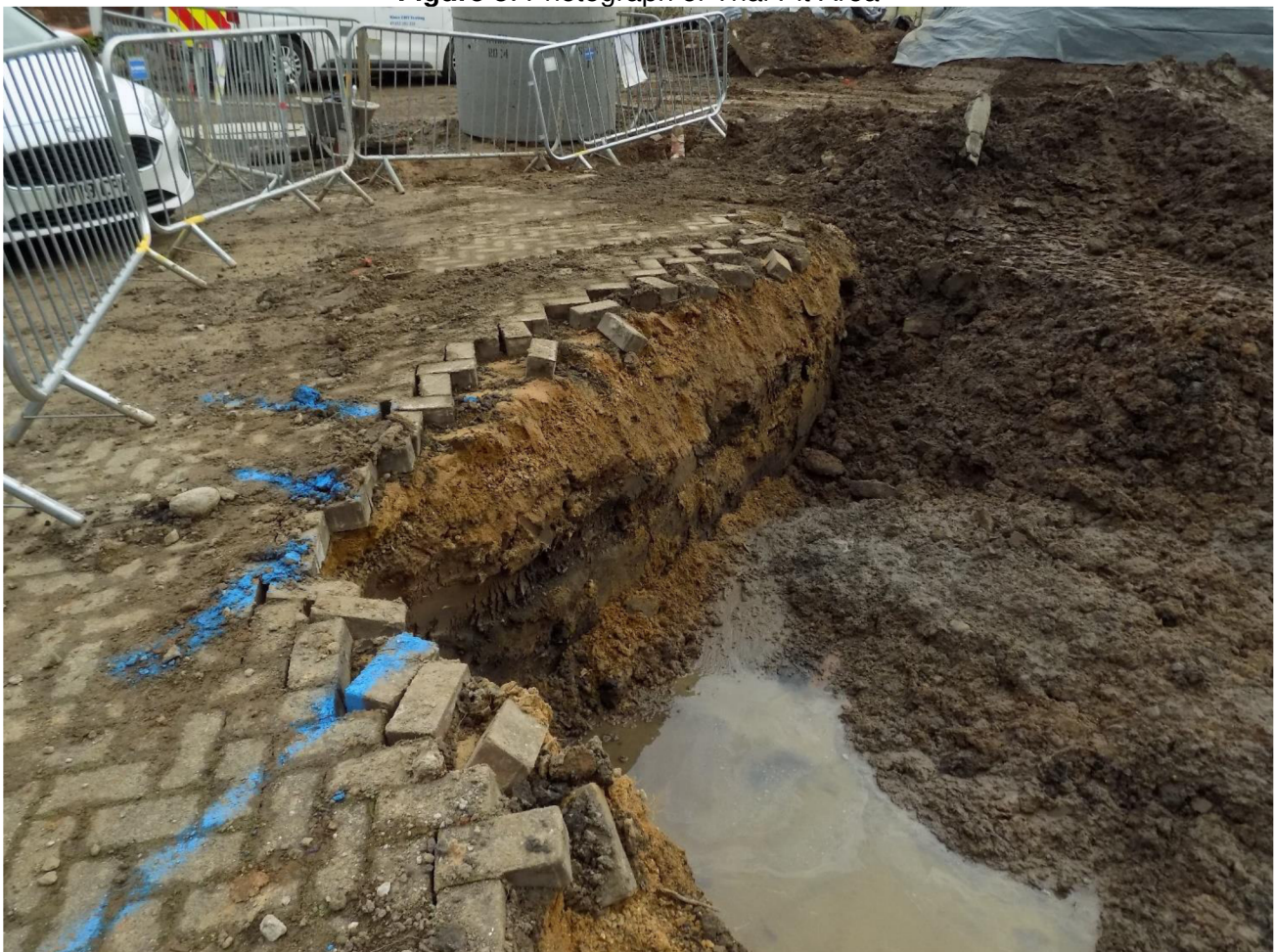
Figure 6: Photograph of Trial Pit Area
