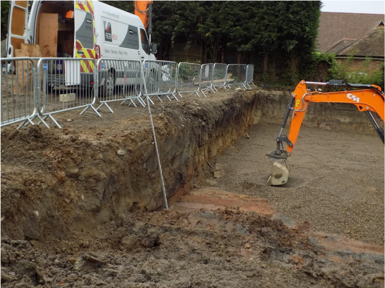
Figure 6: Photograph of Trial Pit Area
