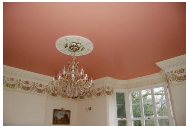
Figure 23: Ph (28). Plasterwork to room 2
