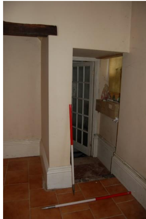
Figure 39: Ph (60). Room 9 facing west
