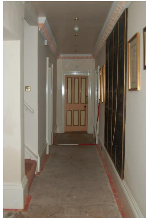
Figure 33: Ph (51). Room 6 facing east
