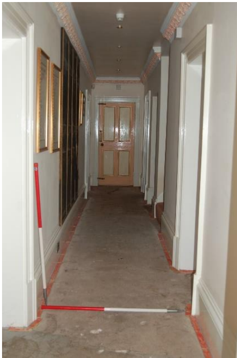
Figure 32: Ph (50). Room 6 facing west
