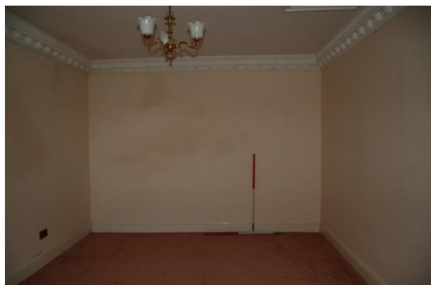
Figure 64: Ph (92). Room 20 facing north
