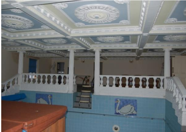
Figure 42: Ph (65). Room 11 facing north
