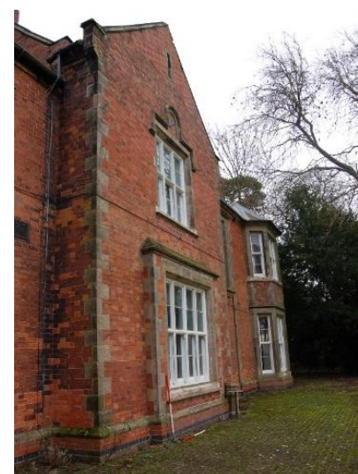
Figure 12: Ph (8). East end of the south elevation
