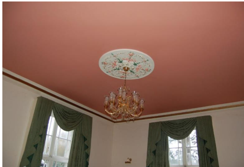
Figure 19: Ph (22). Ceiling rose to room 1
