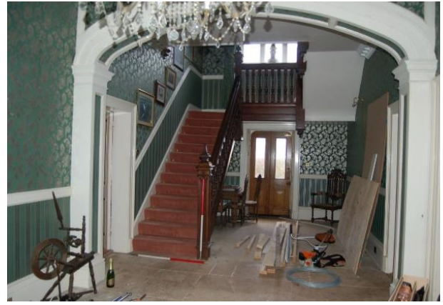
Figure 25: Ph (31). Room 3 facing north
