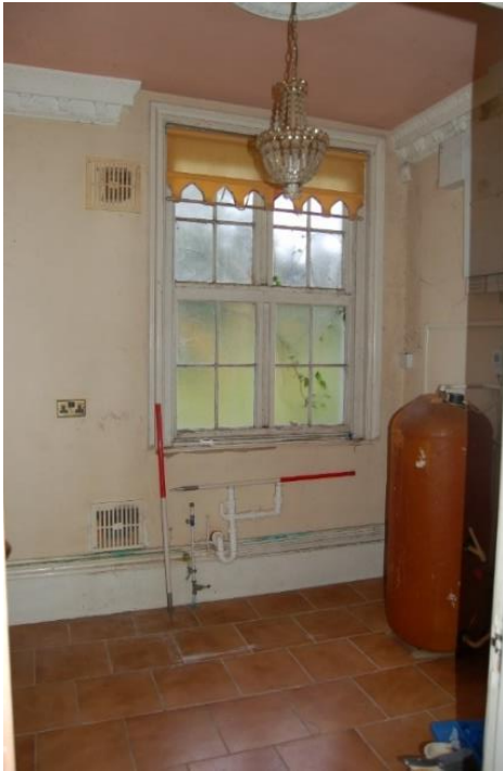
Figure 38: Ph (59). Room 9 facing north
