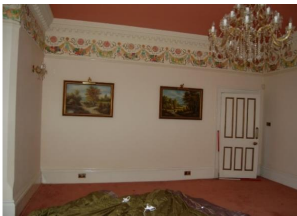
Figure 22: Ph (27). Room 2 facing west
