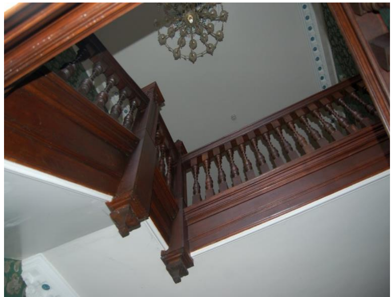
Figure 27: Ph (35). Stair and landing to room 3
