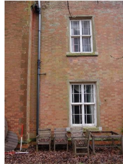
Figure 10: Ph (14). Windows to the east elevation
