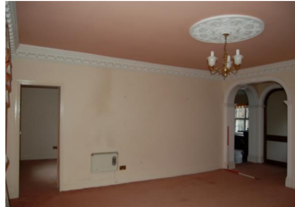
Figure 62: Ph (89). Room 19 facing west
