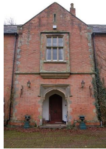
Figure 6: Ph (19). Detail of door to north elevation
