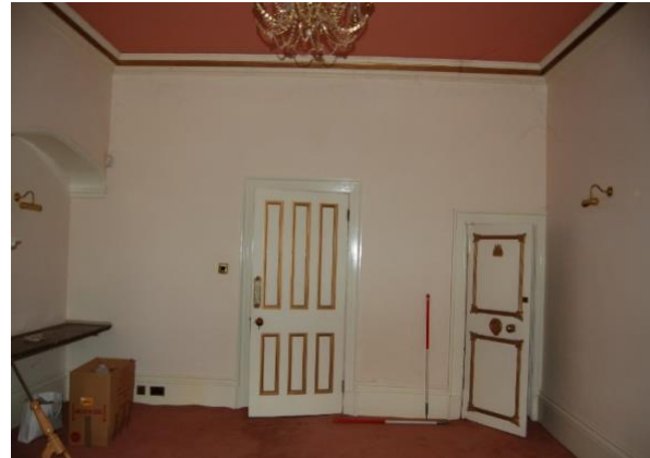
Figure 17: Ph (23). Room 1 facing west
