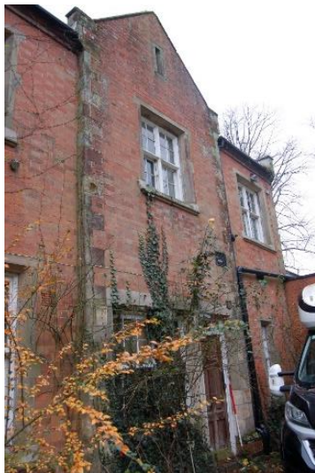
Figure 7: Ph (16). West end of the north elevation
