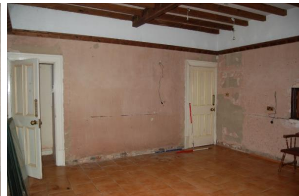
Figure 31: Ph (47). Room 5 facing east
