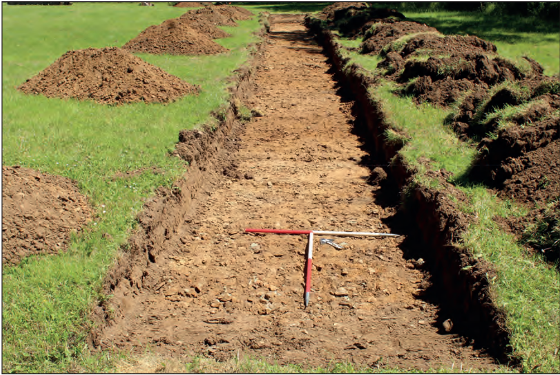
Trench 82, looking north-east (1m scale)
