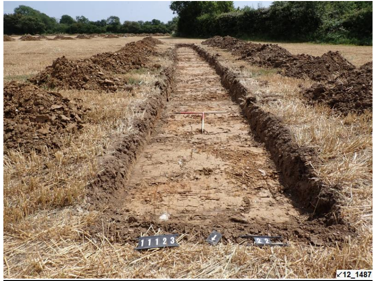
Plate 29: Trench 22 facing south-east, Trench post-strip (scale lengths: 1.0m)
