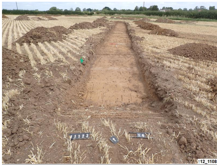
Plate 18: Trench 16 facing north-east, Trench post-strip (scale lengths: 1.0m)
