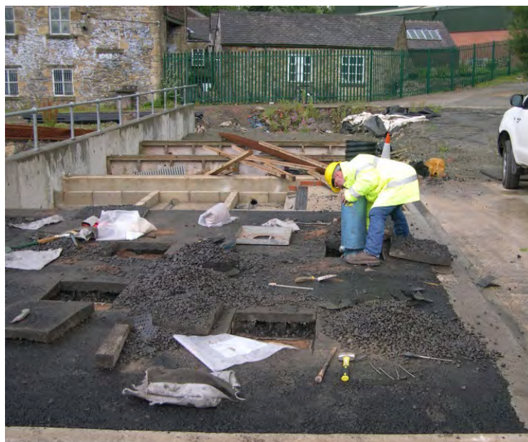
Figure 3 - In situ density tests post-trafficking.
