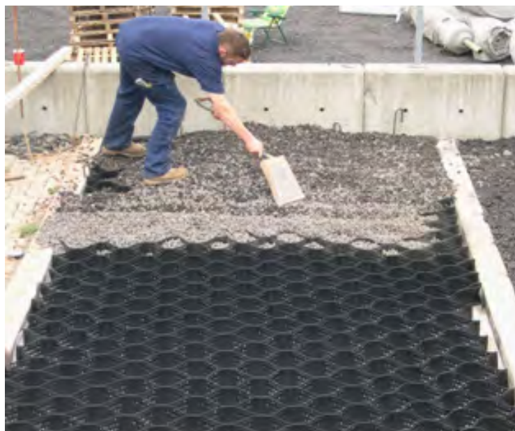
Figure 2 - Cellweb TRP® in construction.
