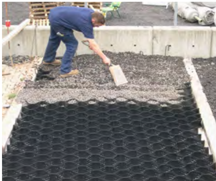
Figure 2 - Cellweb TRP® in construction.
