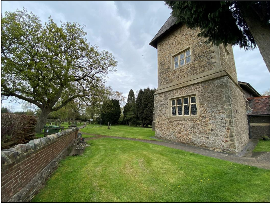
Plate 11: Northeast facing view from Church of St. James (Asset 8) looking towards the Site
