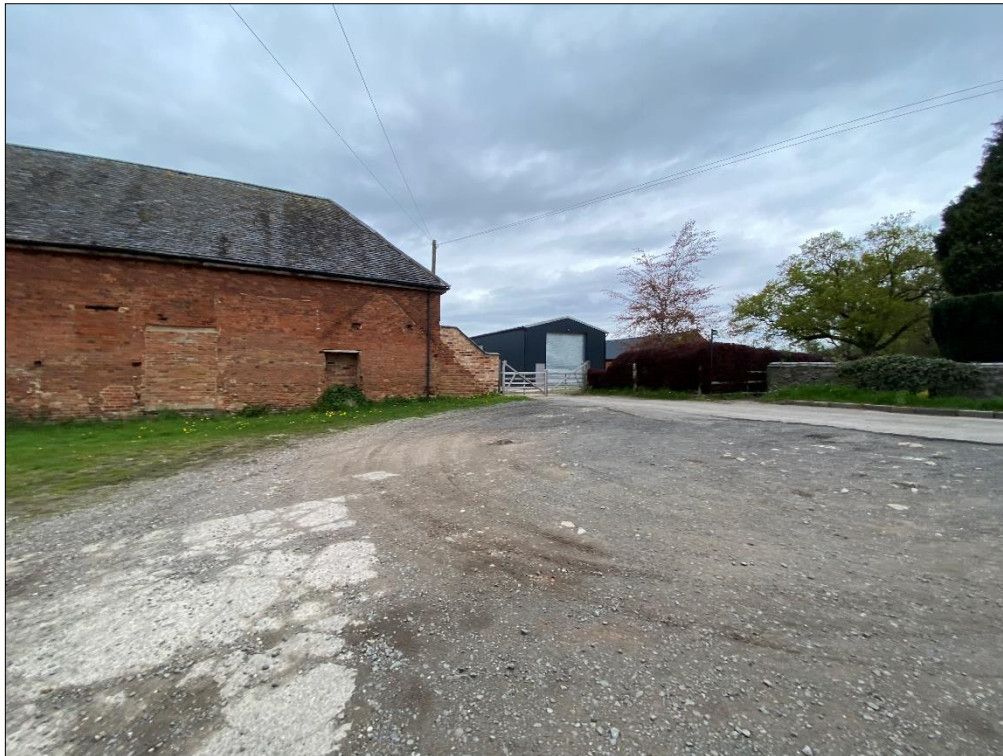
Plate 9: Northwest facing view of Pavilion at southeast Corner of Forecourt at Newbold Verdon Hall (Asset 6)
