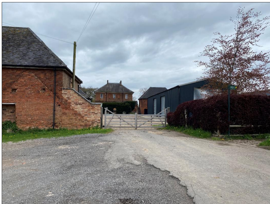
Plate 17: West facing view showing Newbold Verdon Hall (Asset 3) and associated buildings (Assets 6, 11 & 12)
