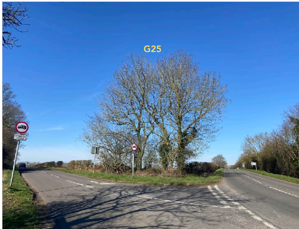
IMAGE 13: The junction of Heath Road (right) with Merrylees Road (Left, looking nwest.
