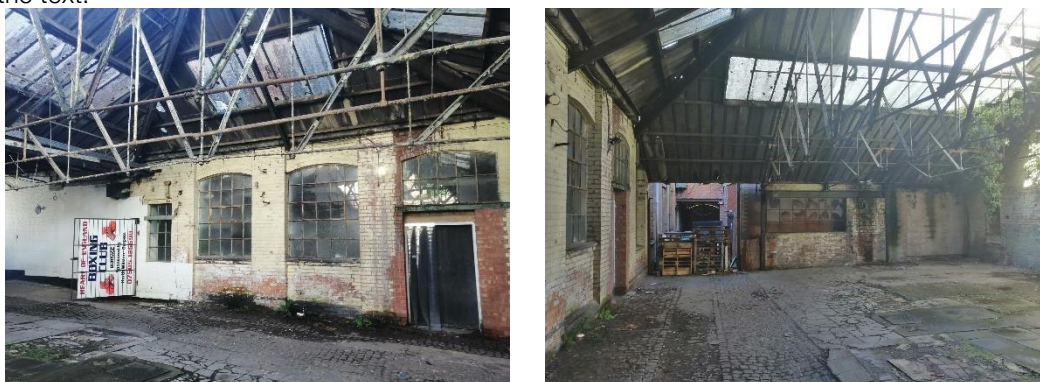
Figure 4 - Existing Boxing Facility 127 Upper Bond St.
