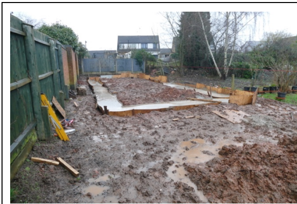
Photo 1: Garden viewed north and concrete footings.
