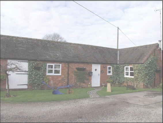
Photo of Existing Front Elevation
