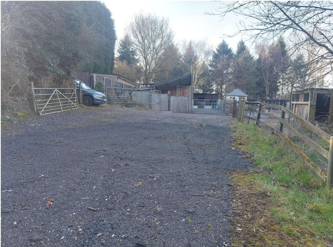
Figure one view of existing stable range and associated hardstanding
