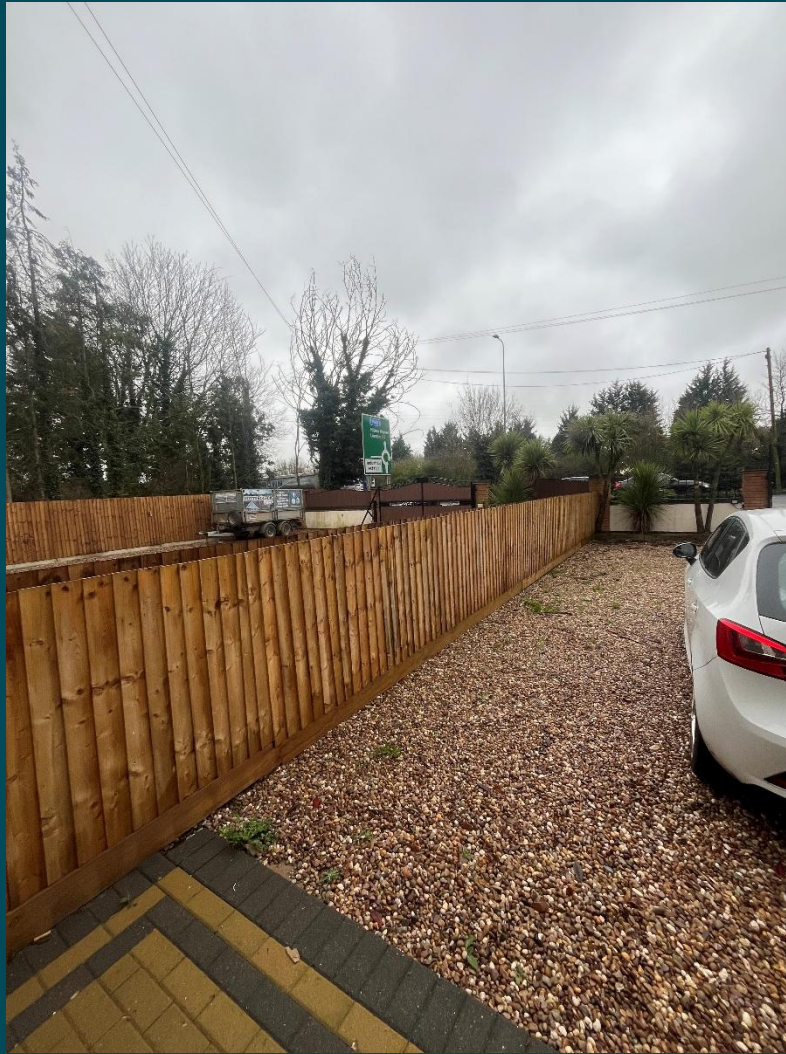
Figure 3: Photograph of Fence
