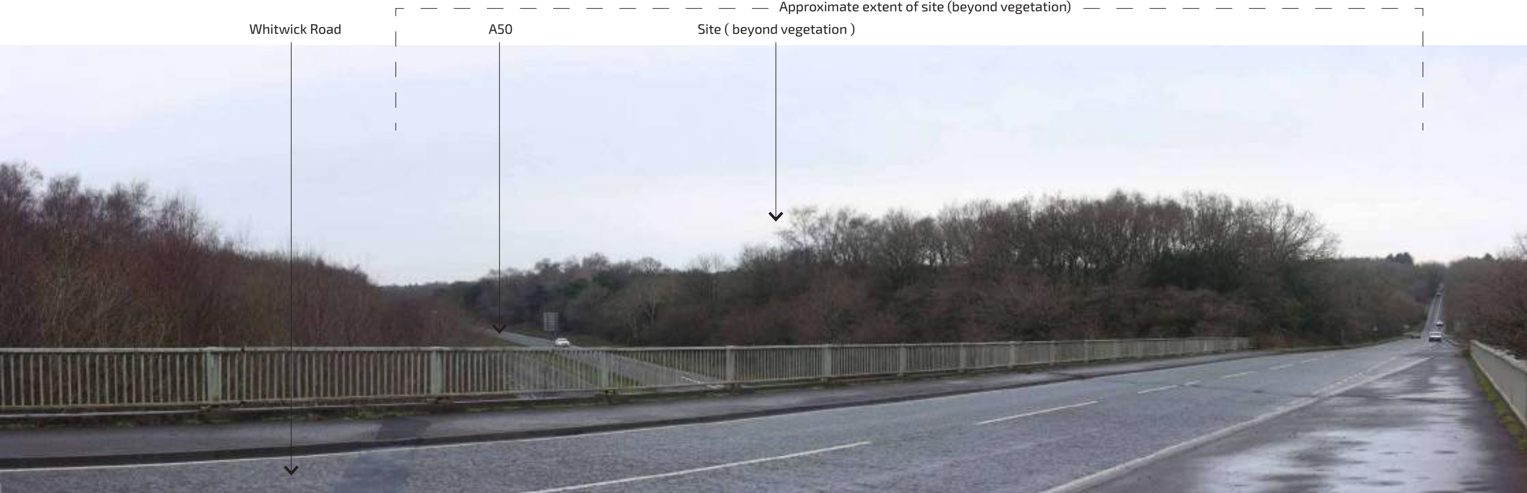
Photo Viewpoint 2f: View north-west from Whitwick Road (A50 overbridge)
