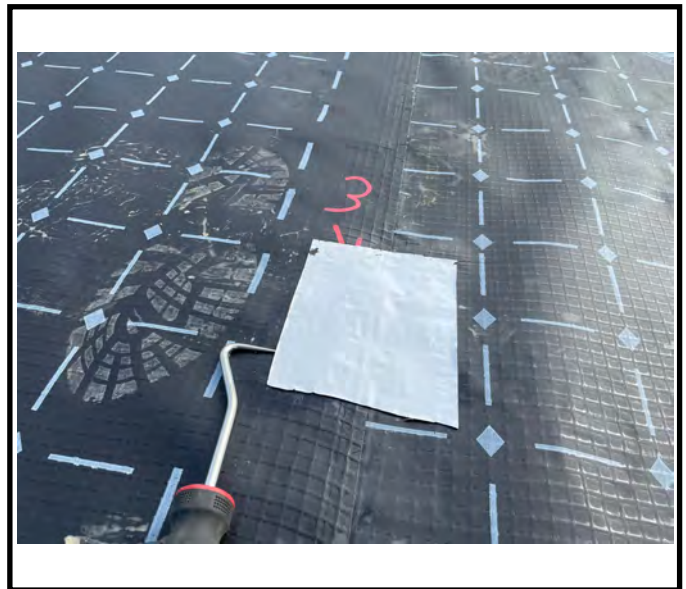
A mechanical point stress test being conducted upon the remediated fault.
