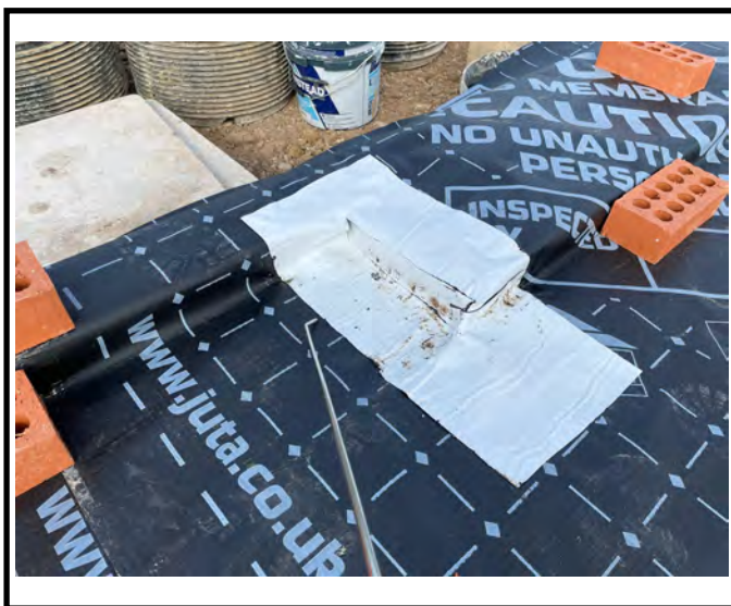
Air lance test on a sealed corner.
