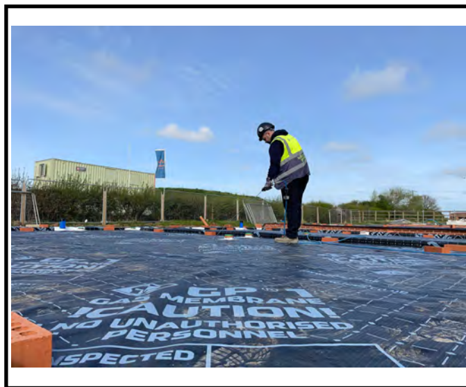
Air lance test on a welded lap.
