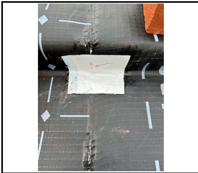
An overview of a patch repair of JUTA GP SAM.
