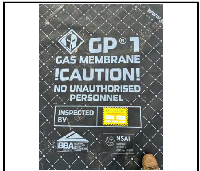
GeoShield verification pre sign off notice for Plots 46, 47, 48 & 49.
