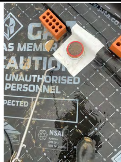
Air lance test on a pipe penetration.
