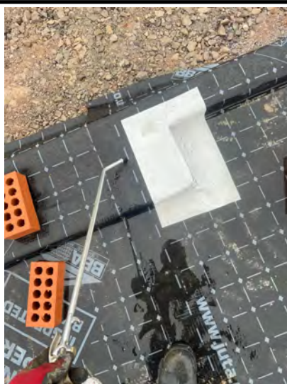
Air lance test on a sealed corner.
