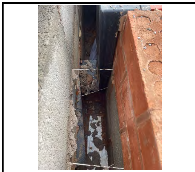
An overview down the cavity wall showing the telescopic vent connecting to the sub floor void.
