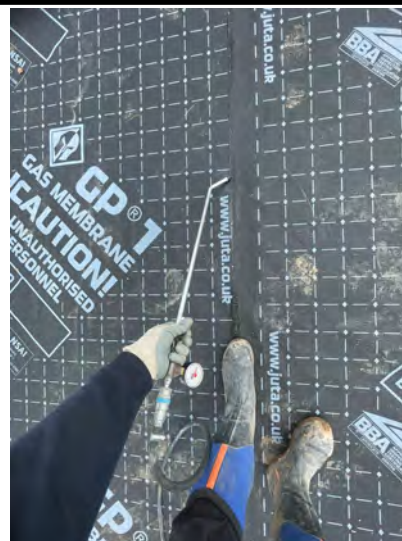
Air lance testing on a welded lap.
