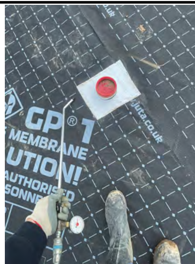
Air lance test on a pipe penetration.
