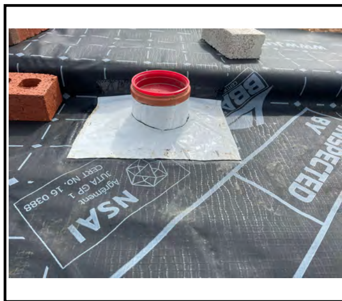
A sealed pipe penetration.
