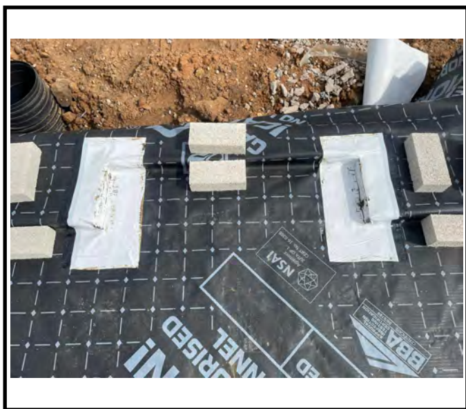
Sealed door threshold.
