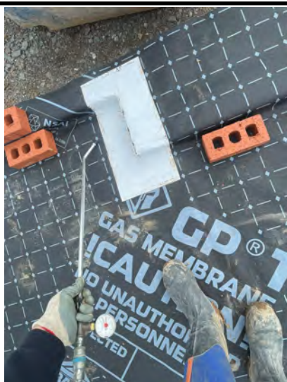
Air lance test on a sealed corner.
