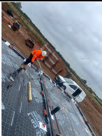
Air lance test on a welded lap.
