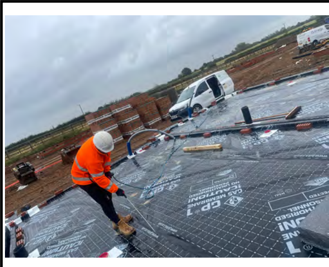
Air lance test on a welded lap.
