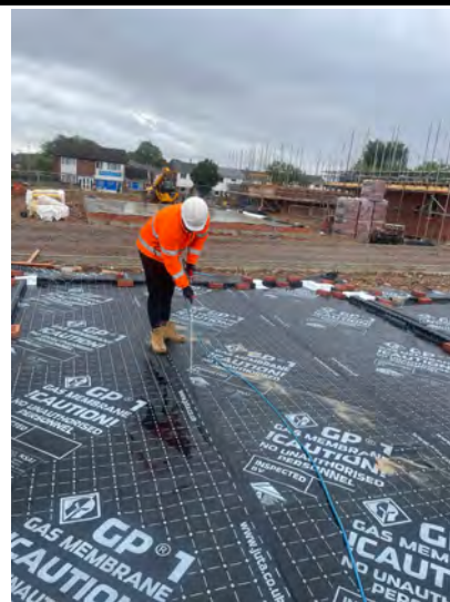
Air lance test on a welded lap.
