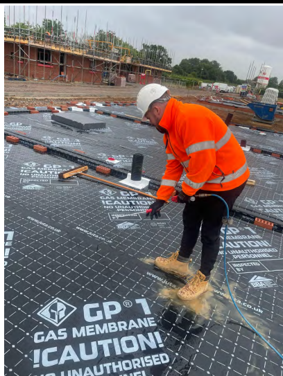
Air lance test on a welded lap.
