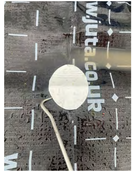
A mechanical point stress test being conducted upon a misweld remediated using a patch of JUTA GP SAM.
