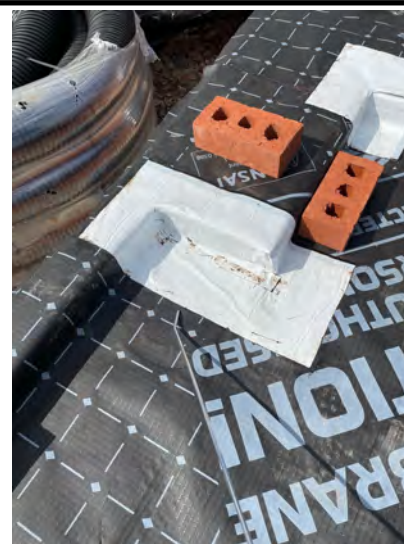
Air lance test on a sealed corner.
