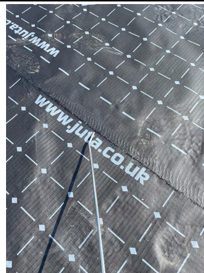
Air lance test on a welded lap.
