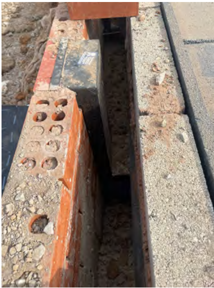
An overview of a vent brick.
