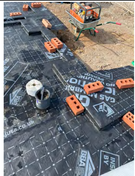
An overview of sealed corner detailing.
