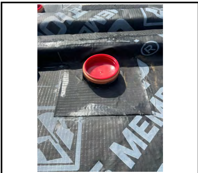
A sealed pipe penetration.
