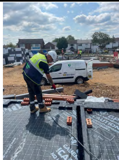
Air lance testing on a sealed corner.
