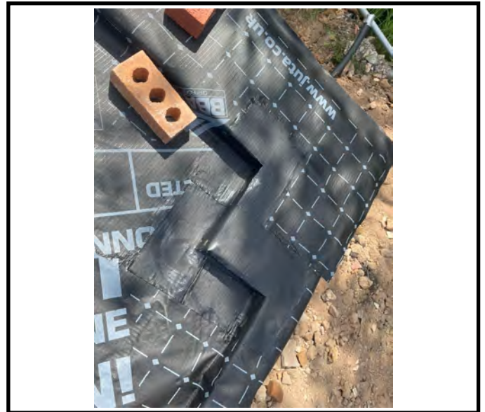
Sealed corner detailing.
