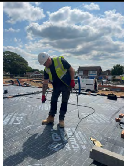
Air lance testing on a welded lap joint.
