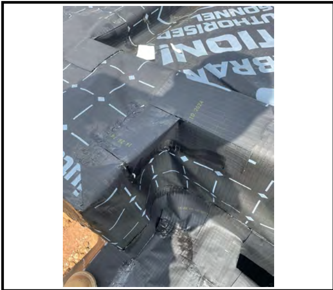
Sealed corner detailing.
