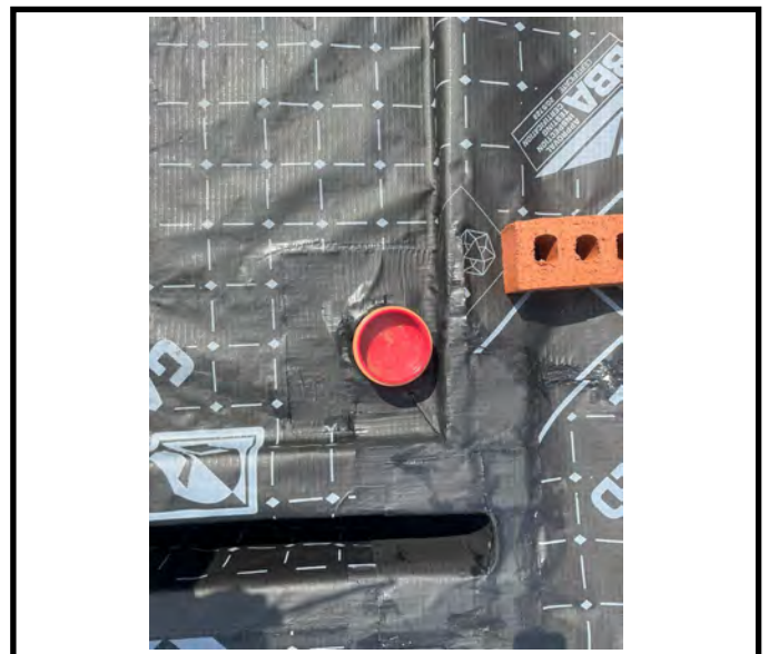
Sealed corner and sealed pipe penetration detailing.
