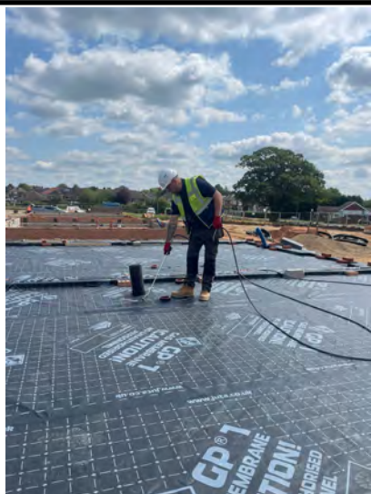
Air lance testing on a pipe penetration.
